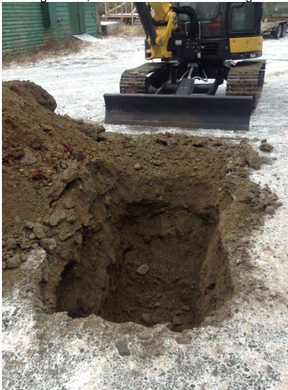
Photo 8 – View, test pit TP1, east of workshop.
