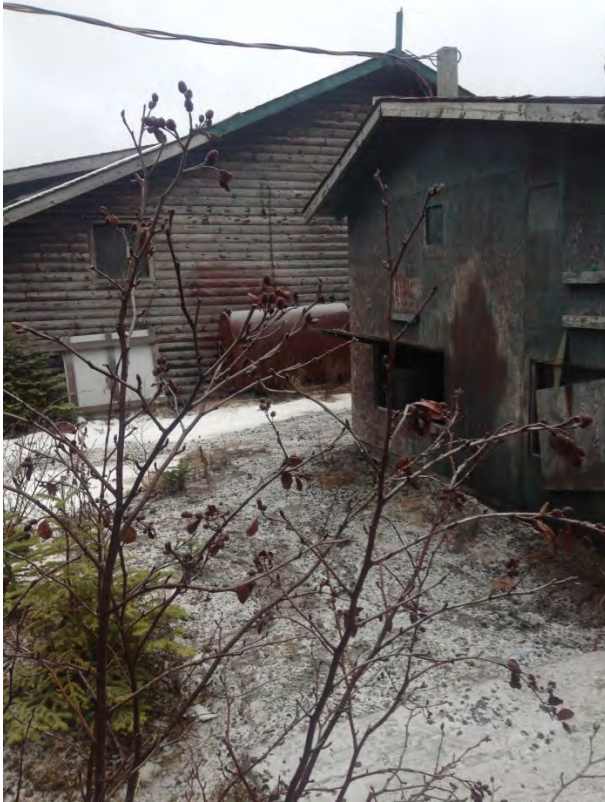
Photo 3 – View, looking northwest towards the generator shed and workshop.
