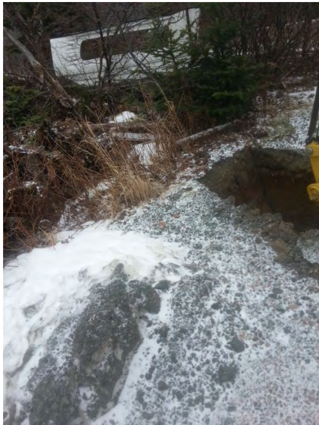
Photo 11 – View, test pit TP5, northeast of generator shed.
