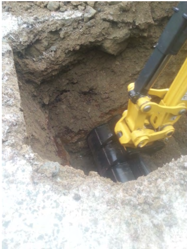
Photo 9 – View, test pit TP2, north of workshop.
