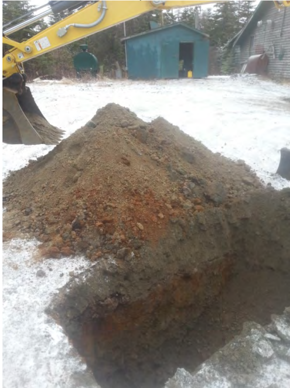
Photo 10 – View, test pit TP4, northeast of generator shed.
