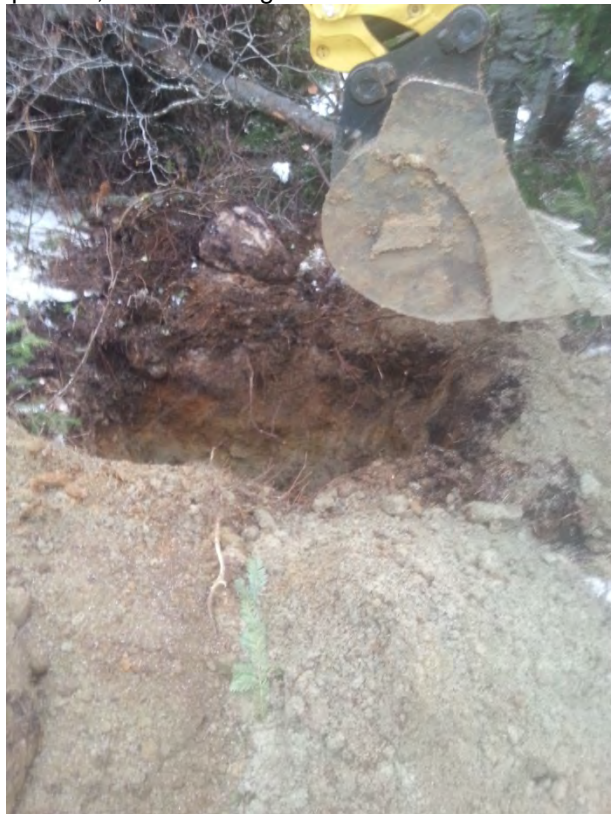
Photo 12 – View, test pit TP6, southwest of workshop.
