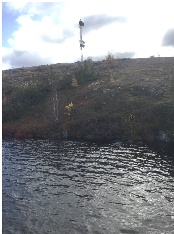
Photo 2 – Former U.S. Military Cartwright Site – General Area: Bell communication tower observed from pond located to the northwest of the Main Complex. Looking east.
