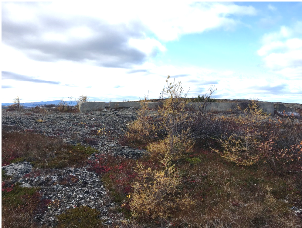
Photo 8 – Former USAF Dump Area and Ammunition Storage Area: foundation of former ammunition storage building. Looking west.
