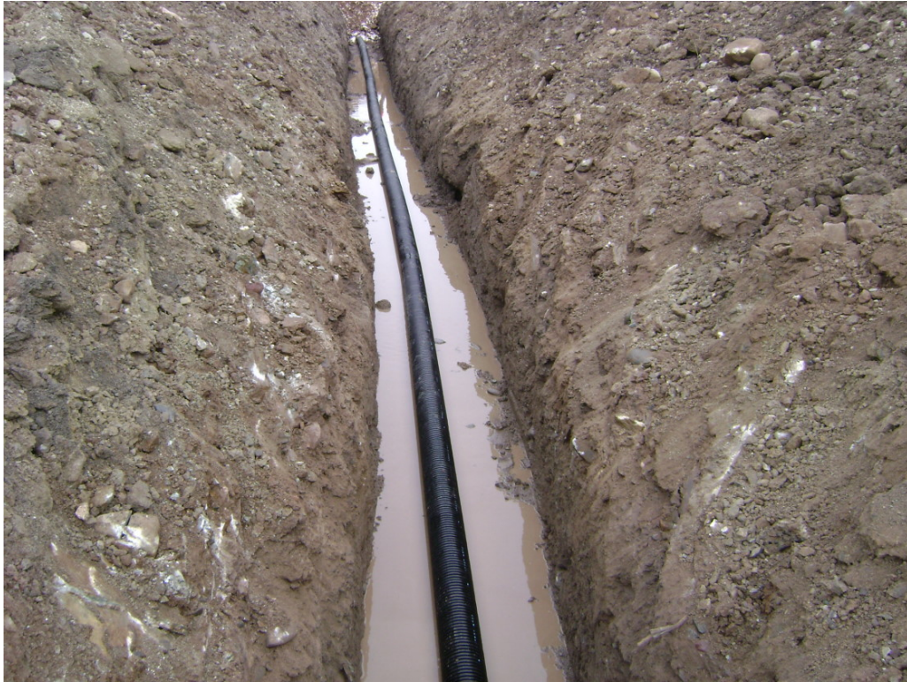
Photo 3: Trenching for Pipe Placement – Typical
