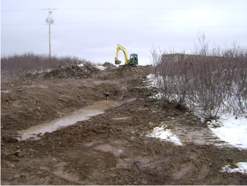
Photo 5: Groundwater Drainage System Outlet – Prior to Rip-Rap Placement
