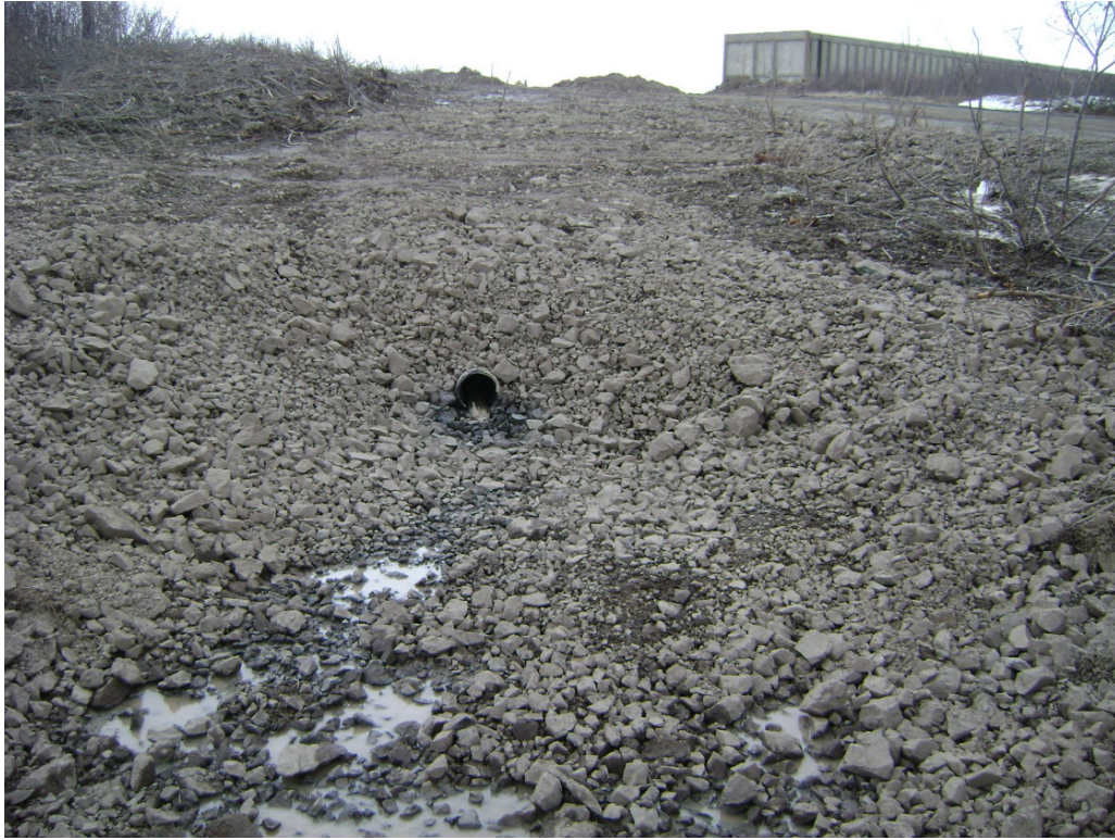
Photo 7: Groundwater Drainage System Outlet – After Rip-Rap Placement
