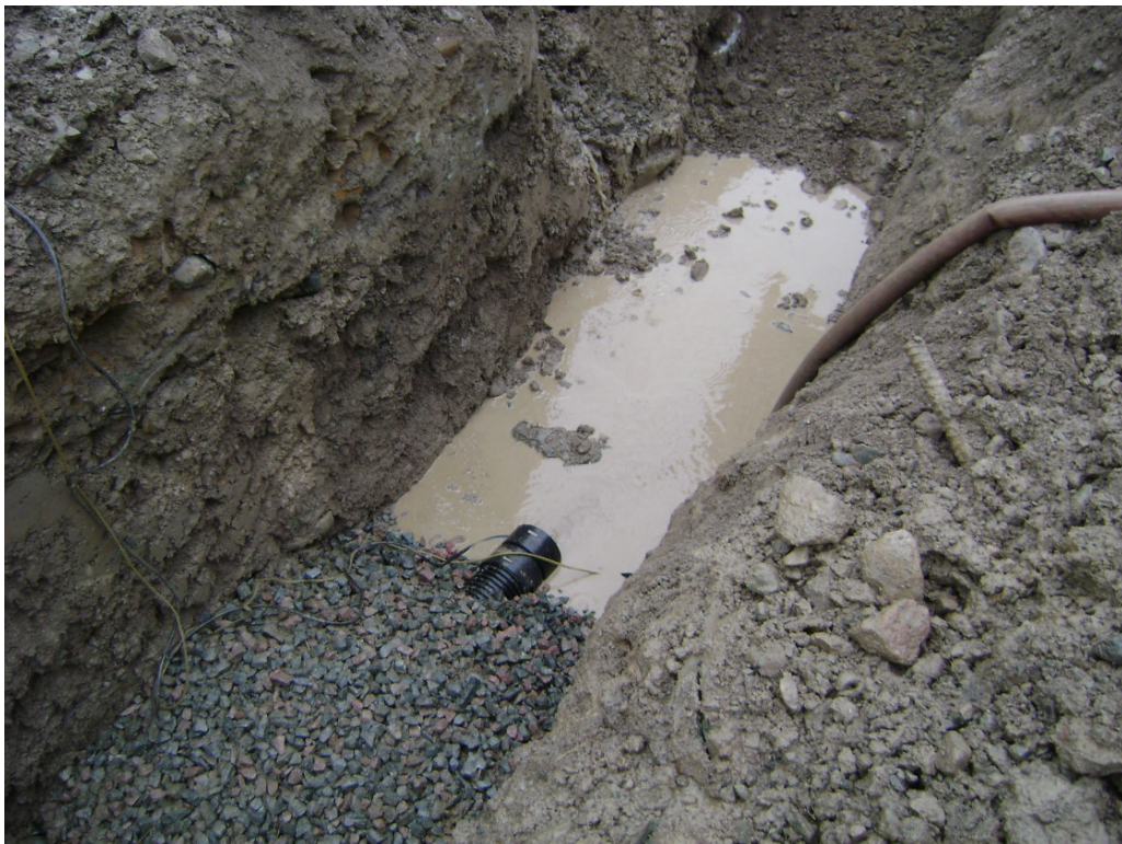
Photo 2: Washed Stone Placed on Perforated Pipe – Typical
