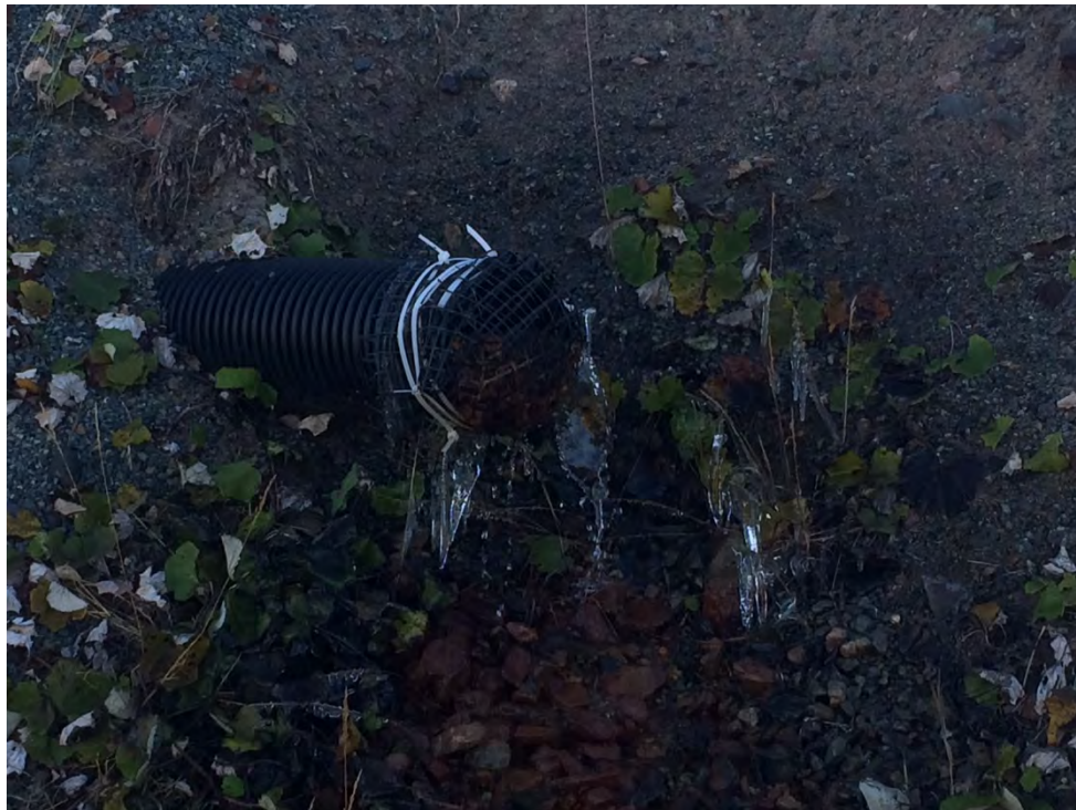
Photo 13 - View, looking east, showing the groundwater drainage system outflow with rodent screen attached.
