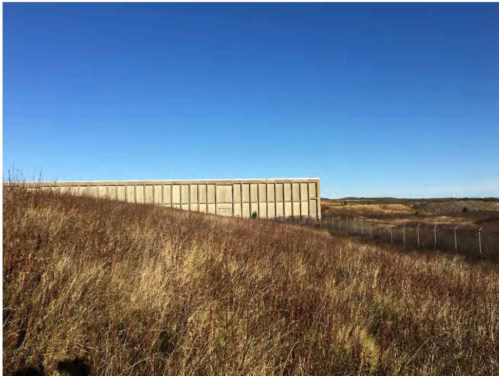
Photo 7 - View, looking north, from the top of the landfill during the inspection and survey of the cap in November 2017.
