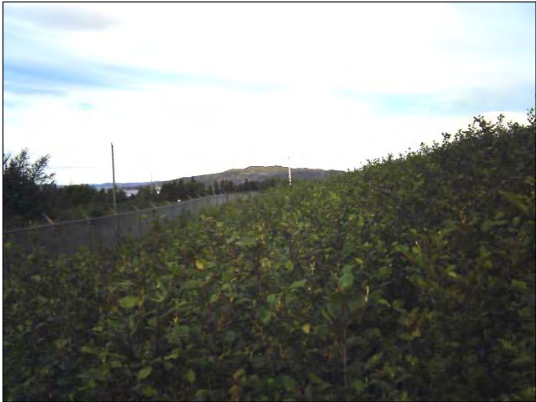
Photo 5: View, looking west, of the typical vegetative overgrowth along the southern slope of the landfill cover.
