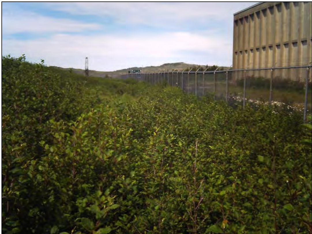
Photo 6: View, looking east, of the typical vegetative overgrowth along the northern slope of the landfill cover.
