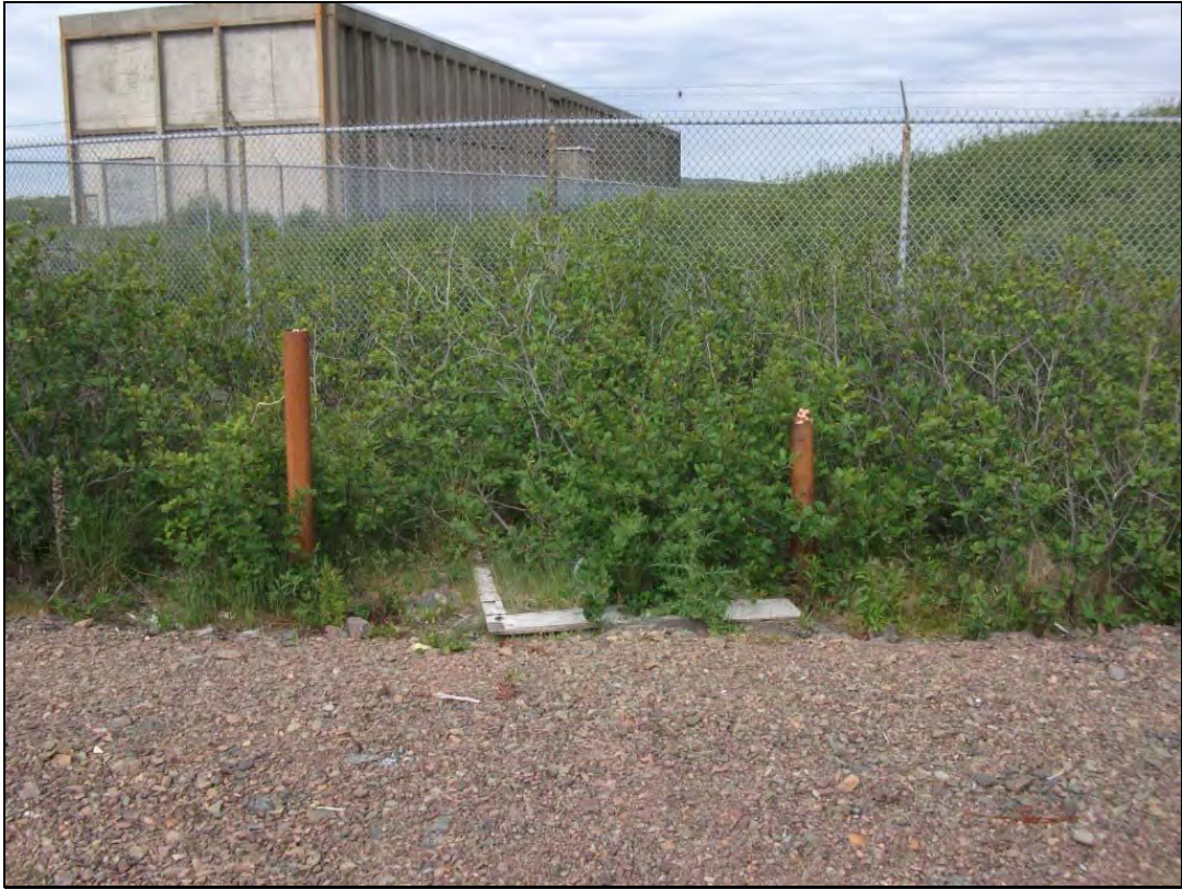
Photo 1: View, looking north, of the damaged stick-up monitor wells 93-3 and 93-3A.
