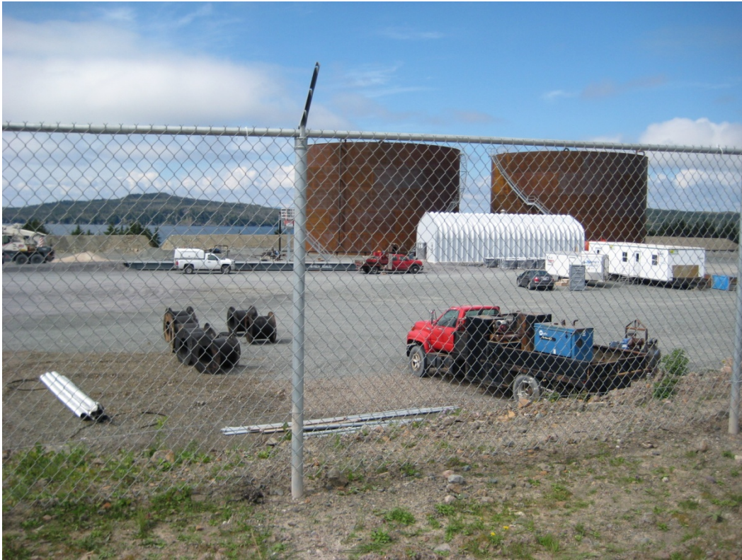
Photo 5: View of industrial development (liquid asphalt storage plant) located west of the landfill.
