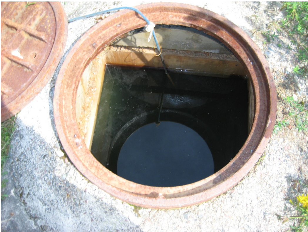
Photo 4: View of open PLCS chamber prior to sampling.
