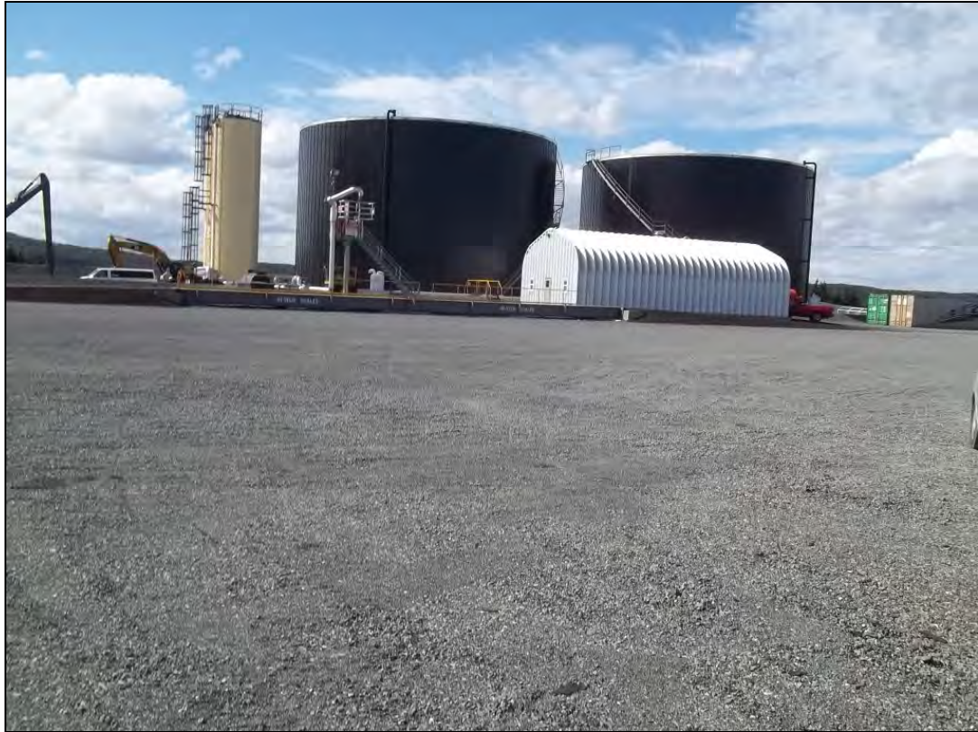
Photo 5: View, looking northwest, of the former SURFACE-DOWN location following construction of a new asphalt plant in 2011.
