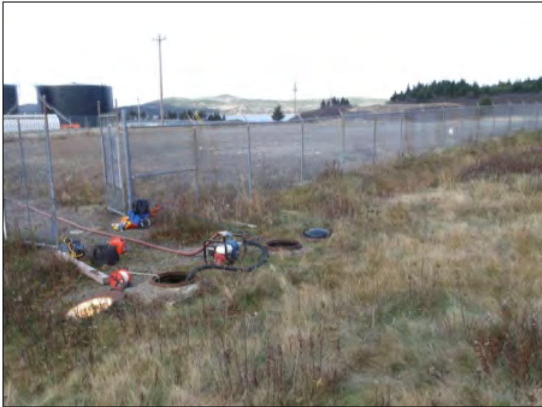
Photo 7: View, looking west, during the initial leachate pump and discharge event in November 2012.
