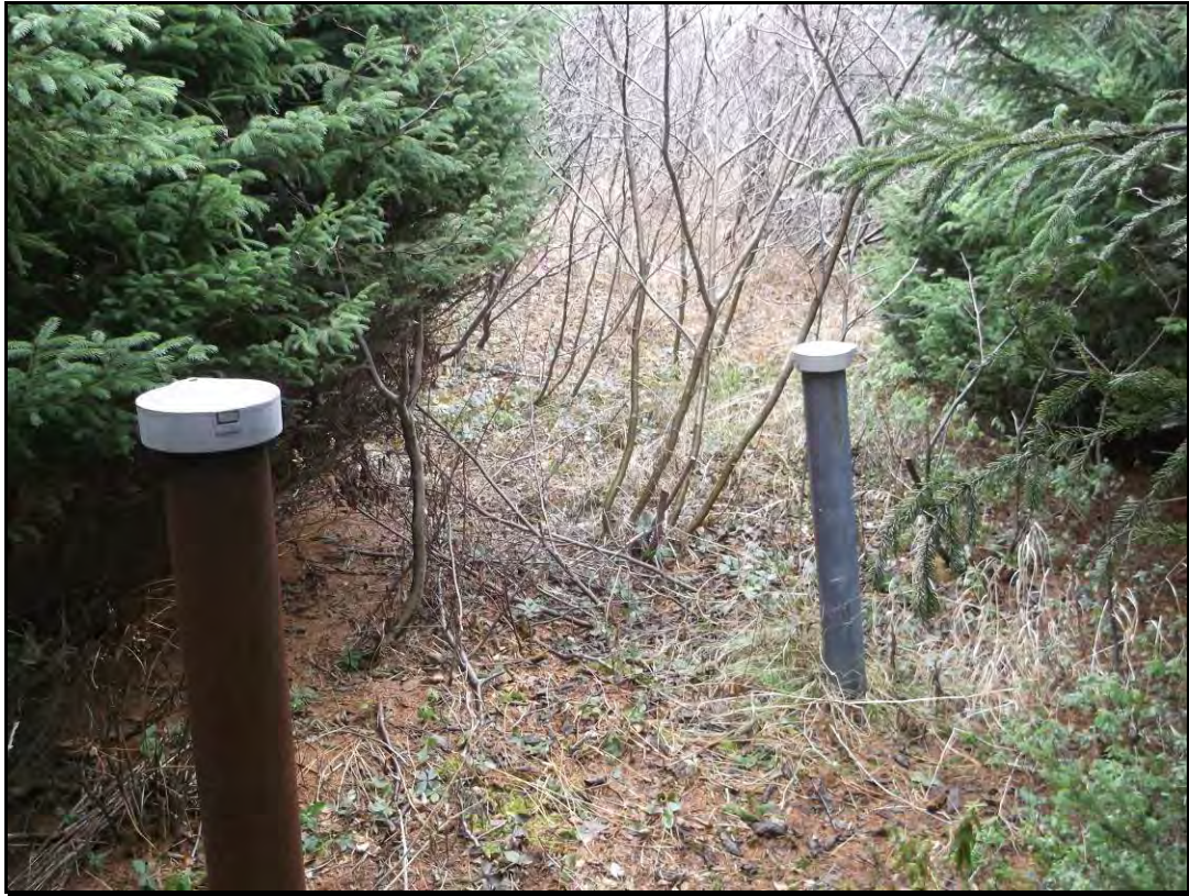
Photo 9: View, looking south, showing MW93-2 and MW93-2A during the November 2014 sampling event.
