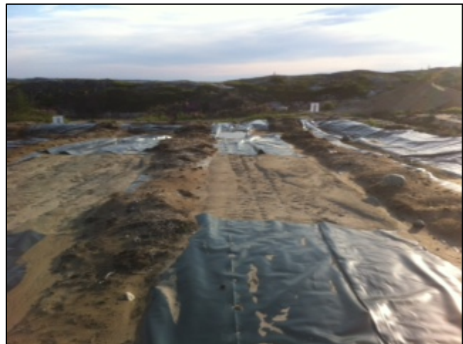
Photo 3 Damaged cover during August 2013 sampling.
