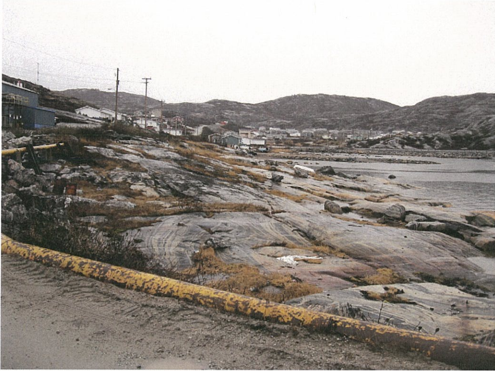
Photo 1 View of pipeline near the Wharf Area (looking northeast)
