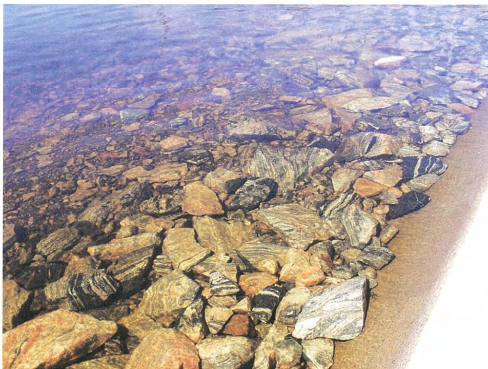
Photo 4 View of rip-rap and rubble protecting the dam at the Reservoir
