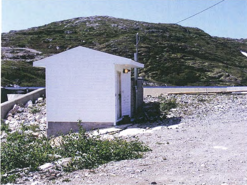
Photo 5 View of structure near the Reservoir (looking north)
