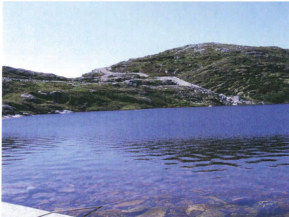
Photo 3 View of Reservoir (looking northeast)
