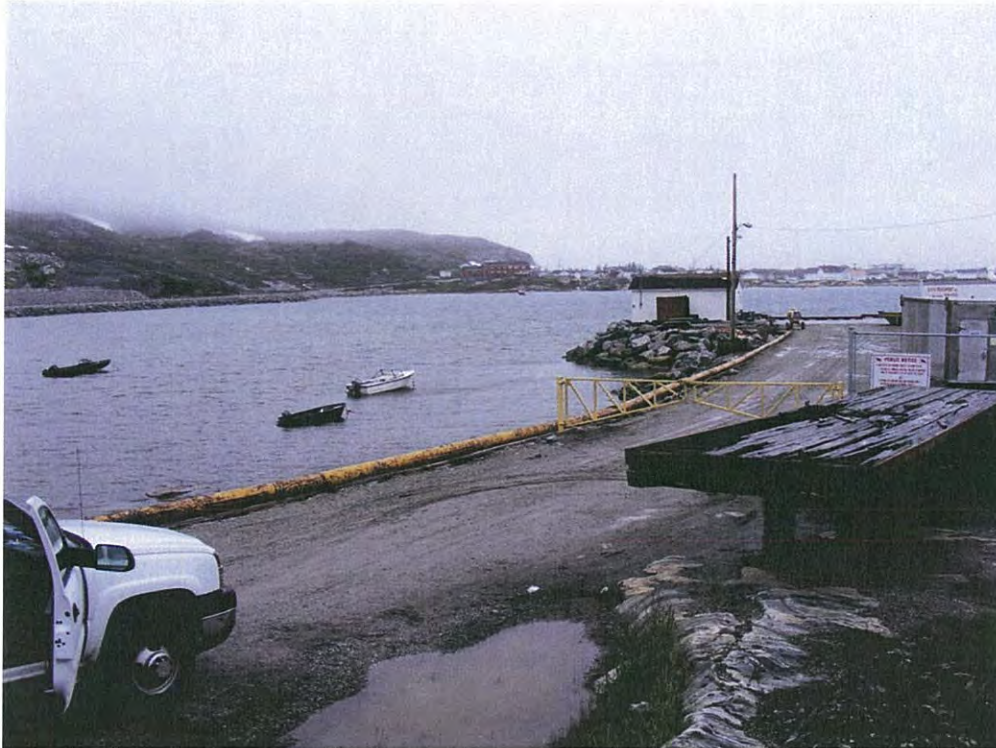
Photo 1 View of wharf, road, pipeline and Hopedale Harbour (looking southeast)
