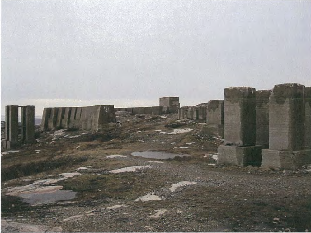
Photo 3 View of antennae bases at the BMEWS site (looking east)
