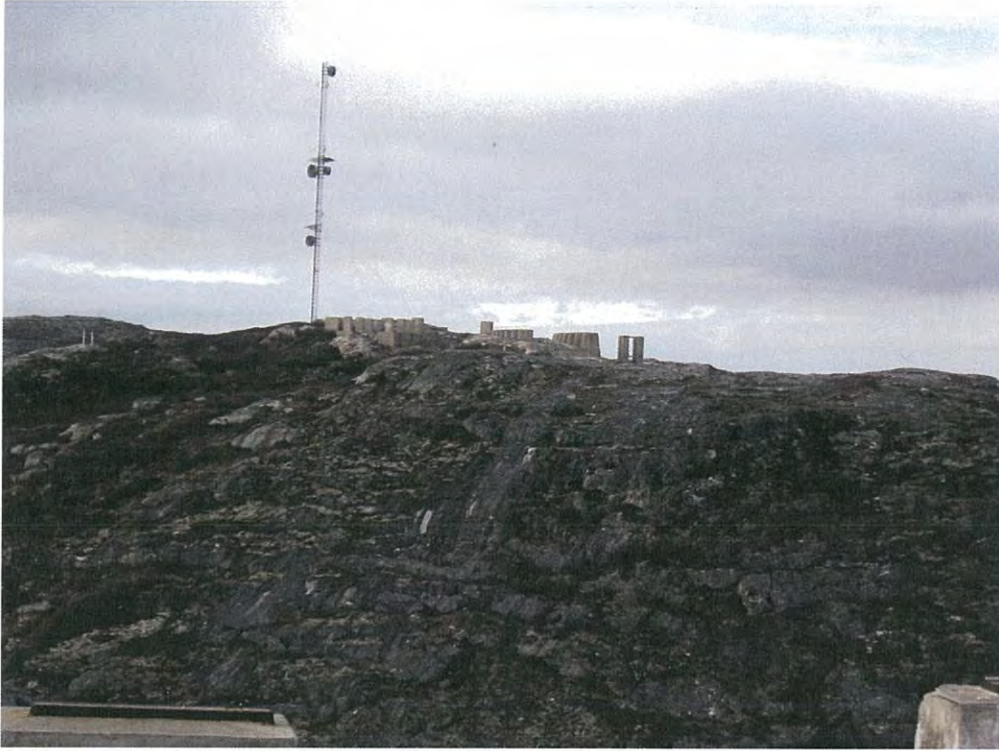
Photo 1 View of the BMEWS site (looking west from Old Base 1)
