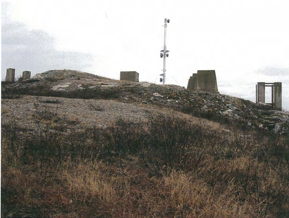
Photo 2 View of antennae bases at the BMEWS site (looking west)
