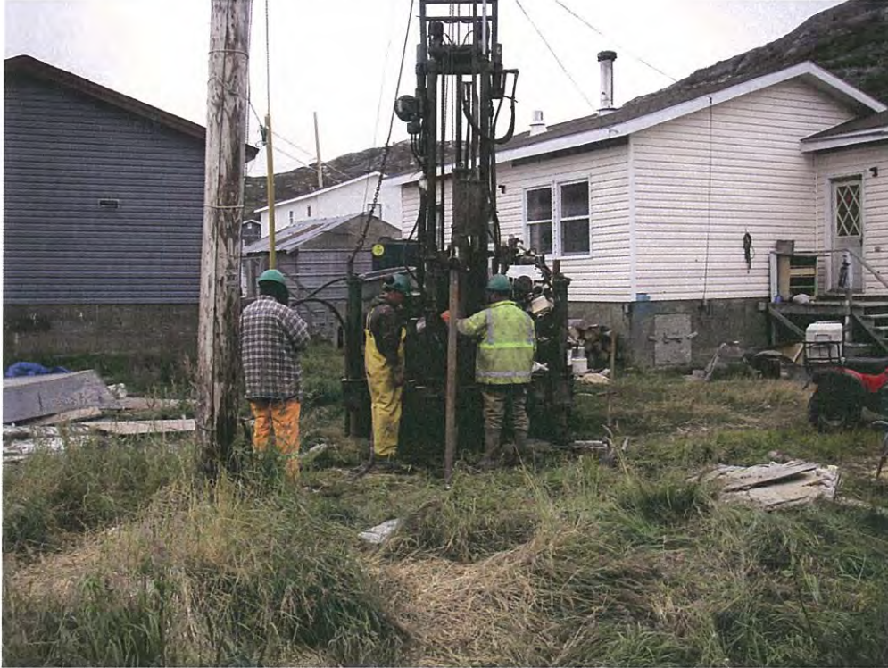
Photo 13 View of track mounted auger drill used to drill monitor wells
