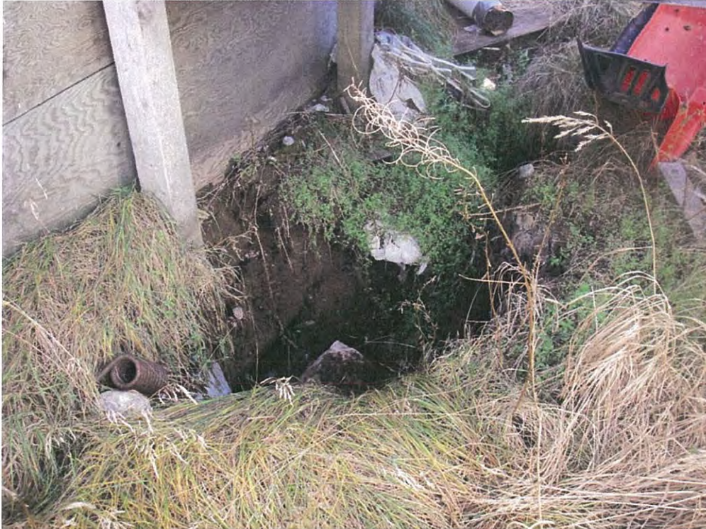
Photo 11 View of buried debris encountered in the Residential Subdivision
