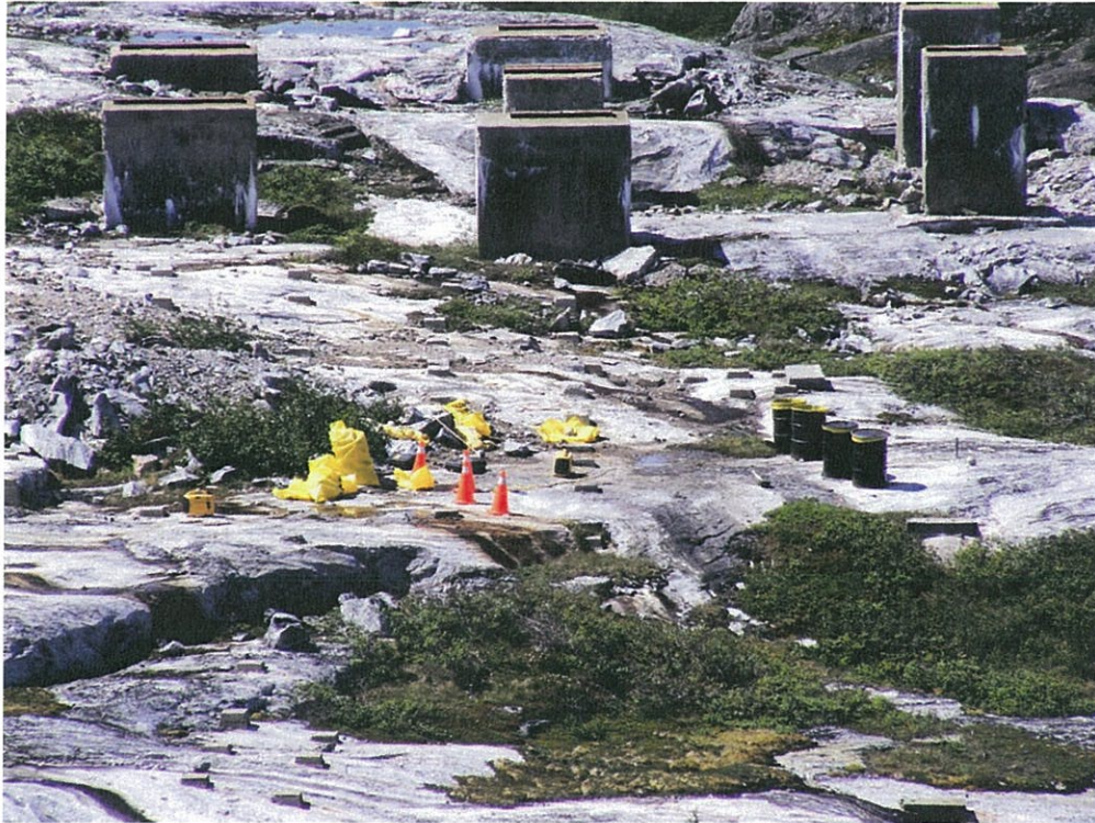
Photo 5 View of PCB-impacted tar remediation activities at Old Base 1 (looking southwest)
