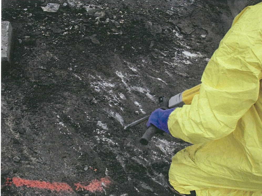
Photo 7 Chipping bedrock to remove PCB-impacted tar at Old Base 1
