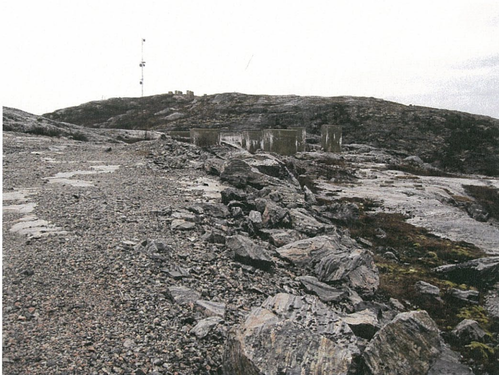
Photo 2 View of road and concrete foundations at the Old Base 1 site (looking west). The BMEWS site is apparent in the background.
