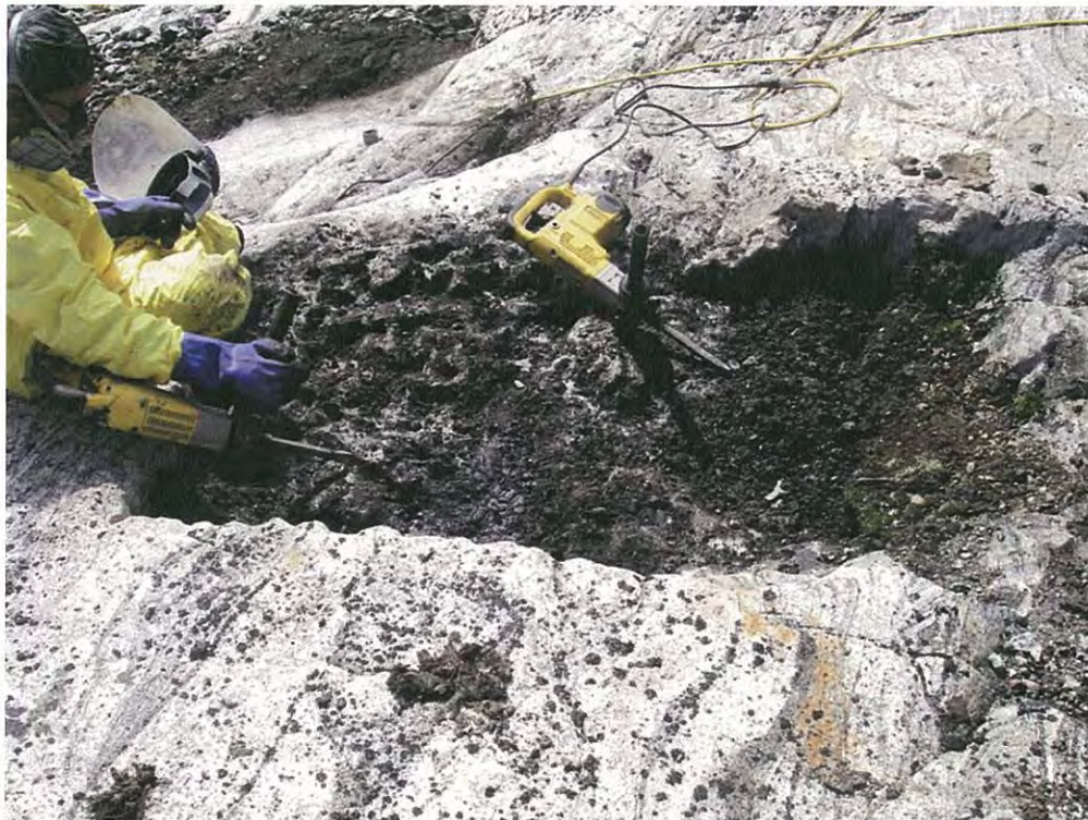
Photo 18 View of limited remediation of PCB-impacted tar at the Main Base site
