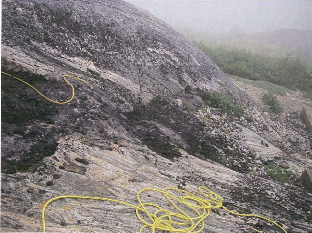
Photo 19 View of limited remediation of PCB-impacted tar at the Main Base site
