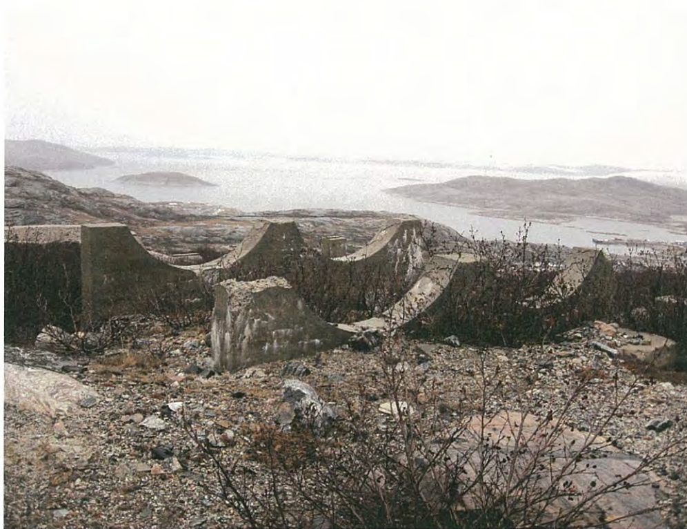
Photo 6 View of former tank location at Main Base
