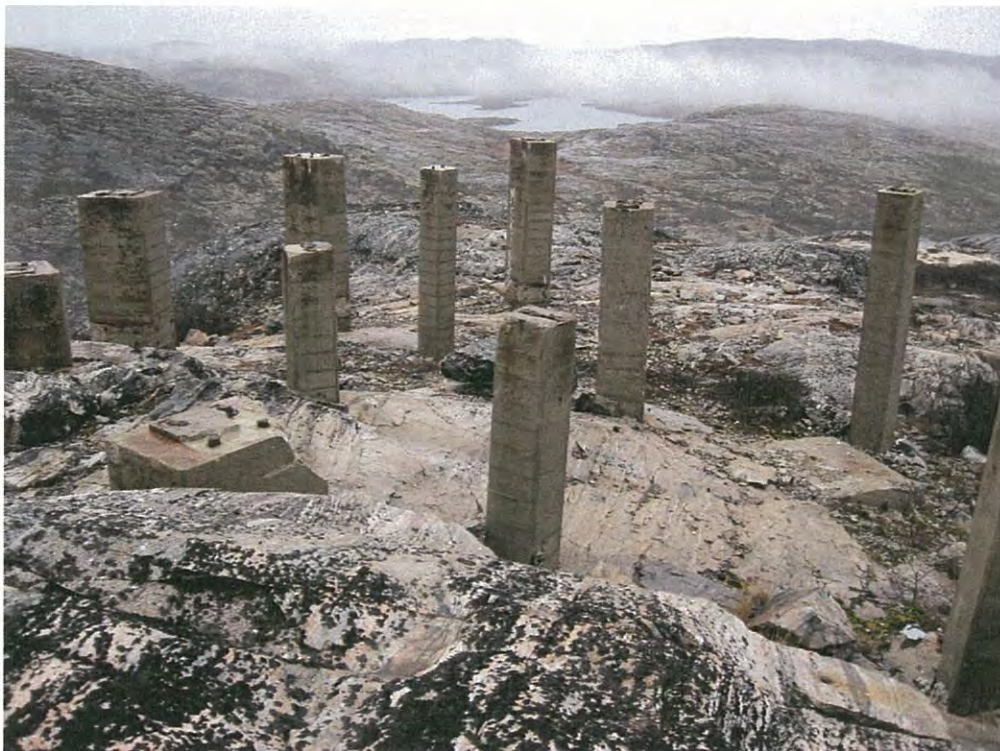
Photo 8 View of Main Base
