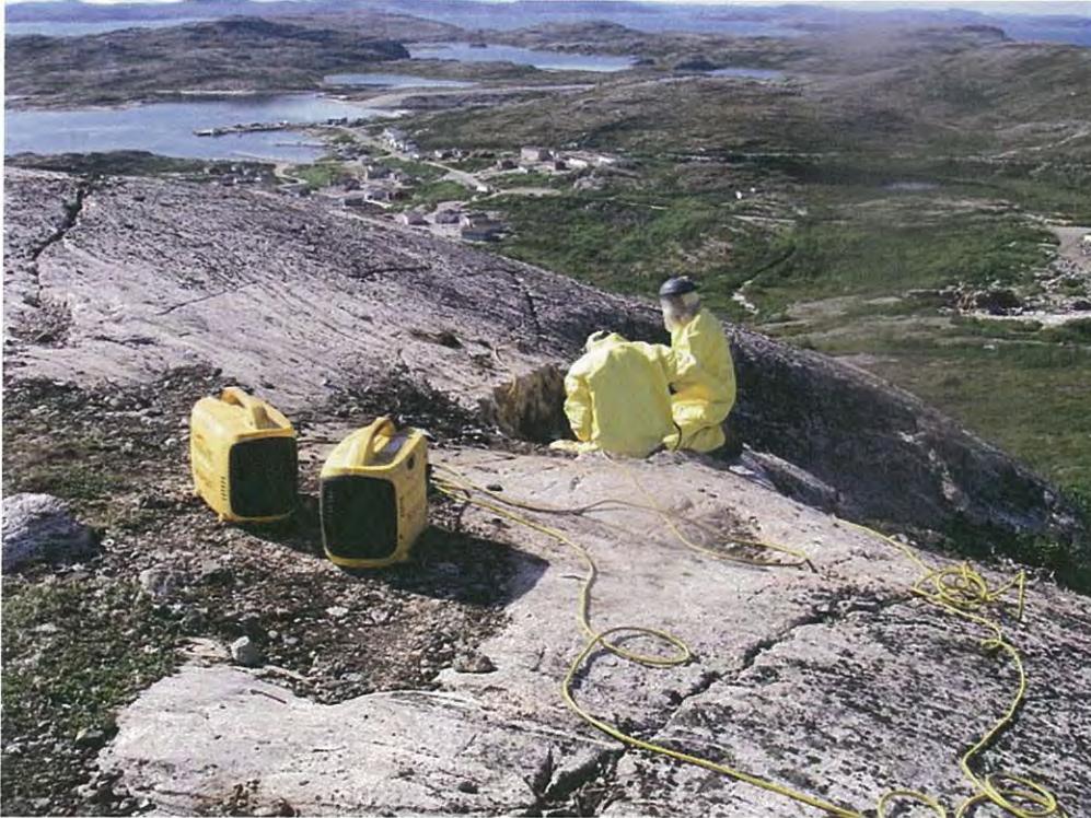
Photo 17 View of limited remediation of PCB-impacted tar at the Main Base site
