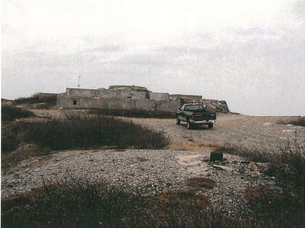
Photo 4 View of Main Base (looking west)
