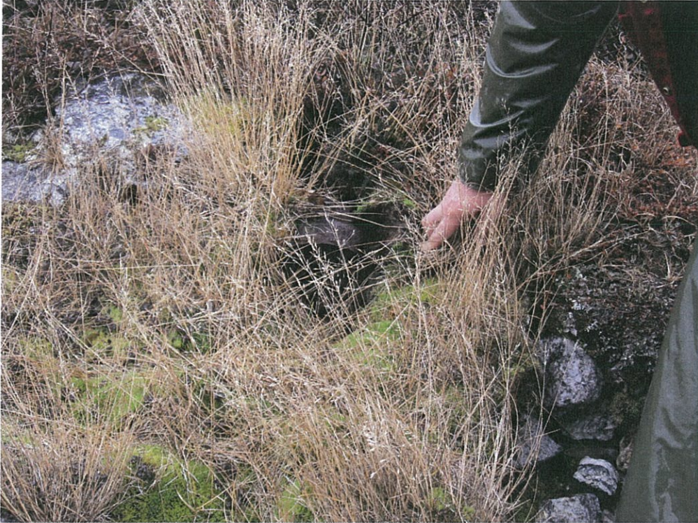
Photo 1 View of Sewage Outfall culvert
