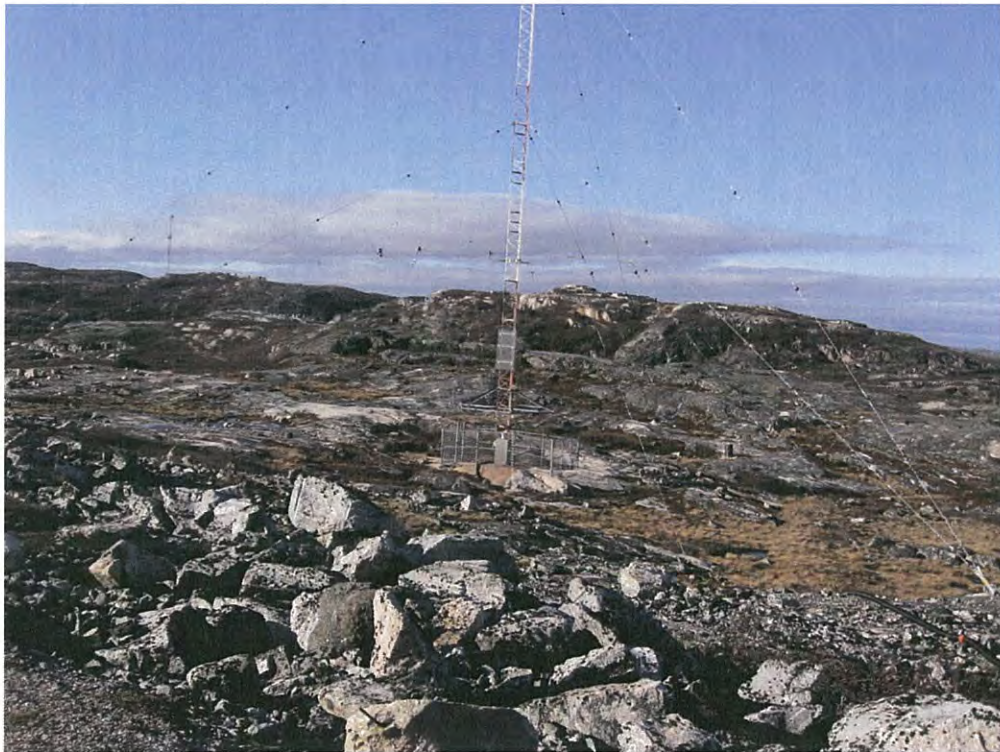
Photo 2 View of antenna at Mid-Canada Line site
