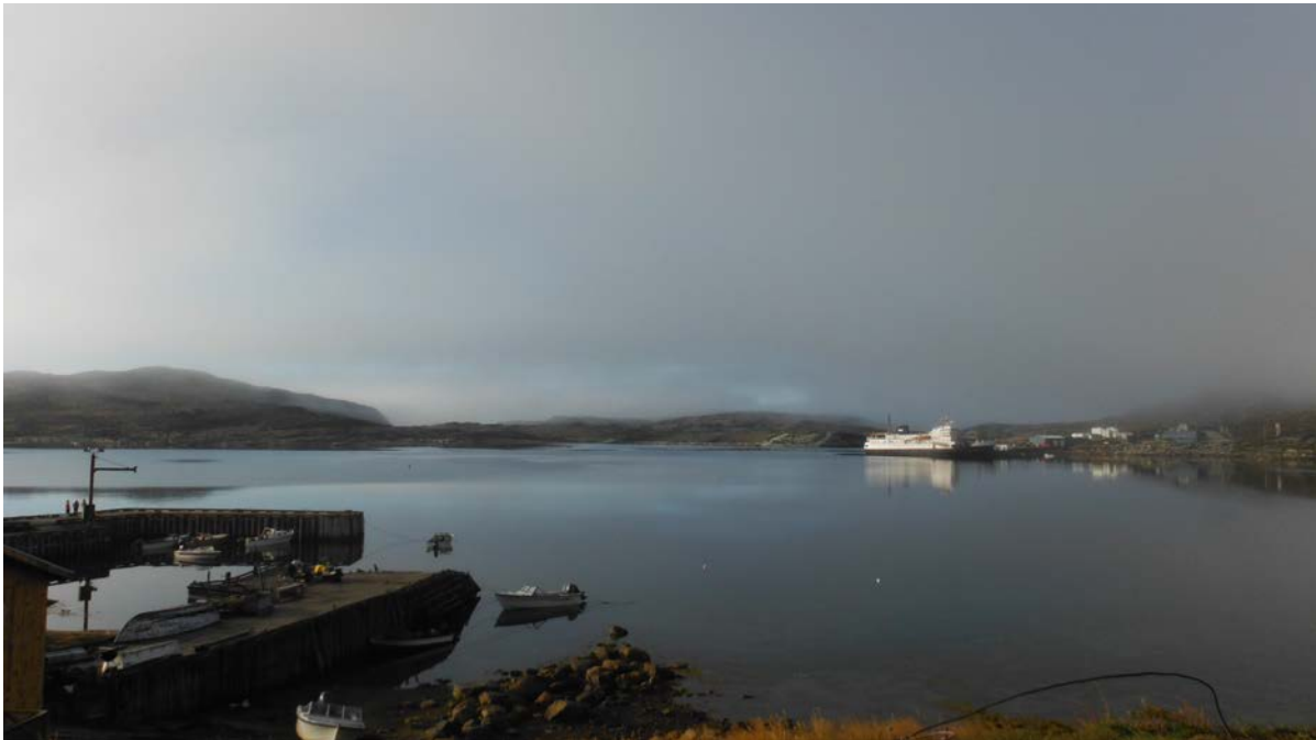
Photo 3 Wharf, looking southwest.
