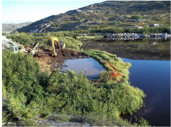
Photo 6 Remedial excavation adjacent to Old Dump Pond.
