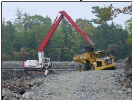
Photo 6 Sediment Removal by Excavator
