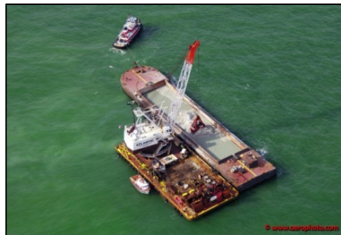
Photo 10 CableArm and barge.
