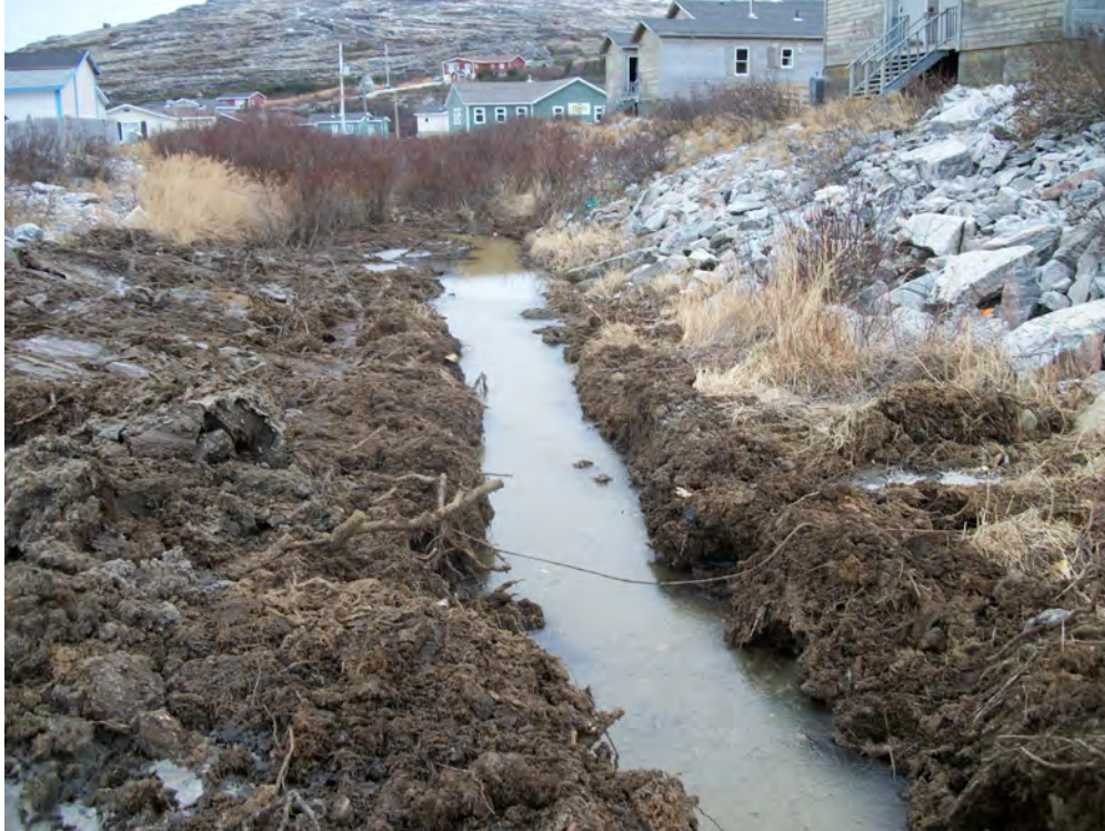
Photo 22 View of trenched stream on October 30, 2011.
