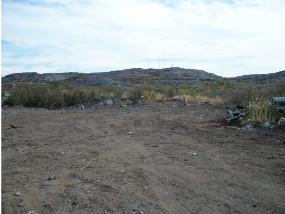
Photo 23 View of laydown area prior to installation of the liners.
