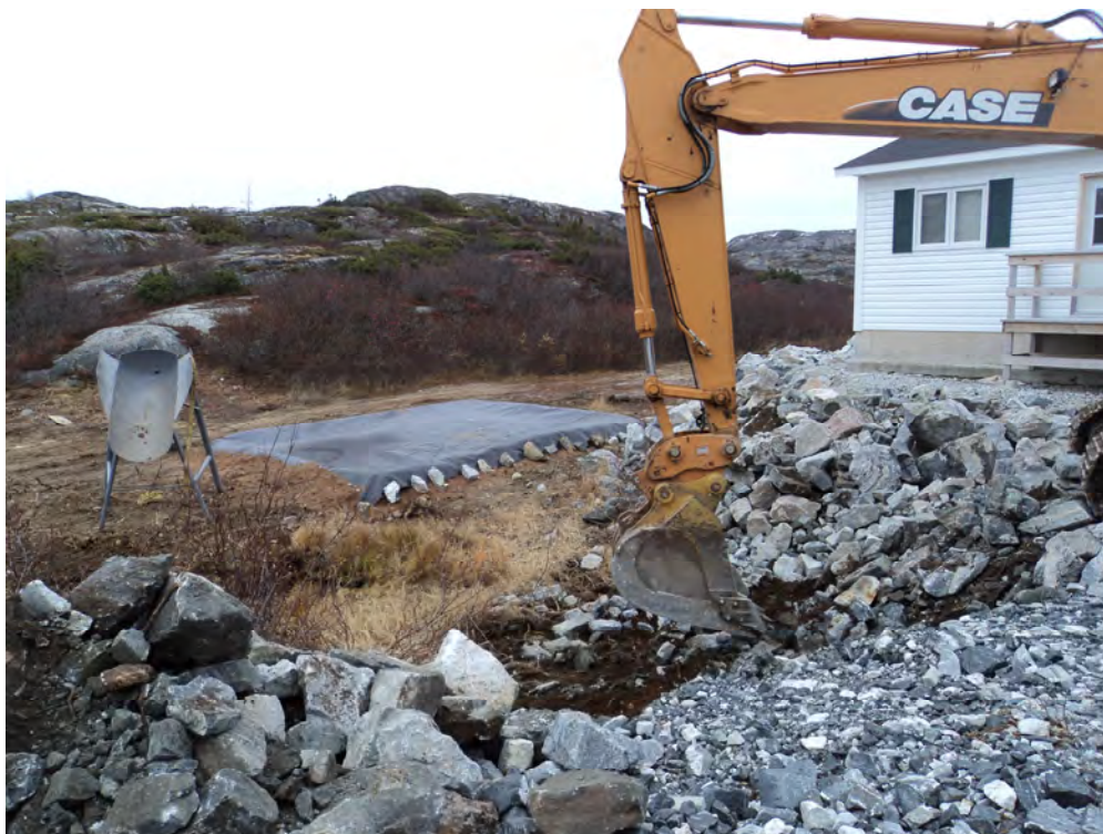
Photo 6 Removal of large rocks.
