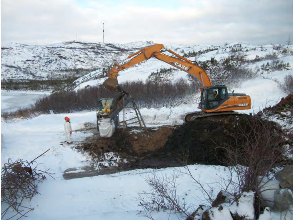
Photo 13 View of remedial excavation on November 5, 2011.
