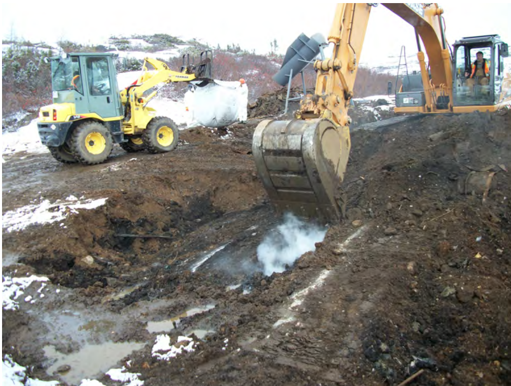
Photo 10 View of bedrock encountered at the base of the remedial excavation.
