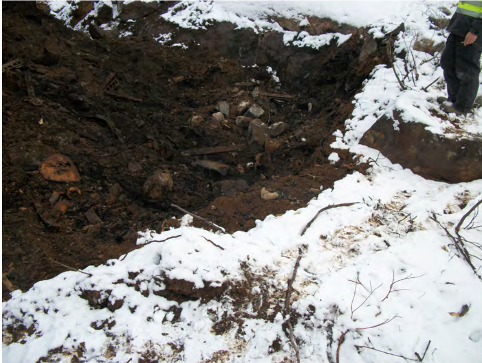
Photo 9 View of buried debris encountered in the remedial excavation.
