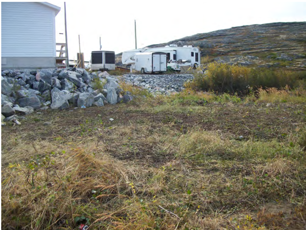
Photo 2 View of area requiring remediation surrounding MW-61 following site clearing and grubbing, looking south.
