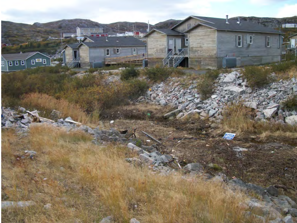
Photo 20 View of grubbed stream on October 4, 2011.
