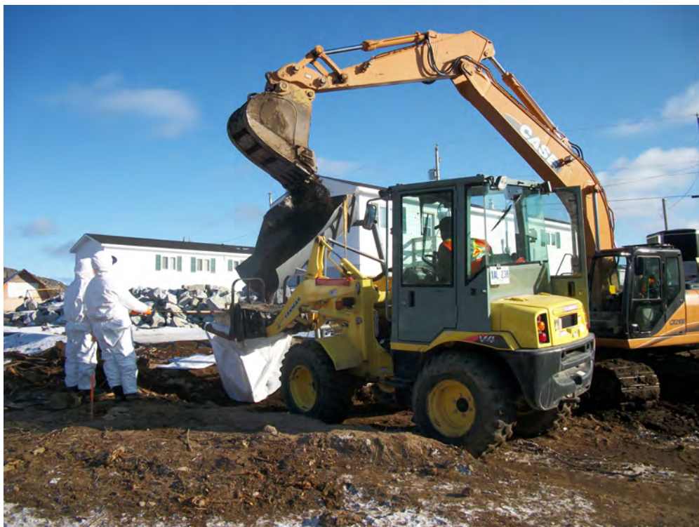
Photo 8 View of soil being loaded into bag on November 1, 2011.
