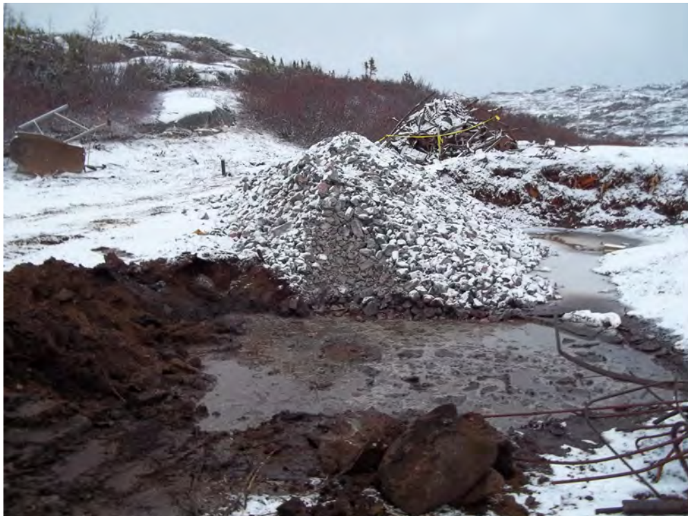
Photo 14 View of site during backfilling on November 16, 2011.
