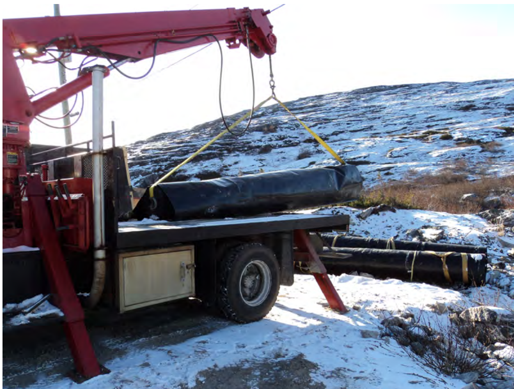
Photo 24 View of liner installation at the laydown area on November 1, 2011.
