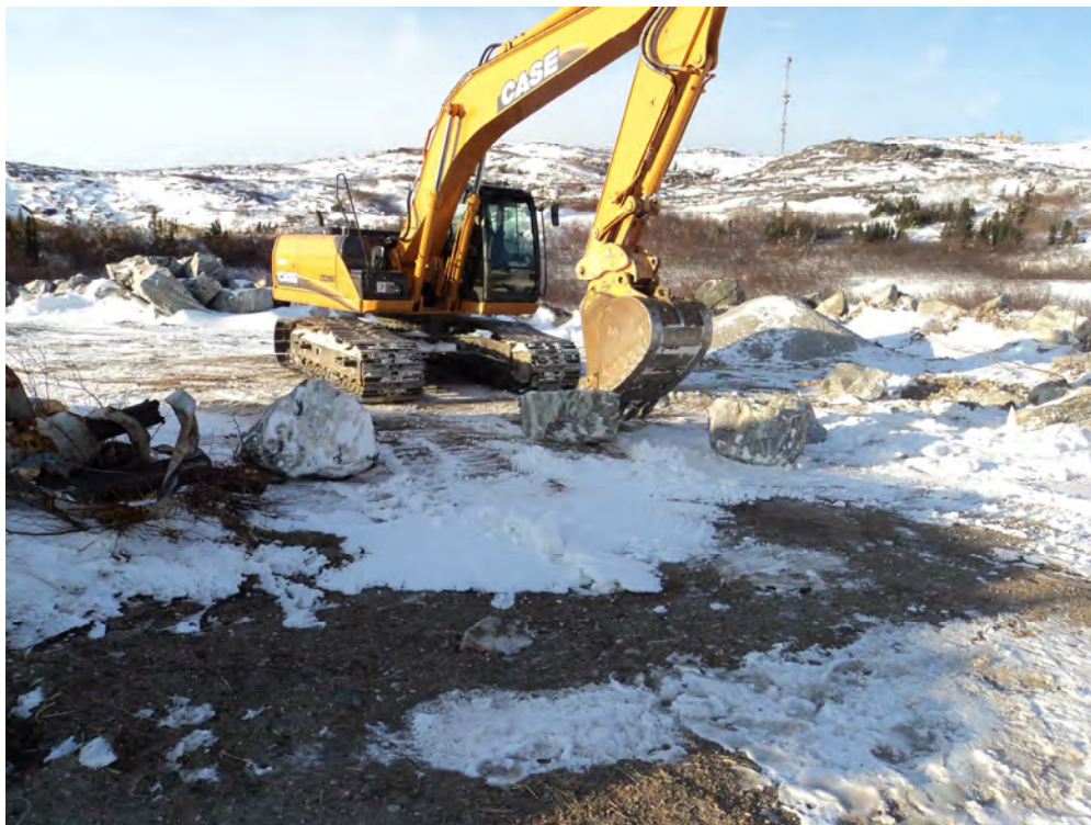
Photo 30 View of excavator blocking access to the laydown area on December 15, 2011.
