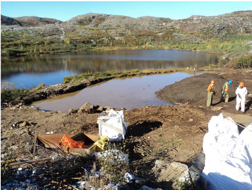
Photo 4 Final limits of ODP – Area 2 remedial excavation.
