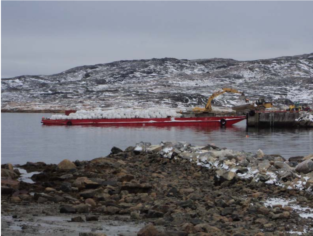
Photo 33 Loading soil bags onto the barge on November 9, 2012.
