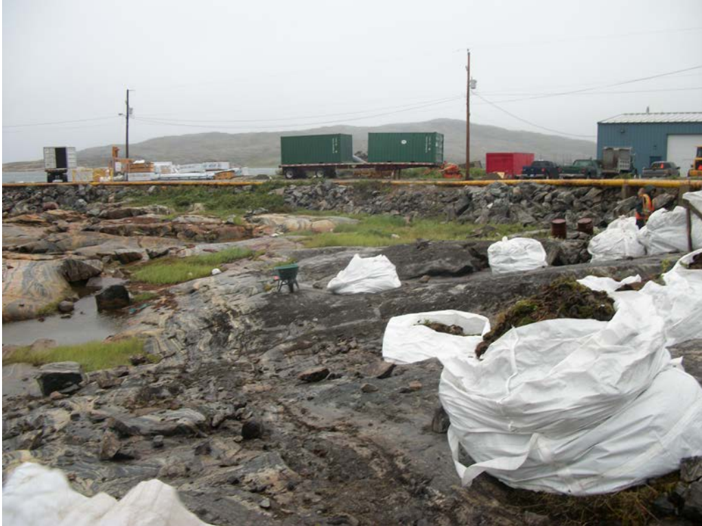
Photo 15 Beginning of soil removal at the Wharf site on July 19, 2012.
