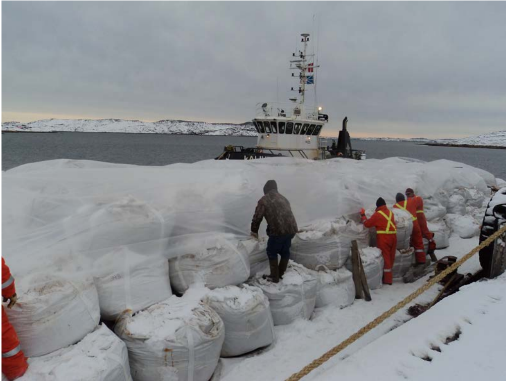
Photo 35 Installation of tarp over soil bags on barge.
