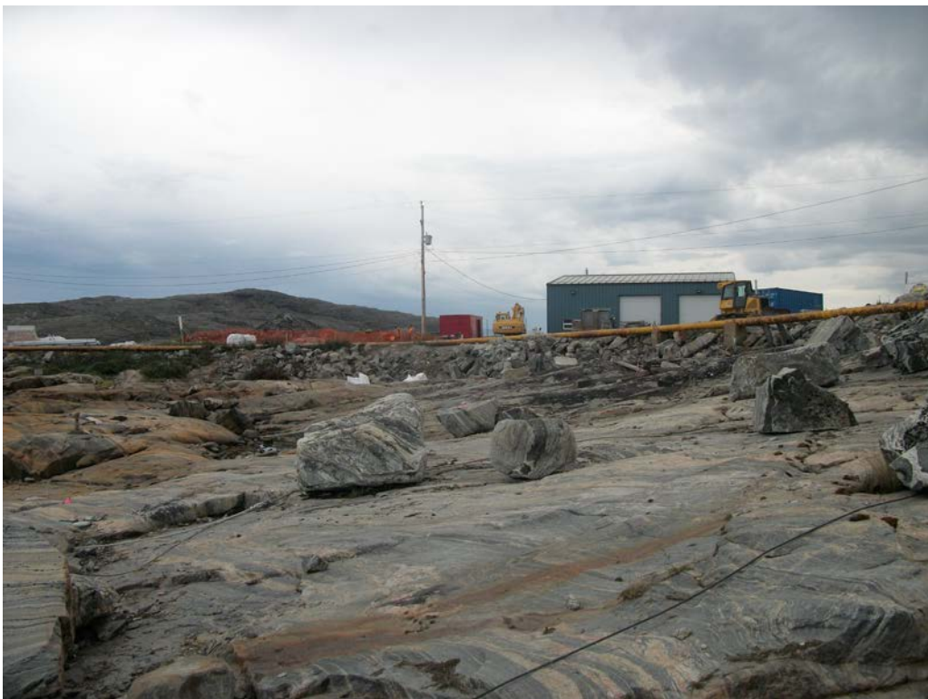
Photo 16 Wharf site between the shoreline and roadbed on August 21, 2012.
