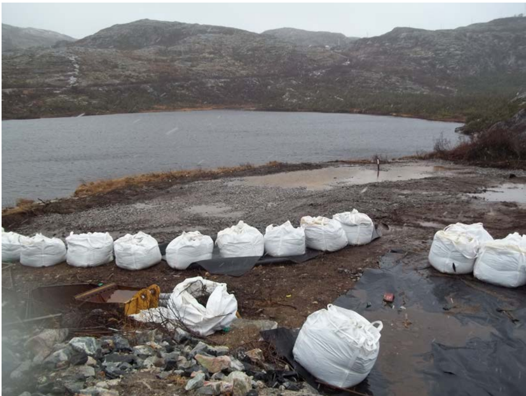
Photo 6 ODP – Area 2 following backfilling.
