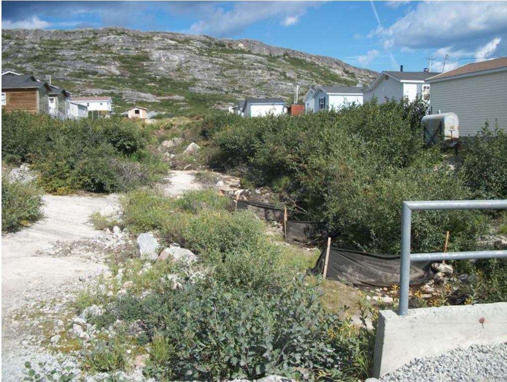
Photo 9 Silt fences installed downstream of the Stream site work area.
