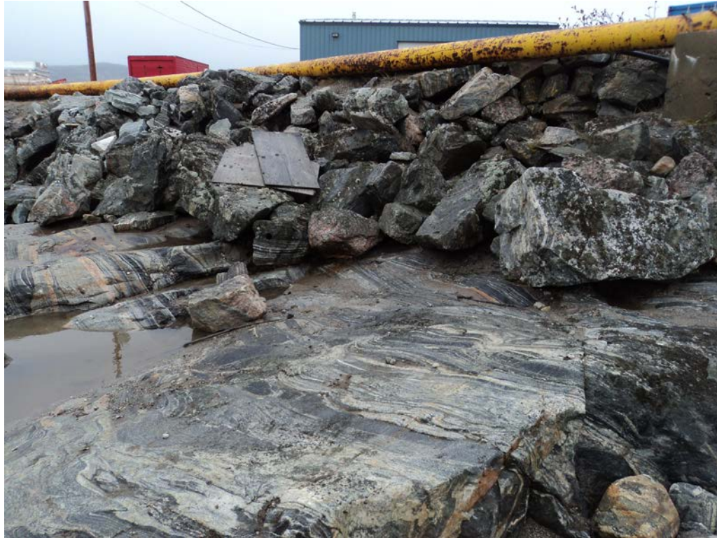
Photo 17 Edge of remedial area along the roadbed/pipeline.
