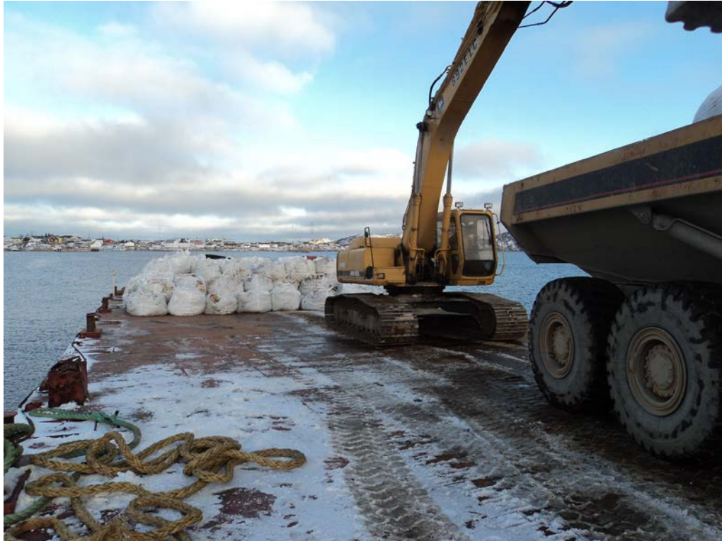
Photo 32 Loading soil bags onto the barge on November 8, 2012.
