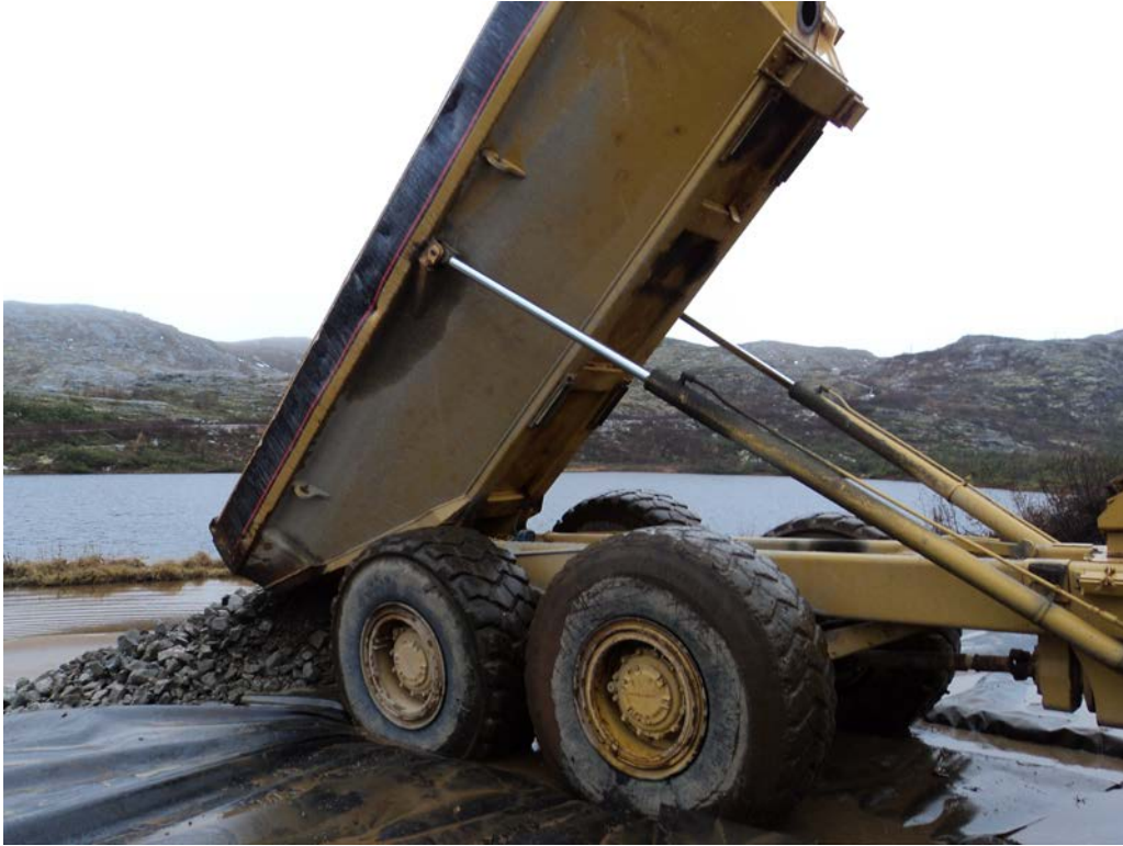
Photo 5 Backfilling at ODP – Area 2.
