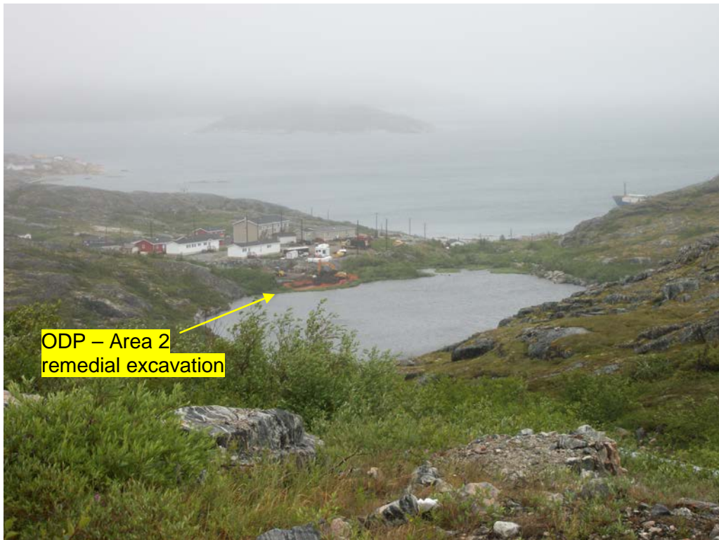
Photo 2 Remedial excavation overlooking Old Dump Pond.
