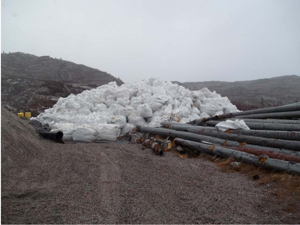
Photo 25 Laydown Area on November 9, prior to loading barge.
