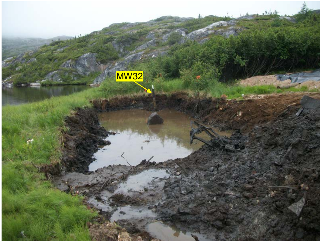
Photo 1 Soil removal at Old Dump Pond (ODP) – Area 2 on July 12, 2012.
