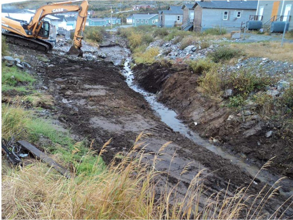
Photo 13 Stream site reinstatement, looking southwest.
