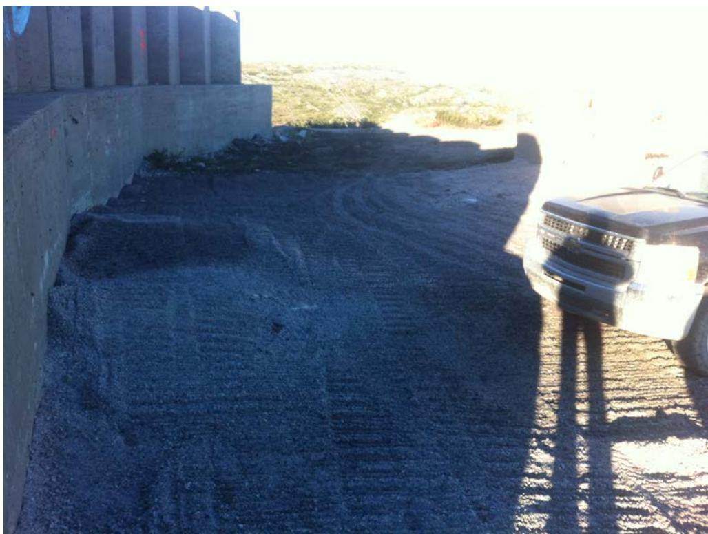
Photo 29 Surficial soil removed and area backfilled at the BMEWS laydown area.
