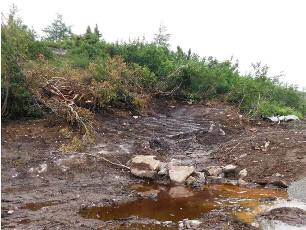
Photo 7 Remedial excavation terminated on bedrock in the vicinity of samples 13-ODP-BS16 and 13-ODP-BS17.
