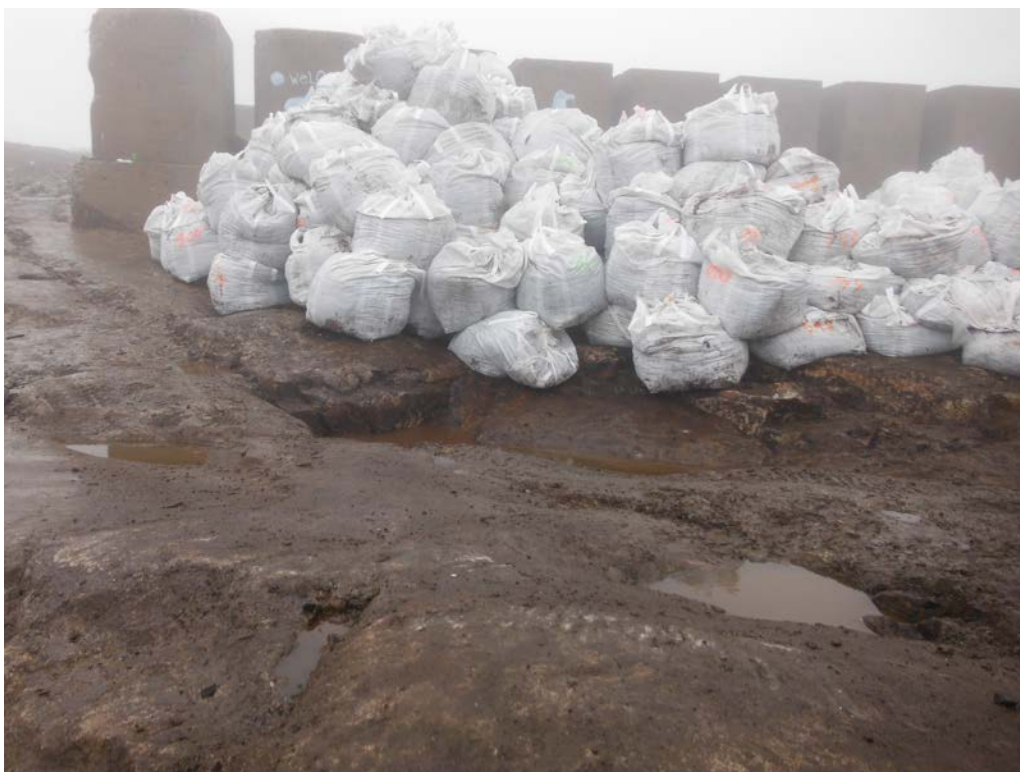
Photo 26 Soil bags temporarily stored on bedrock within the remedial excavation in the BMEWS area.
