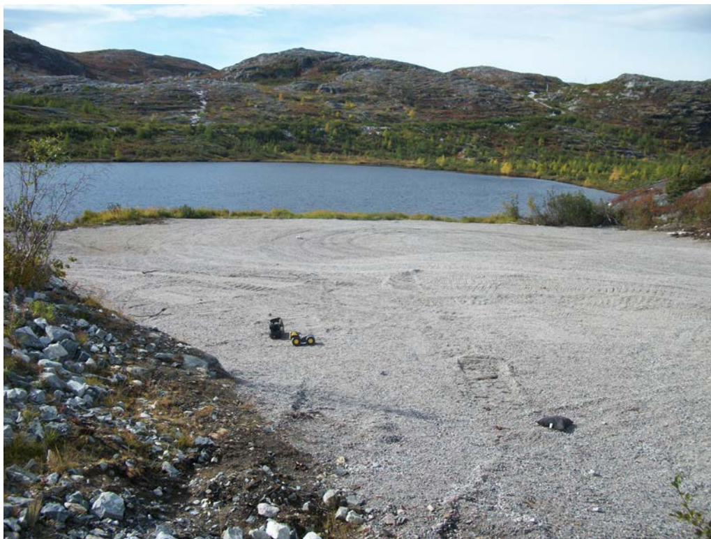
Photo 15 Old Dump Pond area backfilled.
