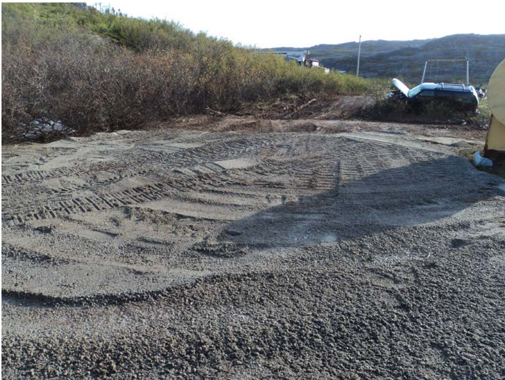
Photo 2 Laydown area prepared at Old Dump Pond.
