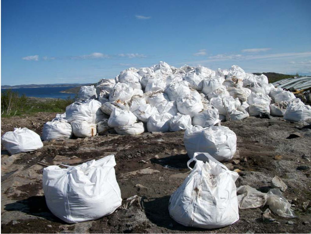
Photo 35 Main Laydown Area. Backfill material shown on bottom liner was subsequently removed and bagged.
