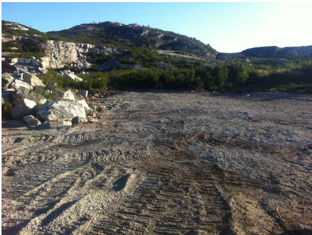
Photo 47 Main Laydown Area on September 2, 2013 following bag removal, surficial soil removal and backfilling.
