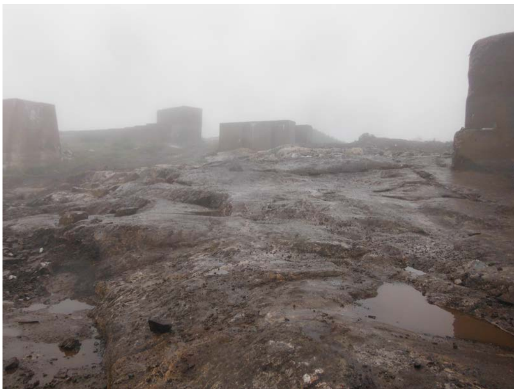
Photo 27 Central portion of BMEWS remedial excavation on August 6, 2013 (removed to bedrock).
