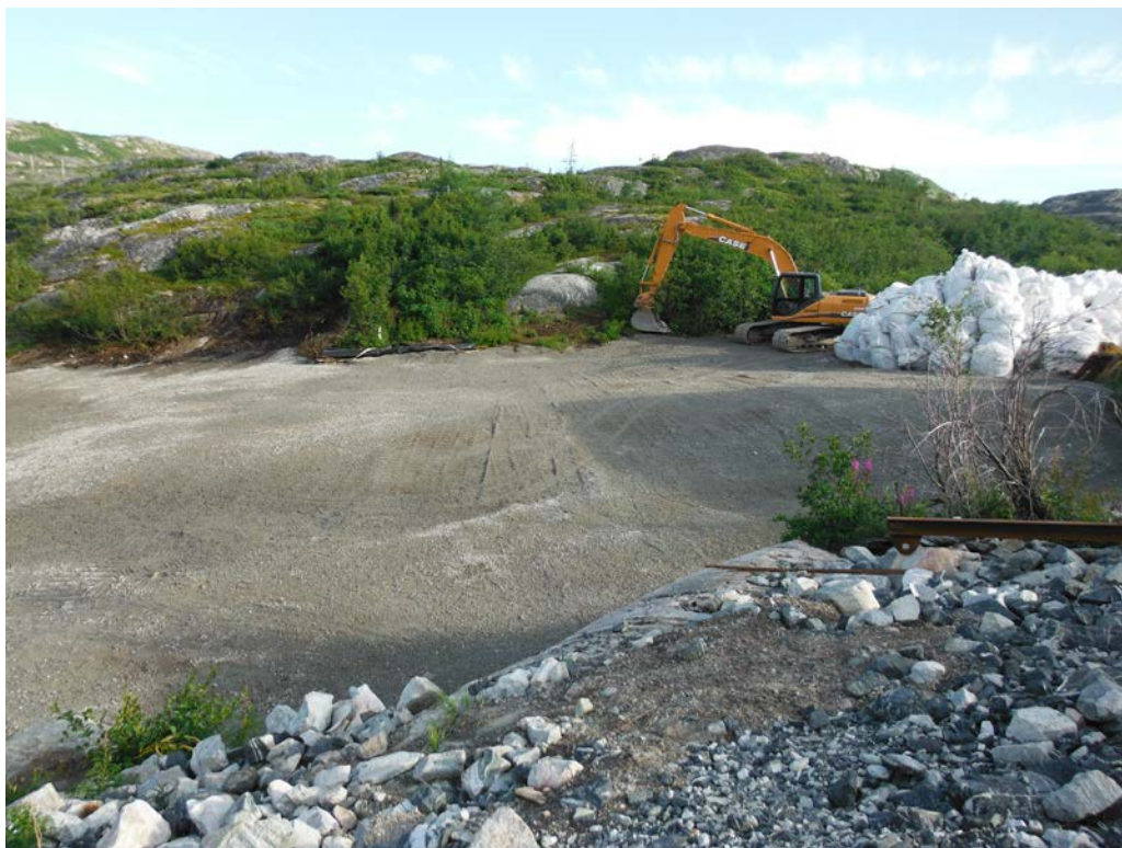
Photo 12 Surficial soil removed and area backfilled in Old Dump Pond area.
