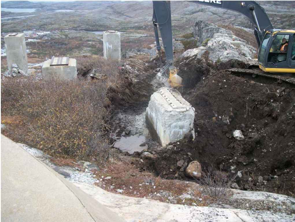
Photo 29 PCB-impacted soil removal at Main Base-Area 1.
