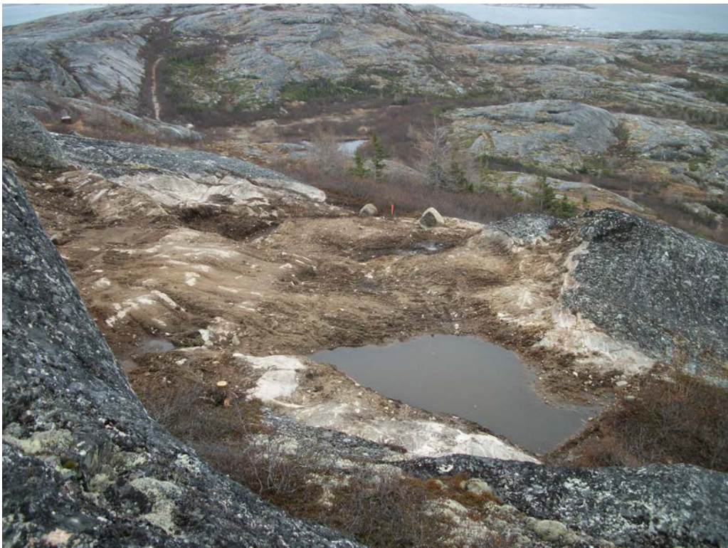
Photo 36 Main Base-Area 8 following soil removal.
