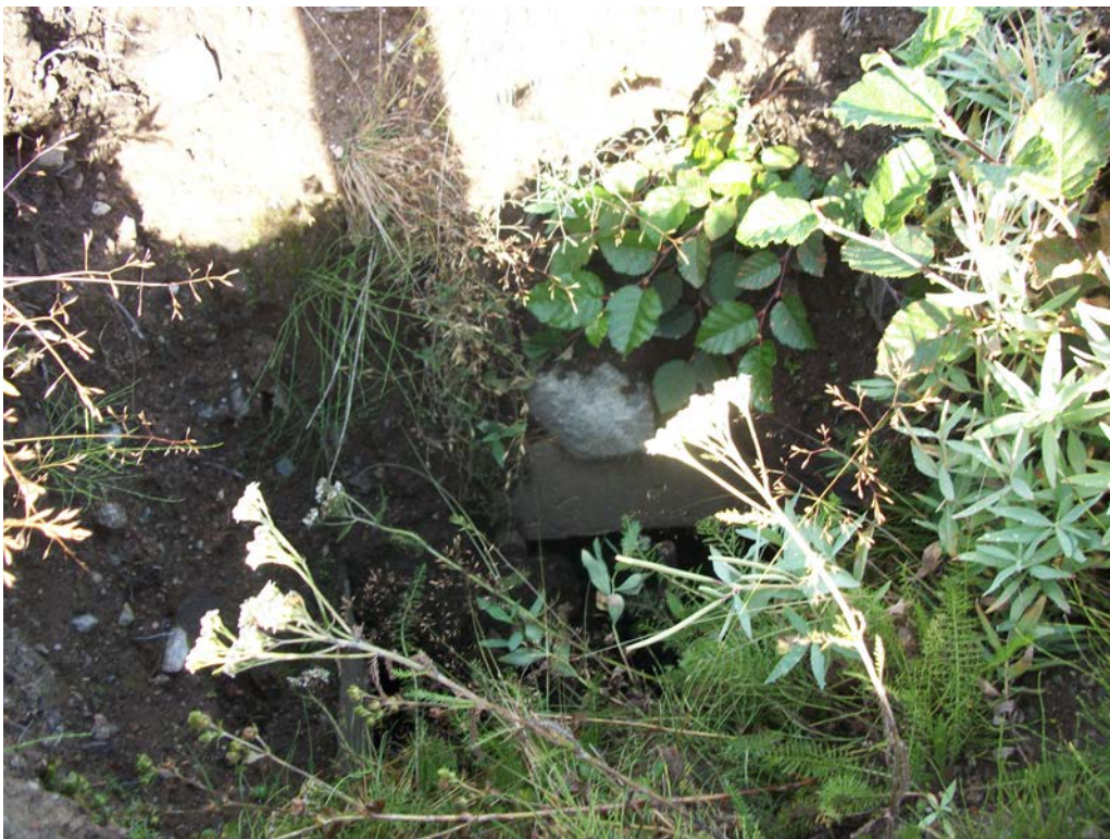
Photo 24 Concrete opening of septic tank (note: area not remediated in 2014).
