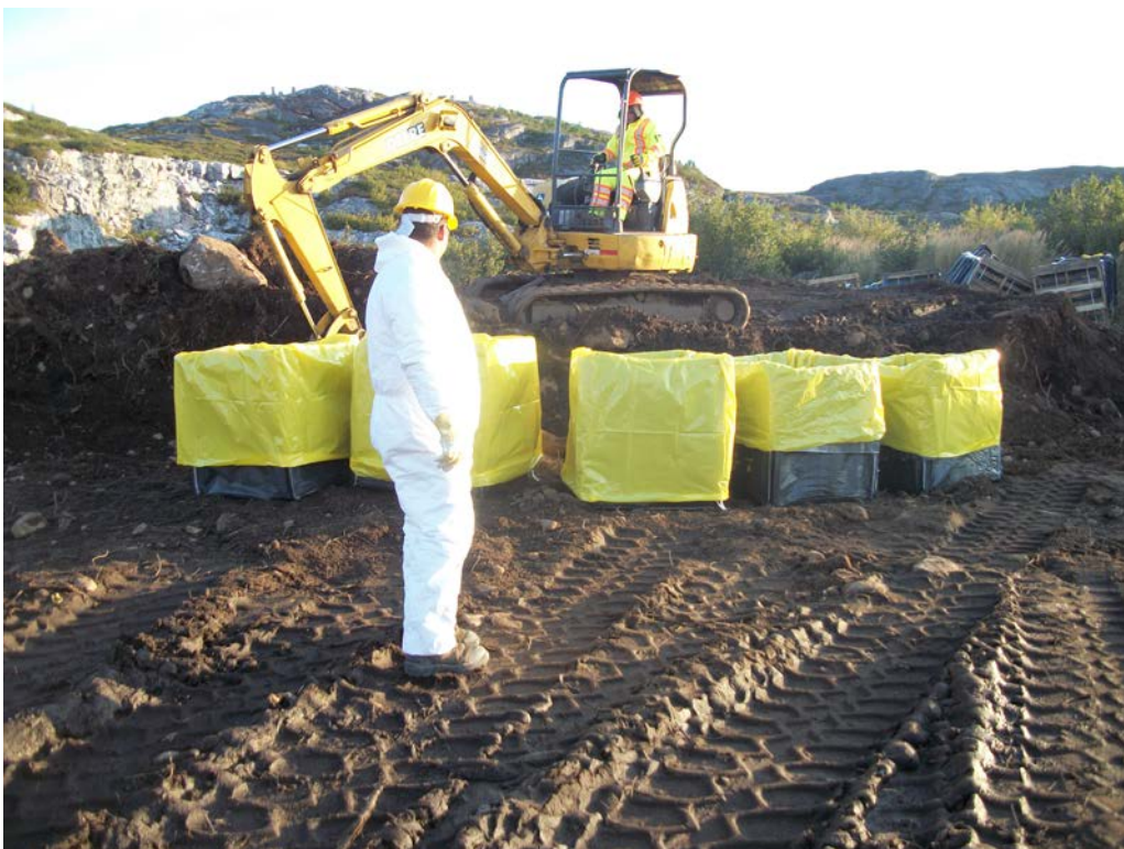
Photo 49 Loading PCB-impacted soil into enviro-bags at the Staging Area.
