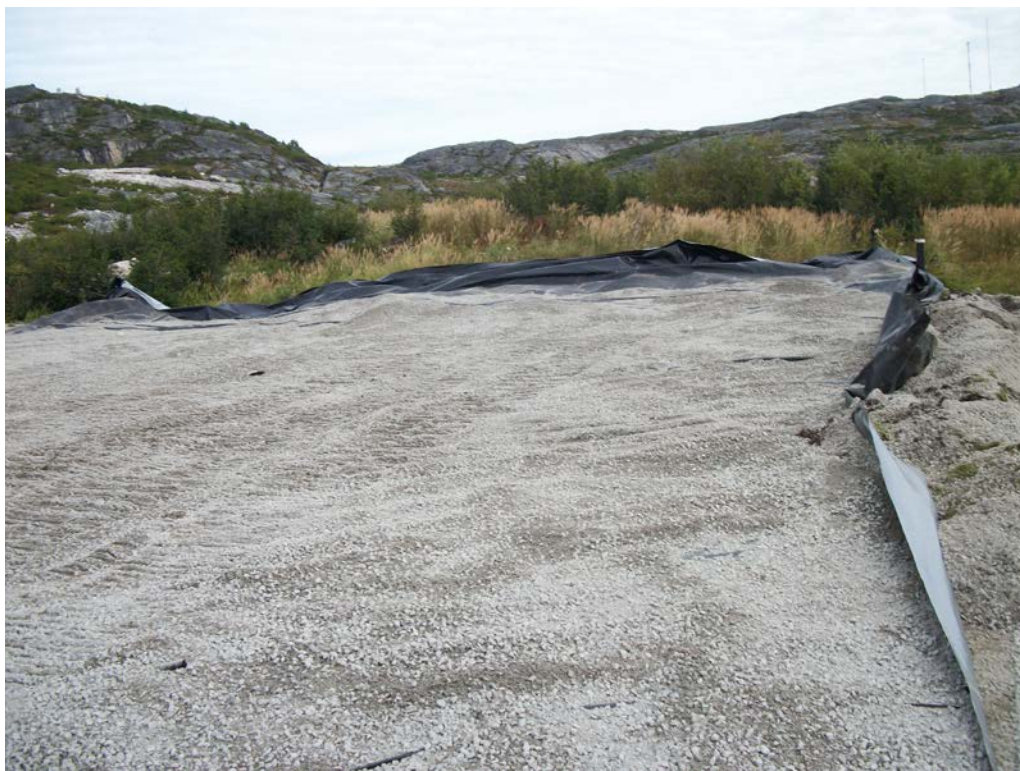
Photo 47 Staging Area liner and berm.
