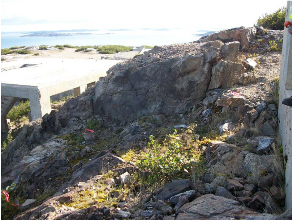
Photo 23 Main Base-Area 5, looking west, prior to grubbing (note: area not remediated in 2014).
