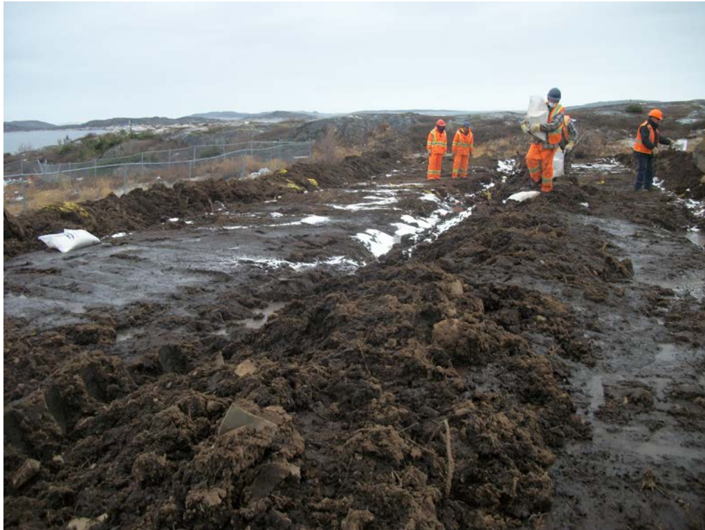
Photo 5 Addition of biopile nutrients/fertilizers.
