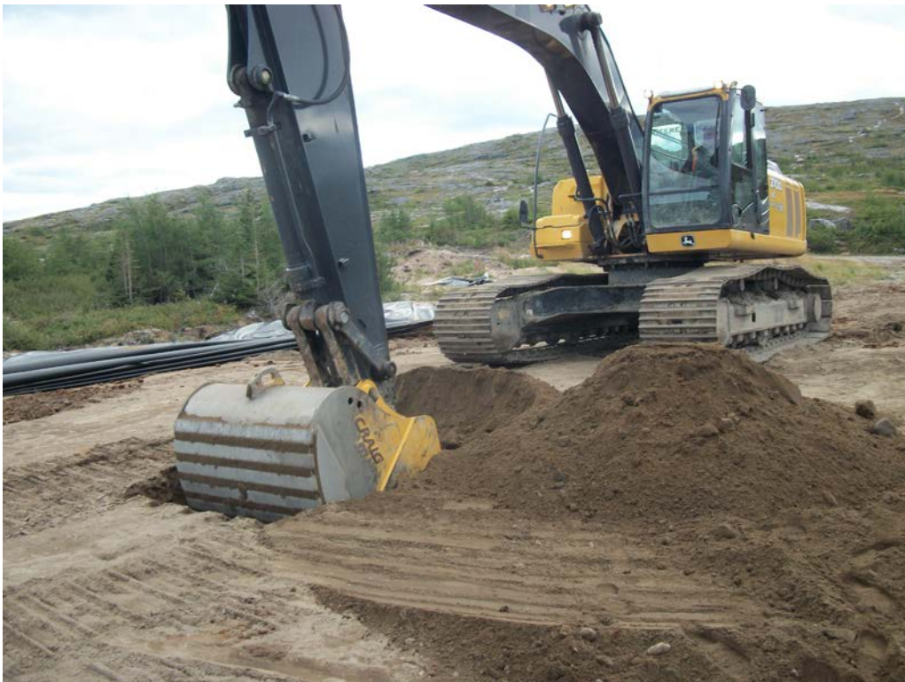
Photo 2 Test pit excavation on September 8, 2014.
