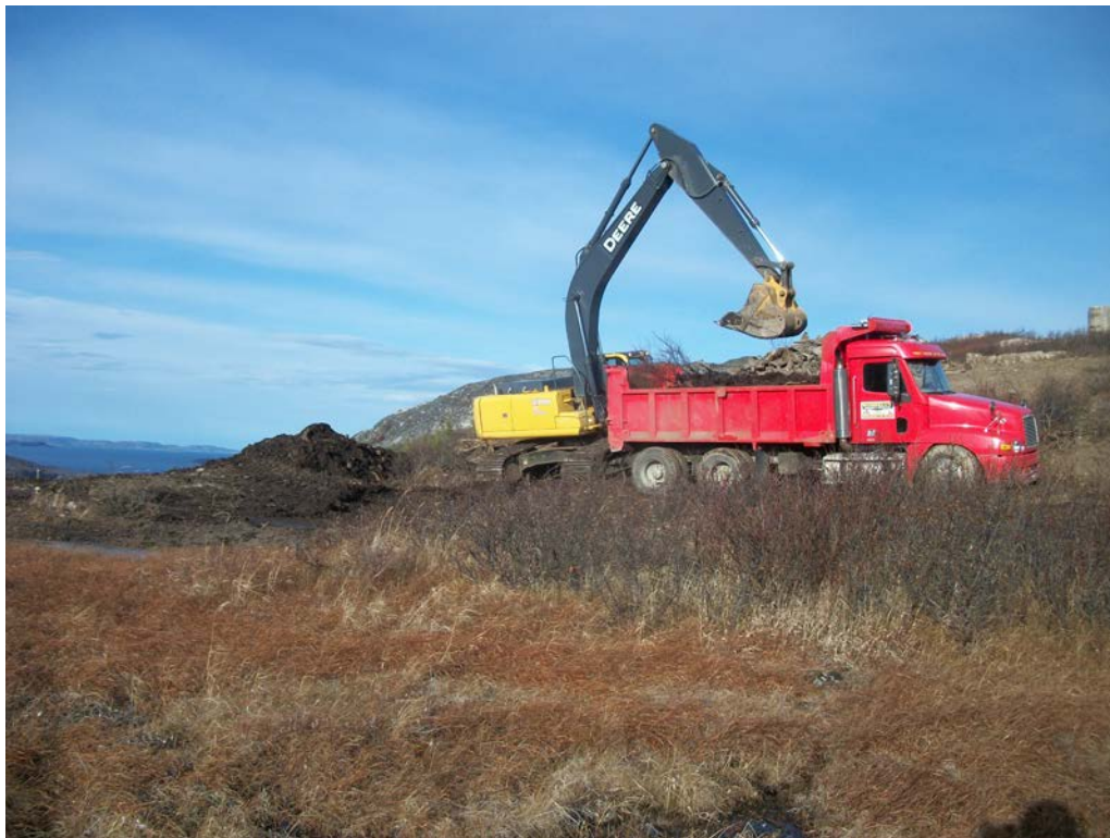
Photo 11 Soil removal at BMEWS-Area 1.
