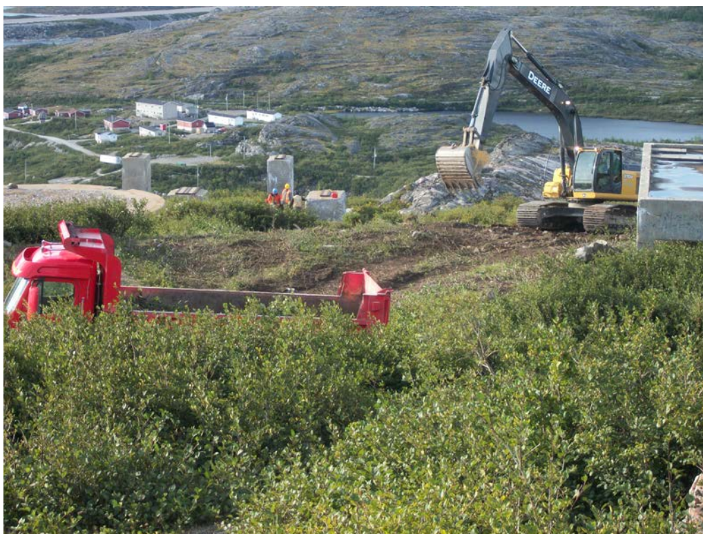
Photo 26 Grubbing at Main Base-Area 1.
