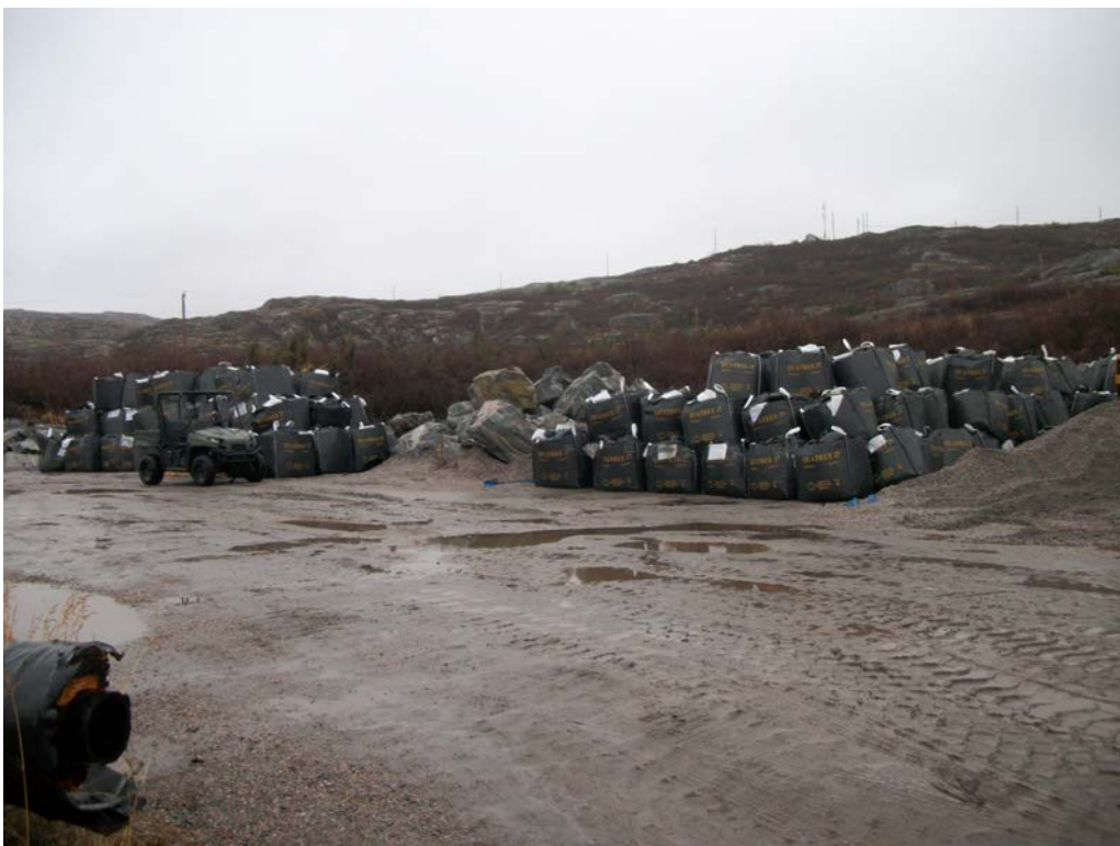
Photo 51 PCB-impacted soil bags.
