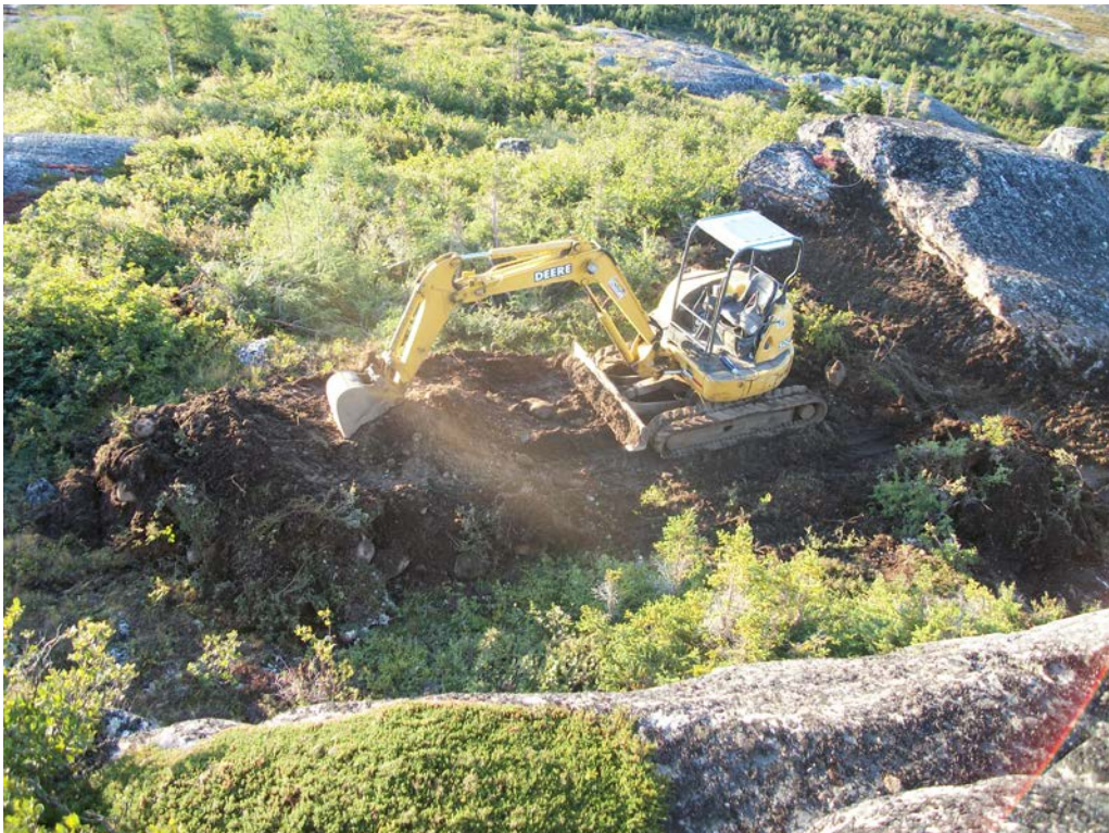
Photo 34 TPH-impacted soil removal at Main Base-Area 7.
