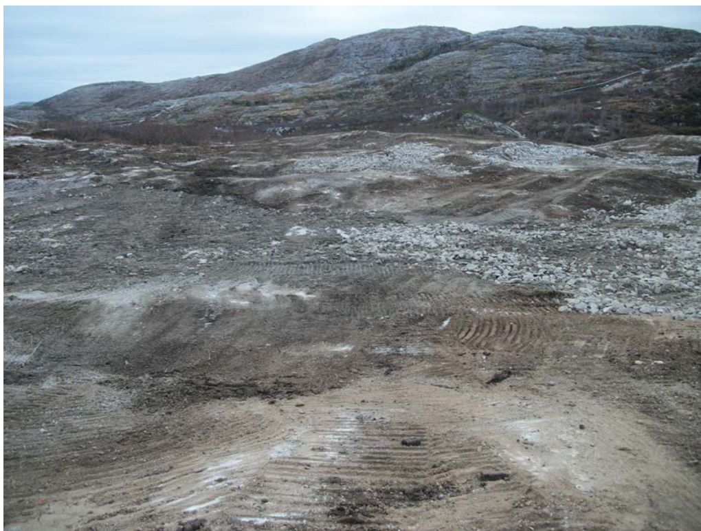
Photo 44 POL-Area 1, looking southwest, following soil removal and backfilling.
