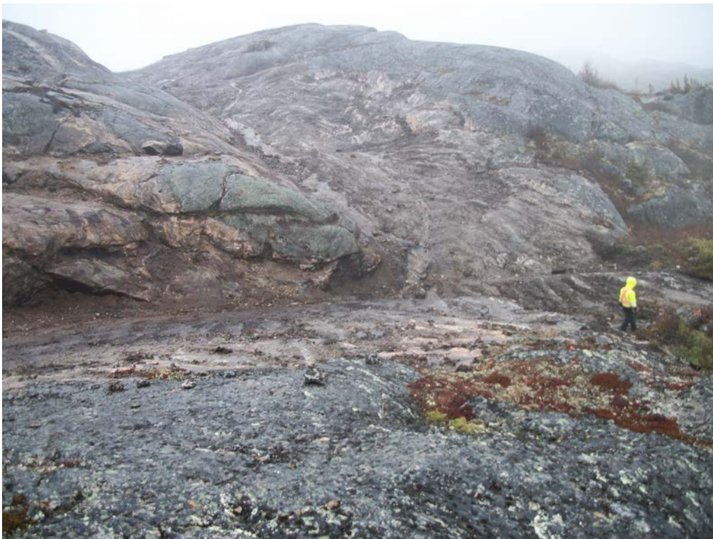
Photo 31 Main Base-Area 1 following the removal of PCB-impacted soil, looking east.
