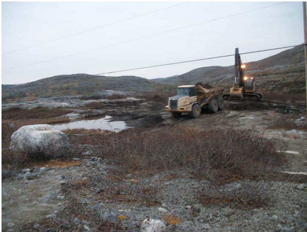
Photo 39 TPH-impacted soil removal at the POL Compound.
