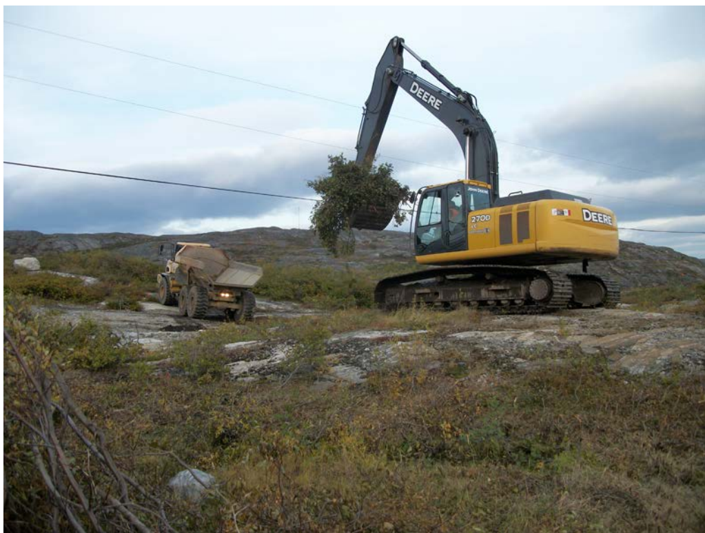
Photo 38 Removing grubblings from POL Compound site.
