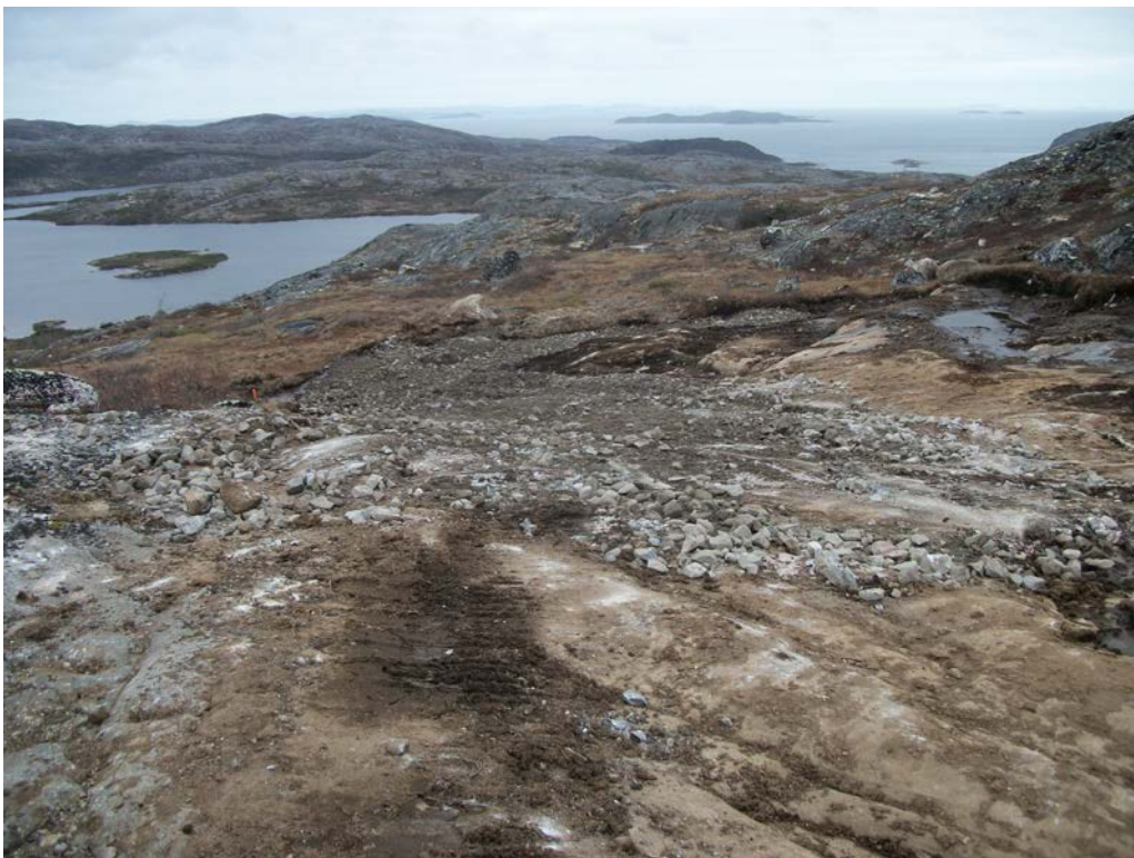
Photo 14 Lower (north) portion of BMEWS-Area 1 partially backfilled, looking north.
