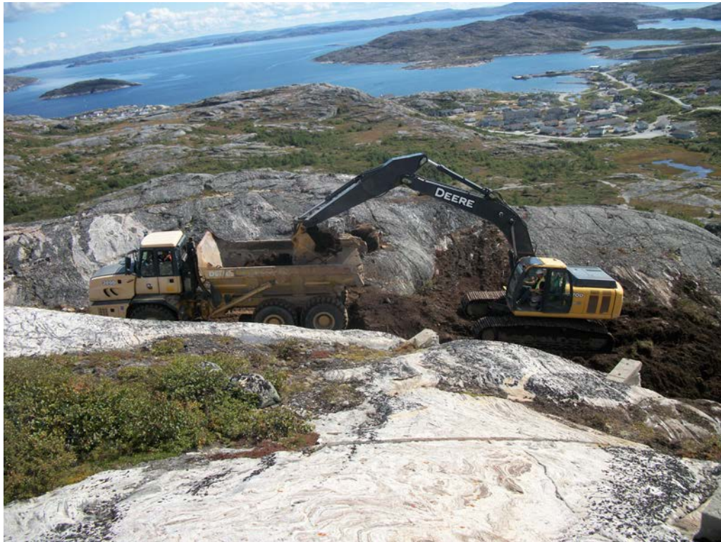
Photo 28 PCB-impacted soil removal at Main Base-Area 1.
