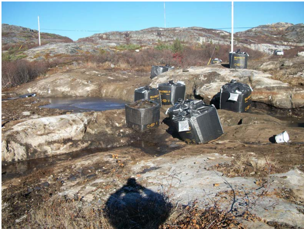
Photo 43 Bags containing soil that was removed manually removed from bedrock.
