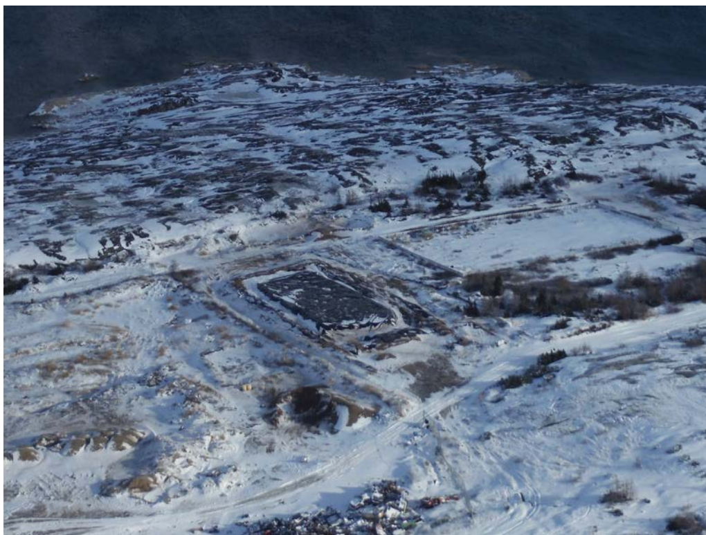
Photo 6 Aerial photo taken of the biopile on November 14, 2014.
