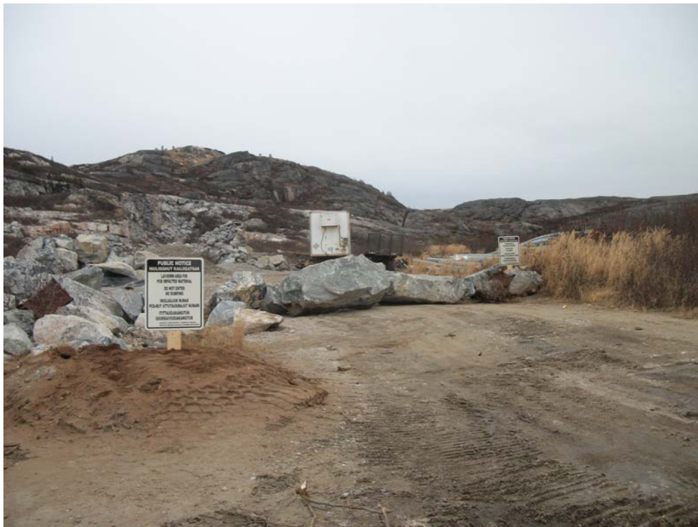
Photo 58 Signs installed at the entrance to the Laydown/Staging Area at Pit No. 1 and boulders blocking access.
