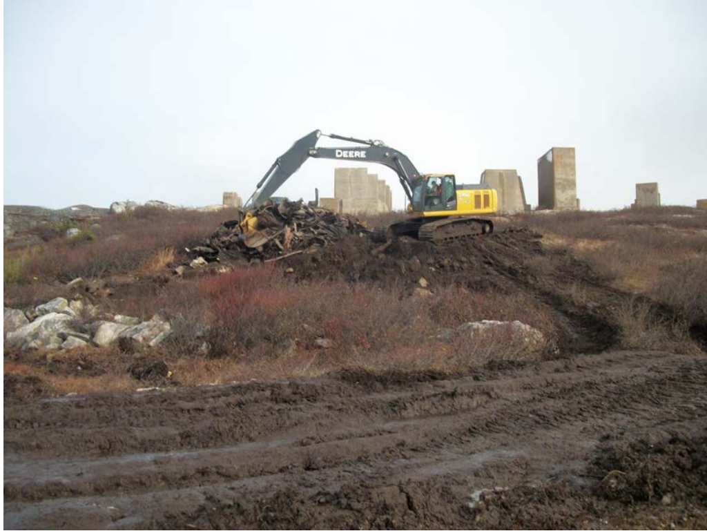
Photo 15 Removal of metal at BMEWS-Area 2.
