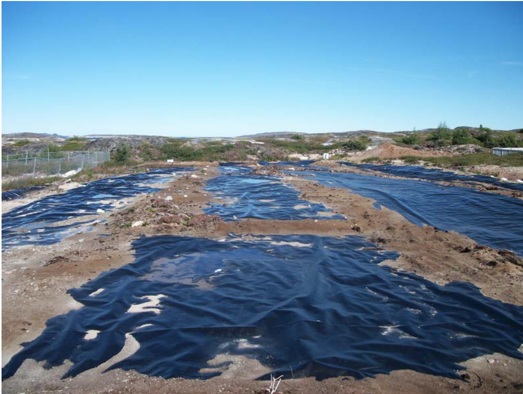
Photo 1 Biopile prior to dismantling in Year 4.
