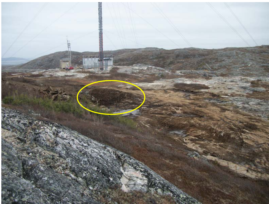
Photo 12 Upper (south) portion of BMEWS-Area 1 following soil removal, looking south. Circle shows area requiring additional soil removal.
