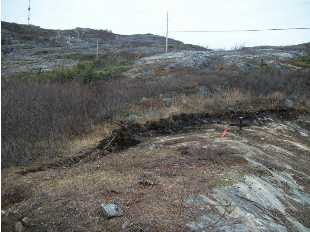
Photo 41 POL-Area 1 during soil removal, looking north in the vicinity of MW-21.
