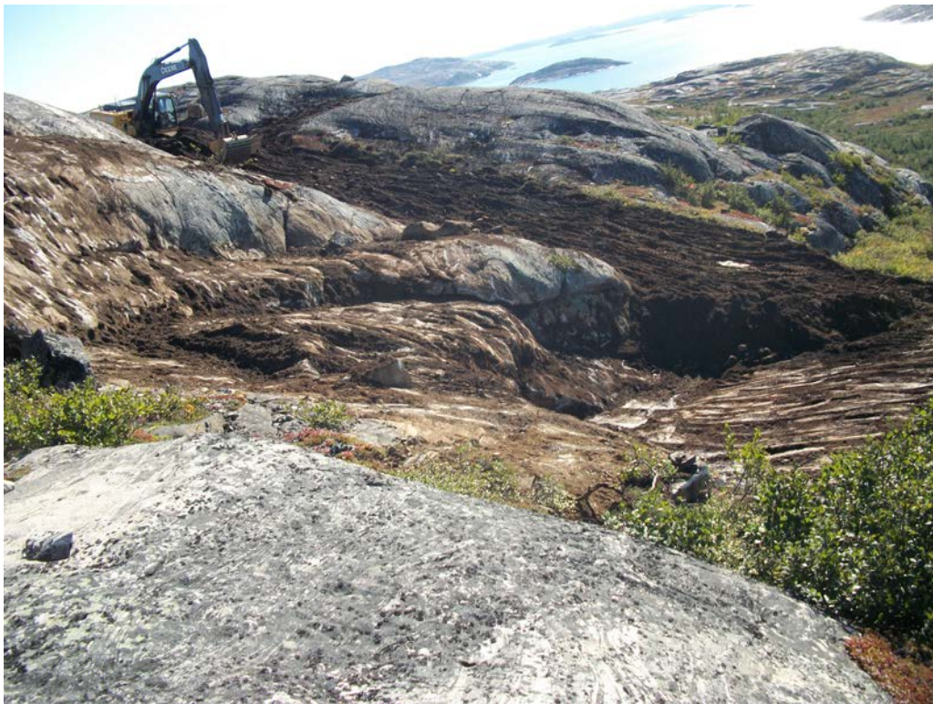
Photo 27 PCB-impacted soil removal at Main Base-Area 1.
