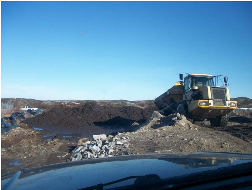
Photo 4 Placement of TPH-impacted soil in the biopile containment cell.
