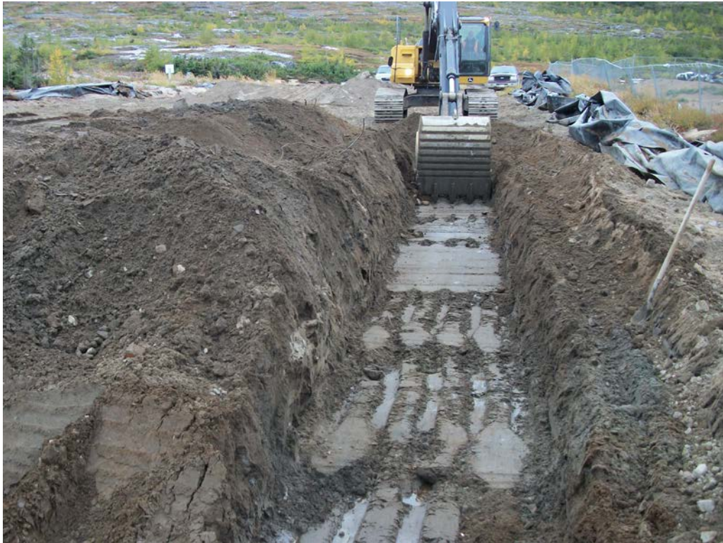
Photo 3 Removal of treated soil from the biopile.
