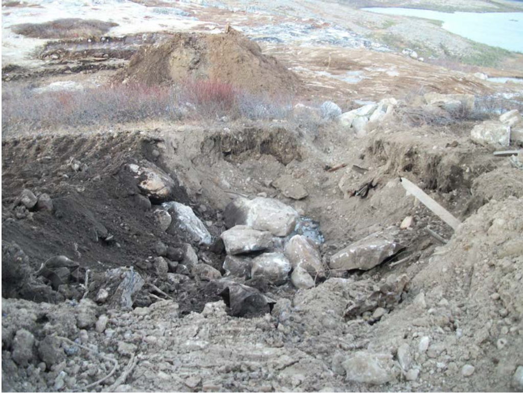
Photo 17 BMEWS-Area 2 excavation, looking west.
