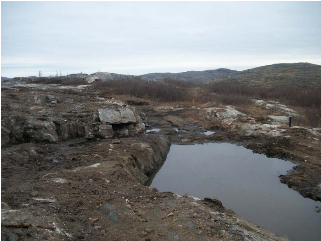
Photo 42 POL-Area 1 during soil removal, looking south in the vicinity of MW-22.
