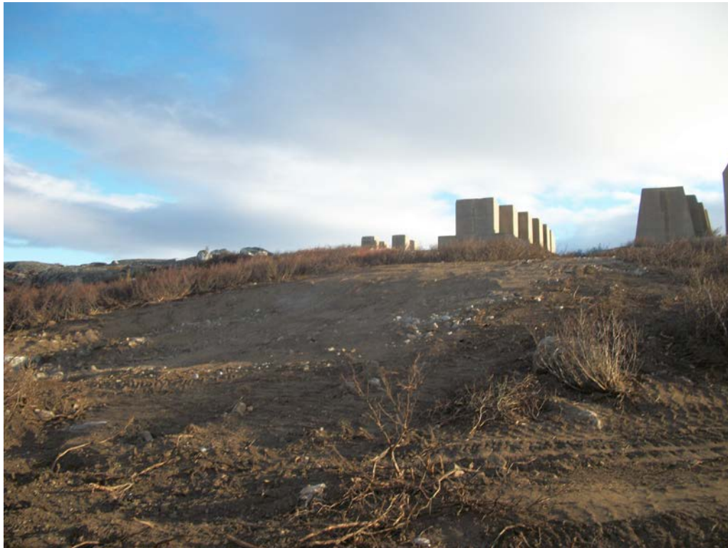
Photo 18 BMEWS-Area 2 excavation following backfilling, looking east.
