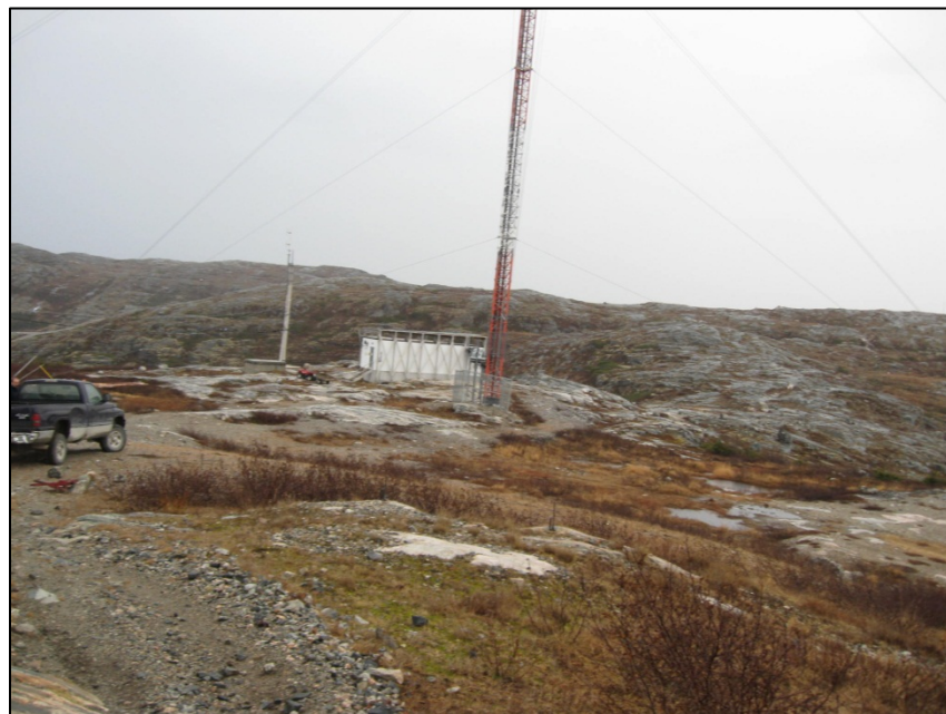
Photo 4. Areas of TPH impacted soil requiring remediation (MW-64, BMEWS-TP2, BMEWS-TP3 and BMWES-TP4, and TP-102 and BMEWS-TP11), looking southwest towards the Aliant trailer and tower.
