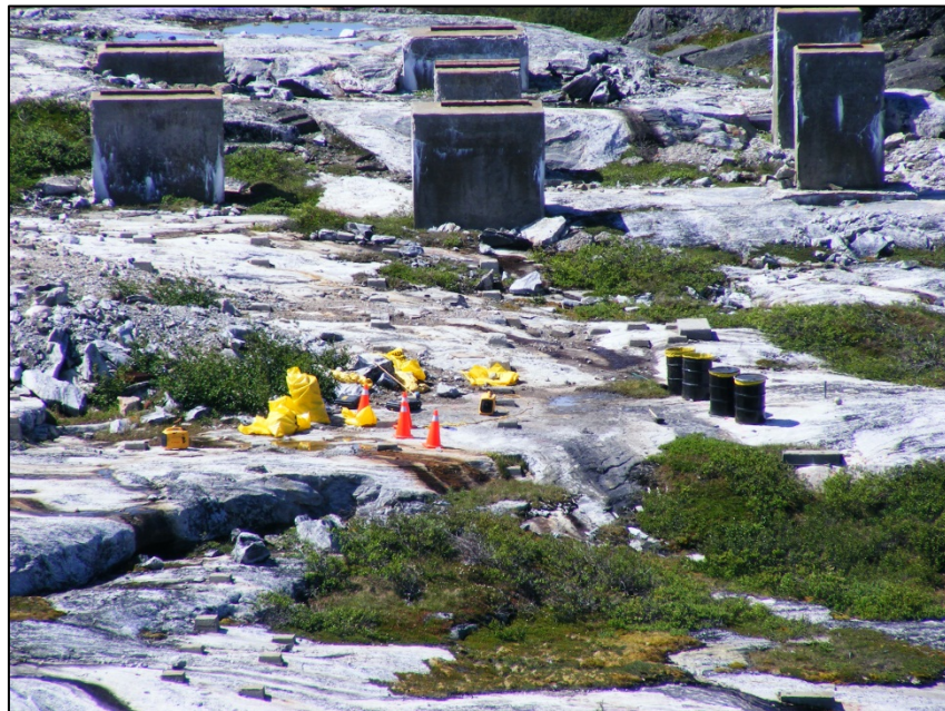
Photo 5. 2009 photo of Old Base 1 during removal of tar-like material, looking southwest
