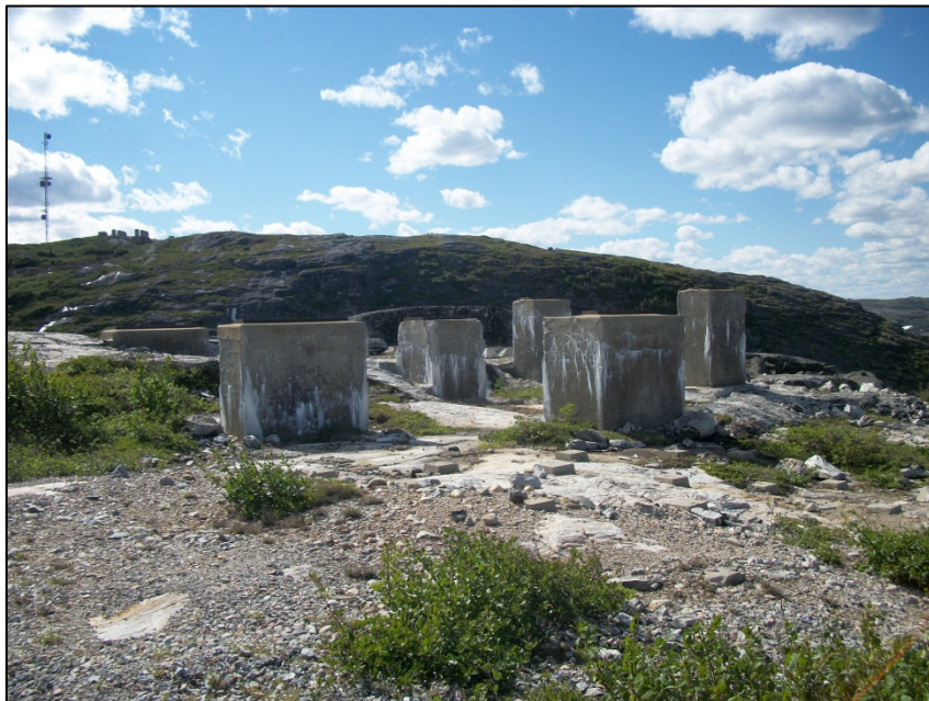
Photo 7. Photo showing soil cover near foundation bases.
