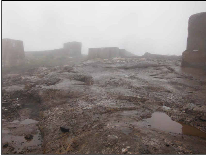
Photo 3. Uneven bedrock surface encountered during remediation at BMEWS in 2013.
