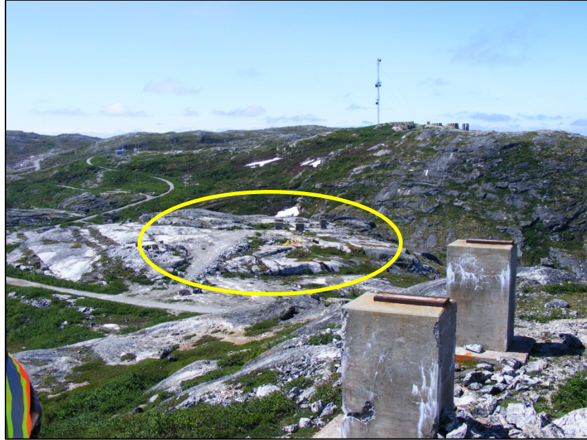
Photo 4. 2009 photo of Old Base 1 during removal of tar-like material, looking southwest.
