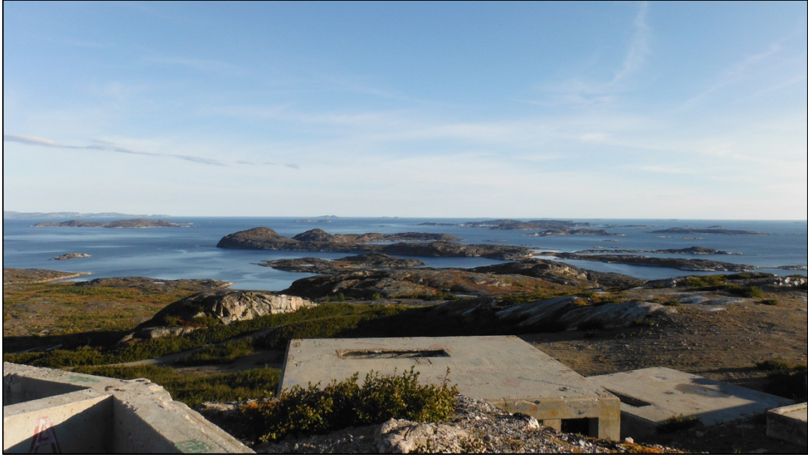
Photo 5. Concrete foundations currently remaining at Main Base, looking northeast.
