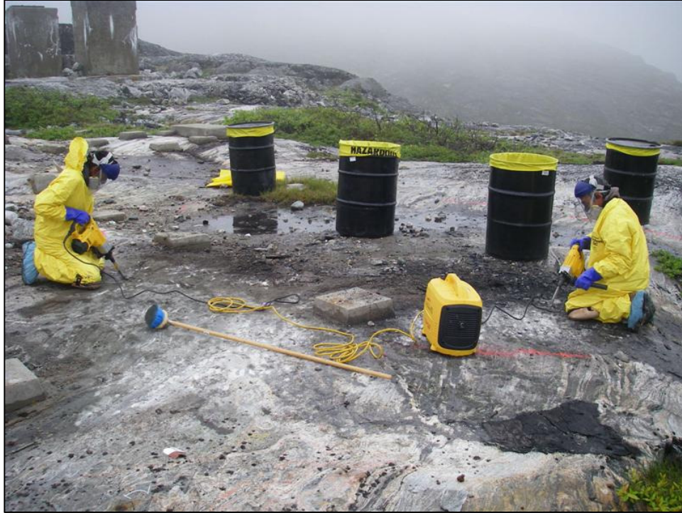
Photo 11. 2009 photo of Main Base during removal of tar-like material, looking east.
