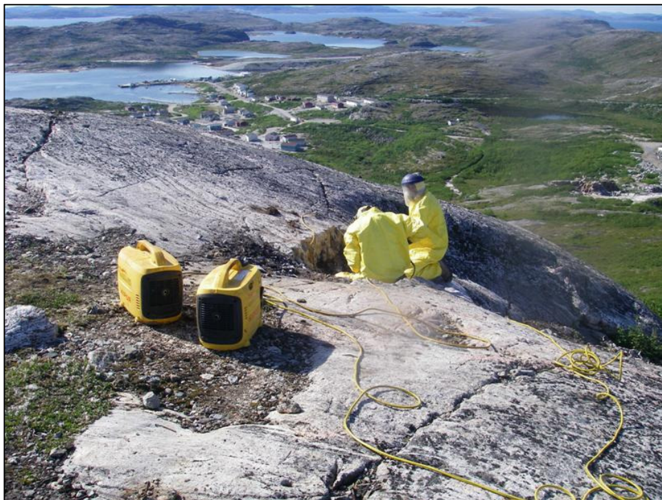
Photo 12. 2009 photo of Main Base during removal of tar-like material, looking south.
