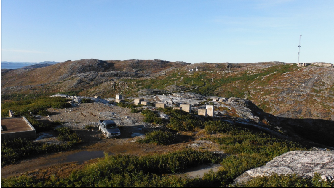
Photo 3. Concrete foundations currently remaining at Main Base, looking southwest.
