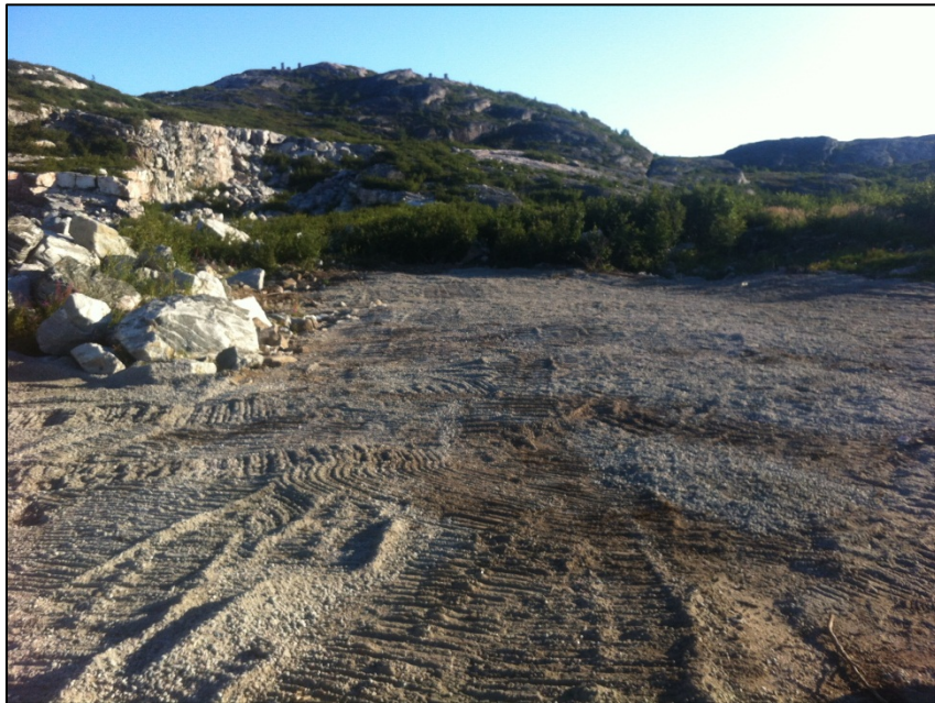
Photo 4. Pit No. 1 following bag removal, surficial soil removal and backfilling in 2013, looking north.
