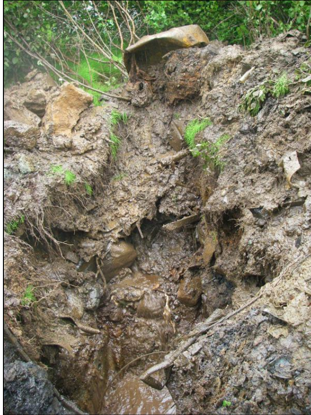
Photo 7. Test pit TP-233 during excavation in 2009.
