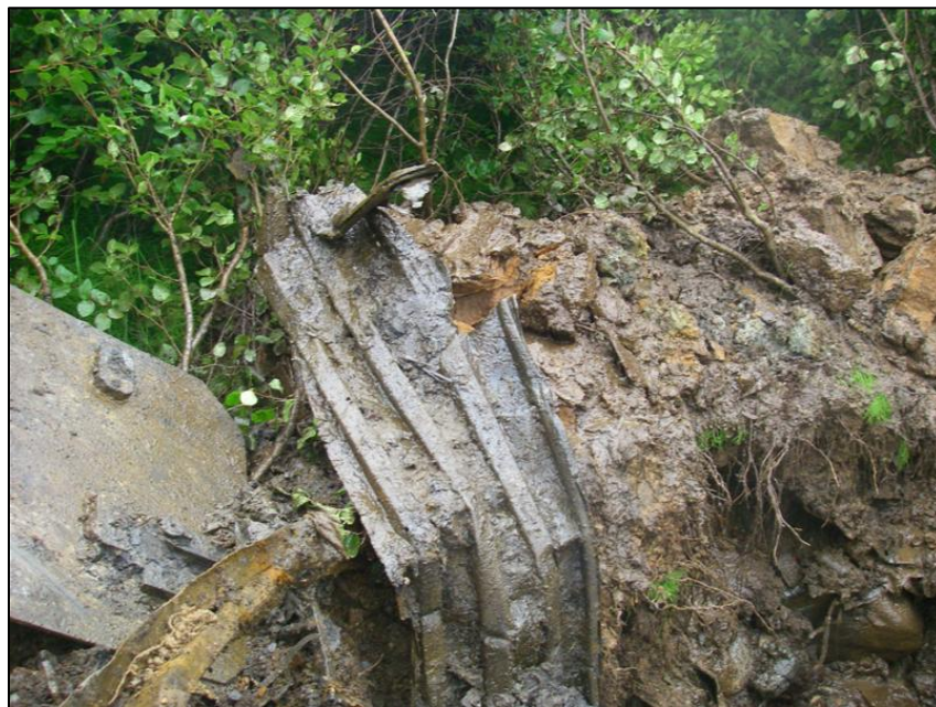
Photo 8. Test pit TP-233 during excavation in 2009.
