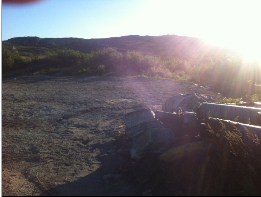
Photo 3. Pit No. 1 following bag removal, surficial soil removal and backfilling in 2013, looking northeast.
