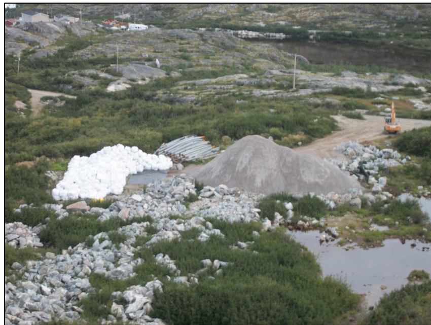
Photo 2. Pit No. 1 in 2012 during temporary storage of PCB-impacted soil (in soil bags) and backfill material, looking south.
