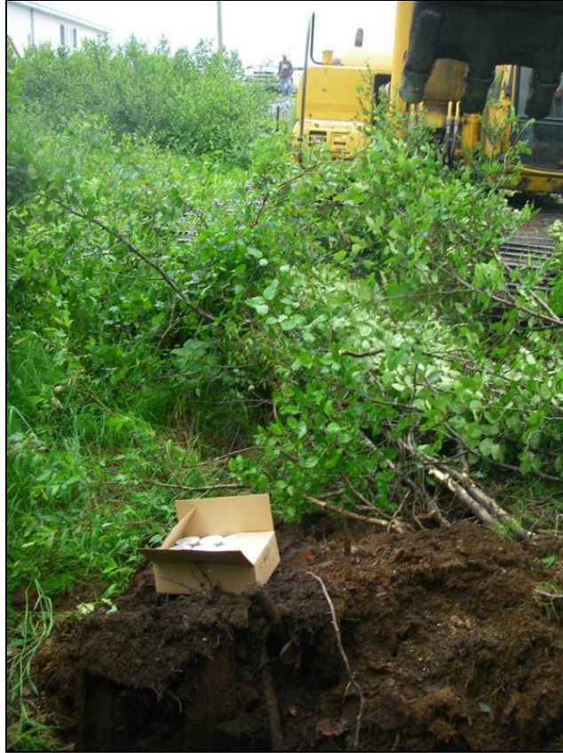
Photo 5. Test pit TP-229 during excavation in 2009.
