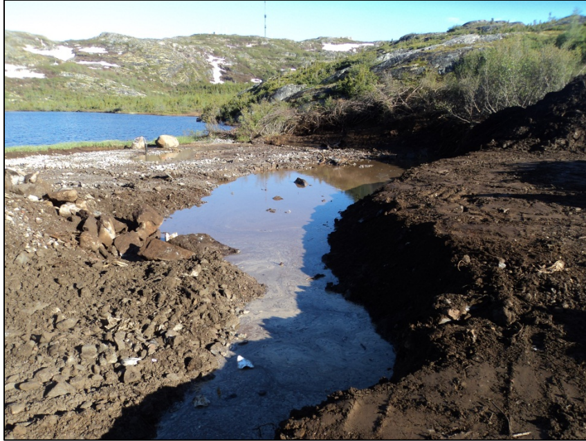
Photo 1. Old Dump Pond remedial excavation on July 2, 2013, looking northwest.
