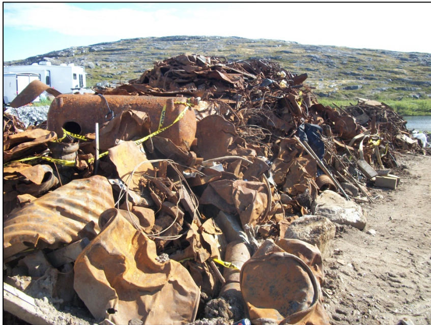
Photo 2. Buried metal removed from the PCB remedial excavation at Old Dump Pond.
