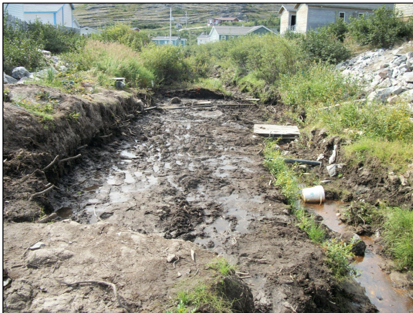
Photo 2. Lower portion of the stream on during soil removal in 2012.
