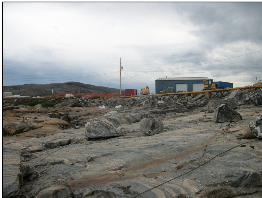
Photo 2. Remediated shoreline at Pipeline/Wharf area in 2012.
