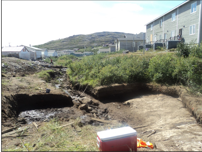
Photo 1. Upper portion of the stream on during soil removal in 2012.
