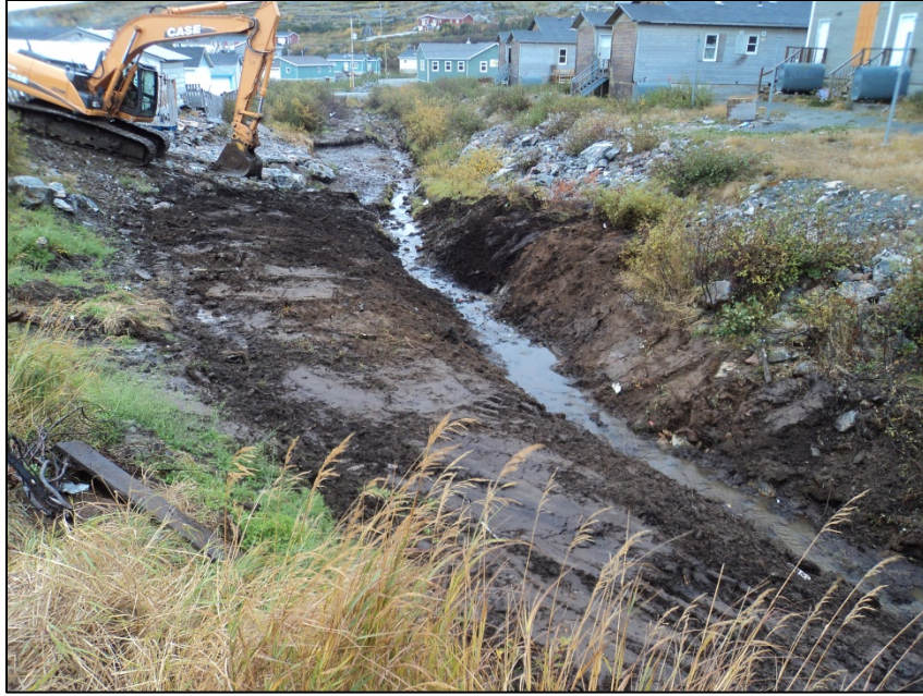
Photo 3. Stream site reinstatement in 2012, looking southwest.
