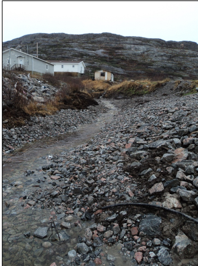
Photo 4. Stream site following backfilling in 2012, looking north.
