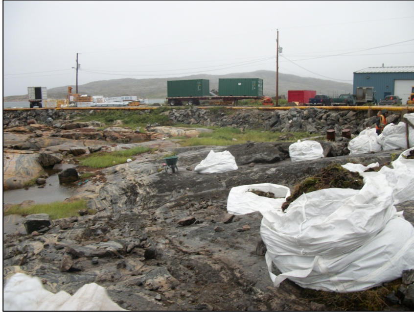
Photo 1. Shoreline at Pipeline/Wharf area during soil removal in 2012.
