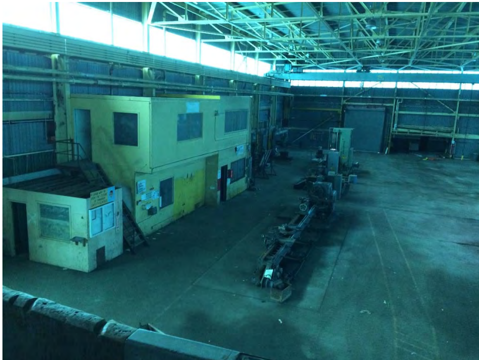
Photo 8: Carpenters & Joiners Building – Main Floor view of the Machine Shop area with offices and lunch room at the left and pipe stock room at the top right.
