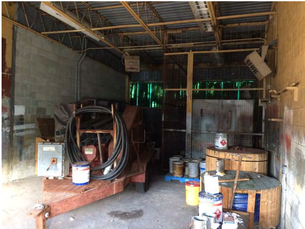
Photo 20: Services Building – Paint Shop or Water Blast Room where flaking or peeling paint or potential ACMs were not observed.
