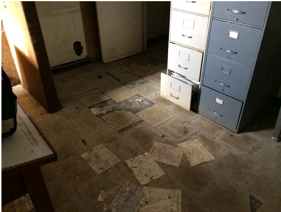
Photo 7: Carpenters & Joiners Building – Second Floor Electrician’s Office where the vinyl floor tile had no ACMs, tile mastic confirmed ACM, teal green walls and white ceilings had no lead-based paint.
