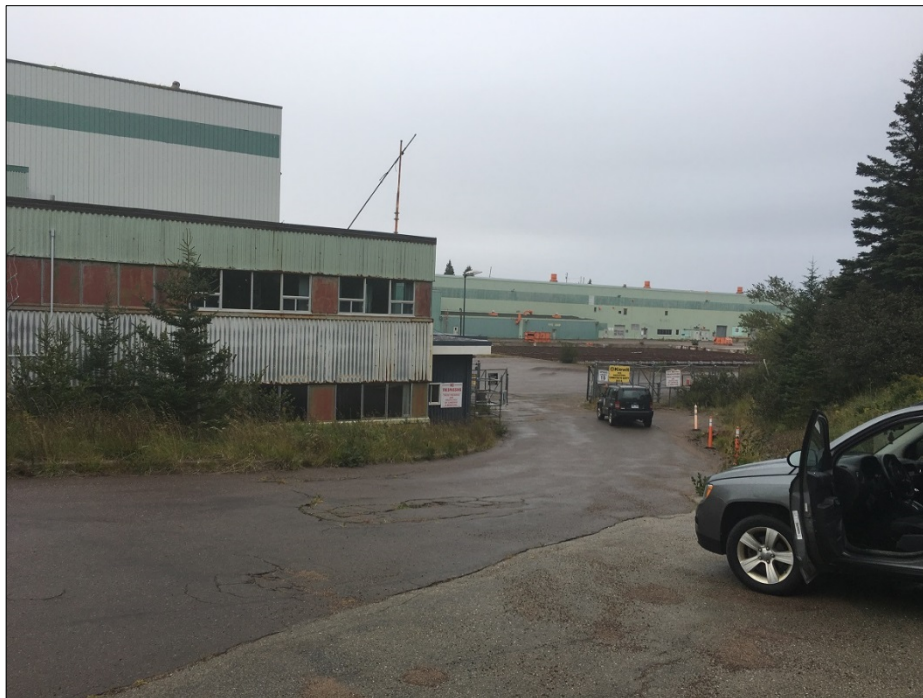
Photo 1 – View, looking northeast of the main Site entrance at the Marystown Shipyard Main Administration and Security Office (MASO) with the Machine Shop and General Stores Building in the background.
