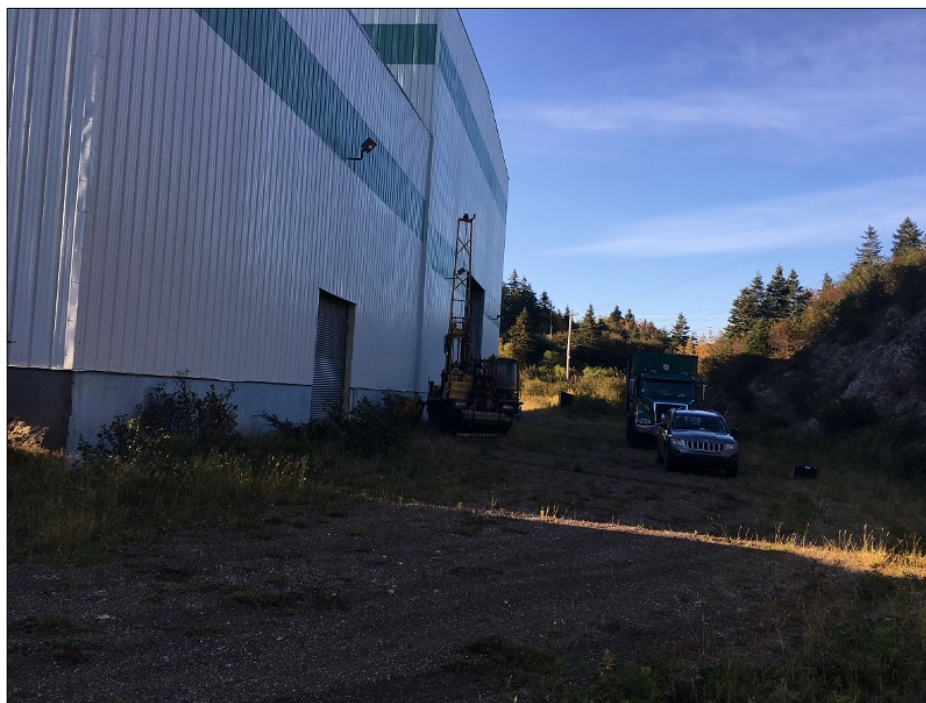
Photo 6 – View, looking west, of the Marystown Shipyard Assembly and Erection Building (MAEB) while drilling MAEB-MW1-2018.
