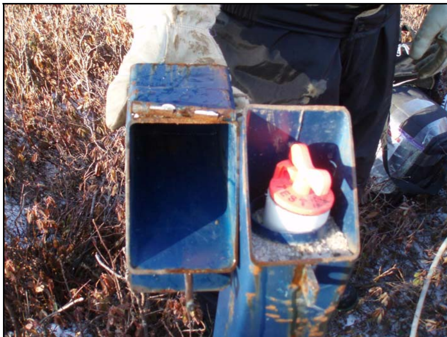
Photo 2: MW-07 broken top hinge.
