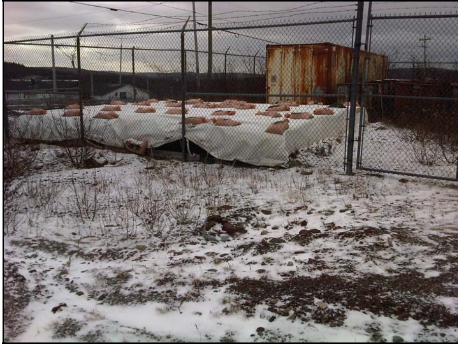
Photo 13: Stored LLDPE geomembrane: south side of secure enclosure.
