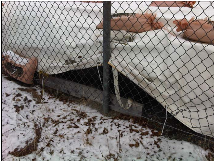
Photo 14: Tarp lifted and LLDPE geomembrane exposed, south storage pad.
