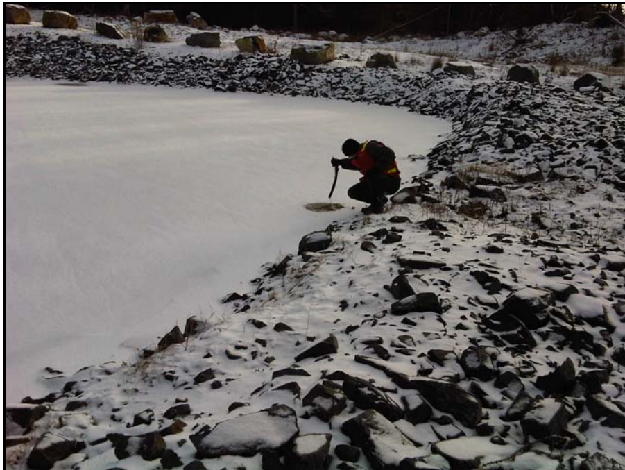
Photo 12: Leachate pond dam.
