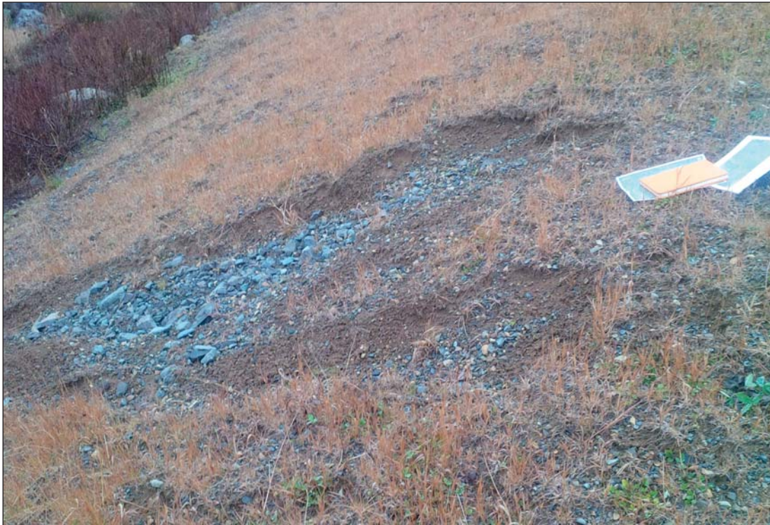
Photo 3 View of the west slope of the PCB disposal area, showing some mass wasting of the slope.
