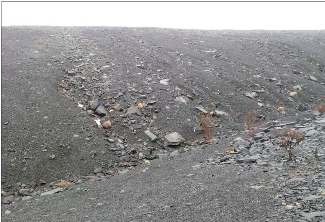
Photo 2 View of the waste disposal site slope, showing erosion of the landfill cover.
