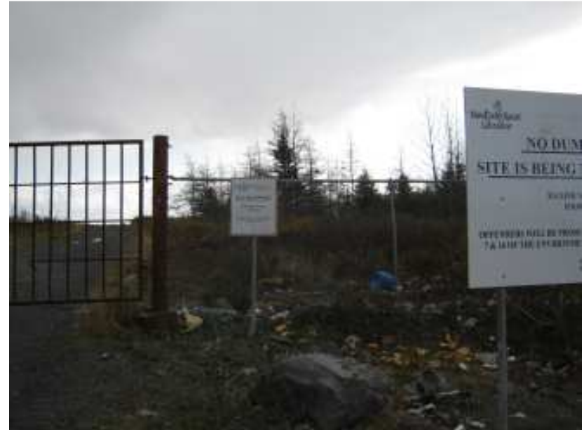
Photo 6 – Current gate and chain link fencing.
