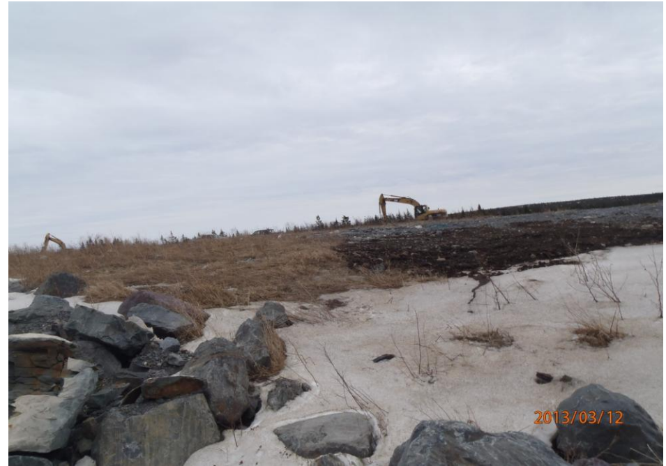
6. Looking southeast at the edge of the PCB Area.
