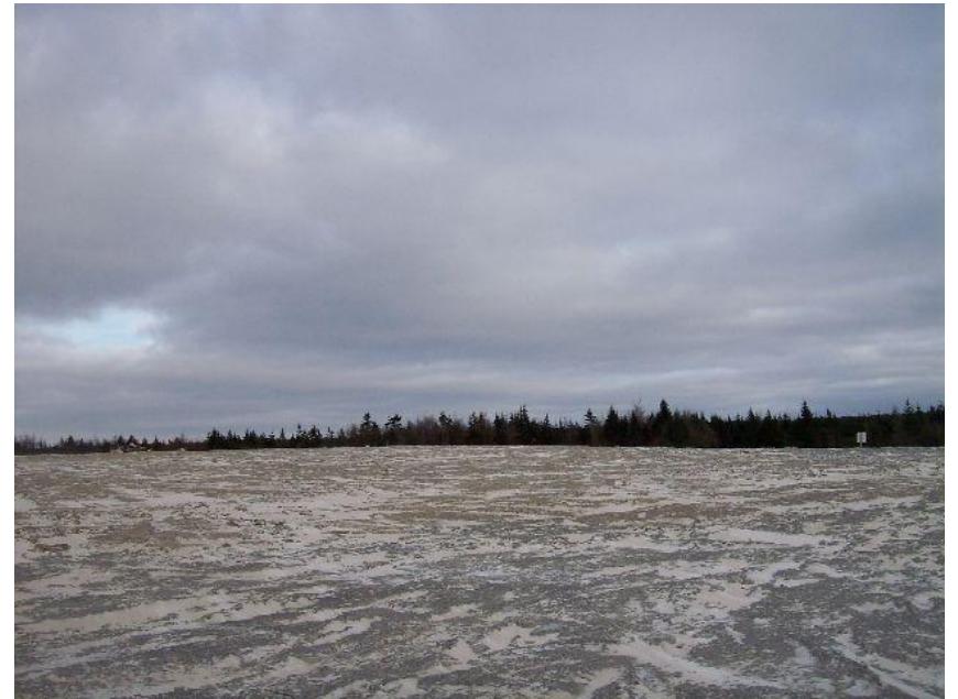
Photo 28 – Covered trench (Dec 14)
