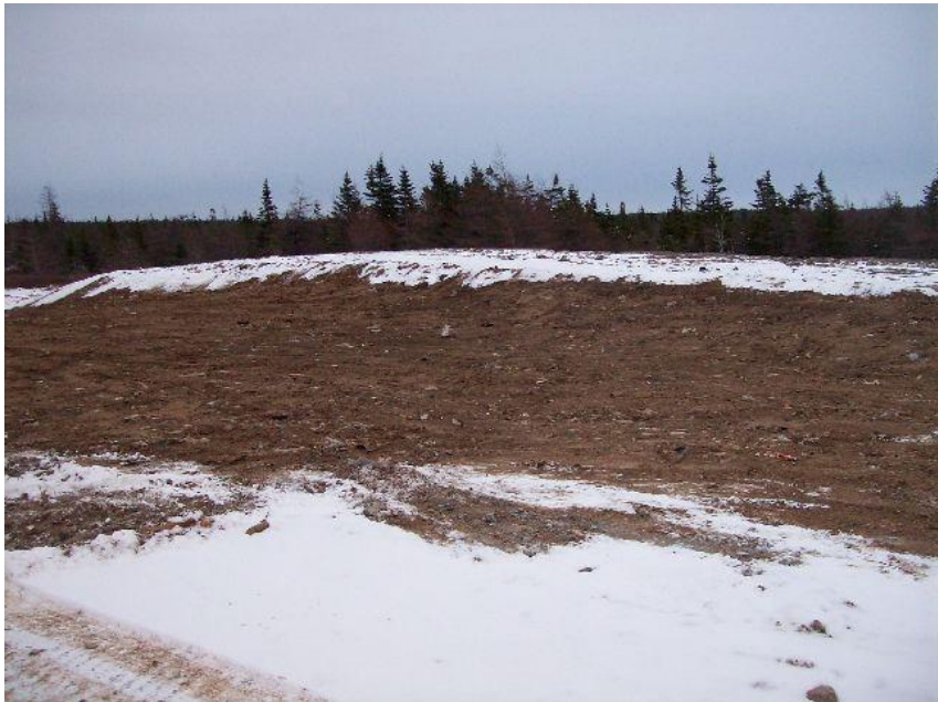
Photo 31 – Covered boulders (Dec 22)
