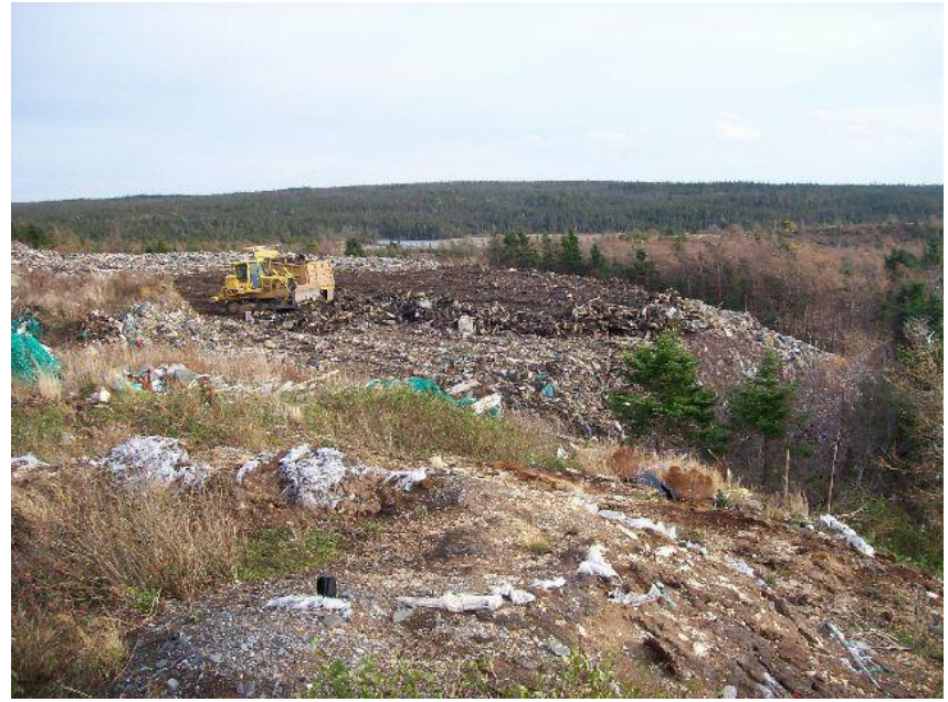
Photo 6 – South facing slope being re-graded
