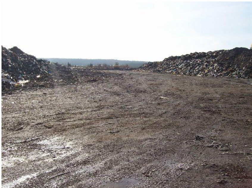
Photo 3 – After windrowing the waste to obtain access to the borrow (Nov 14)
