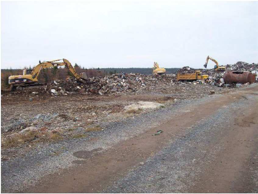
Photo 5 – Metals stockpile being removed (Nov 14)
