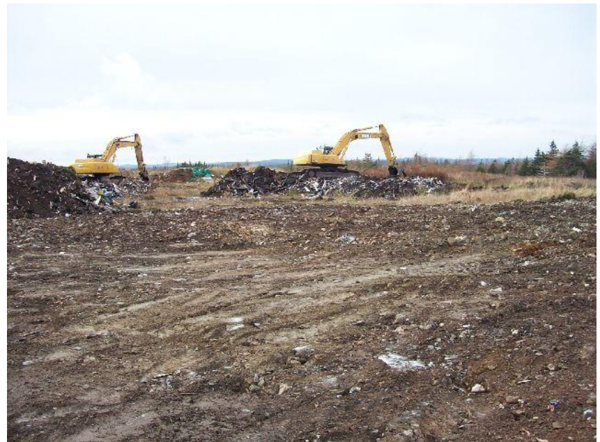
Photo 4 – Northeast stockpile being moved to the East stockpile (Nov 14)
