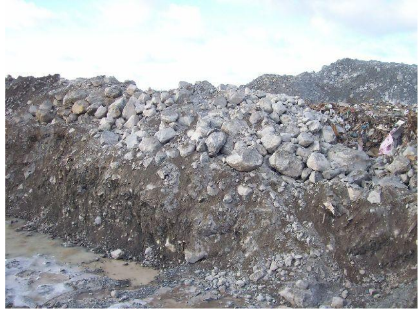
Photo 14 – Typical boulders encountered during trench excavation (Nov 22)
