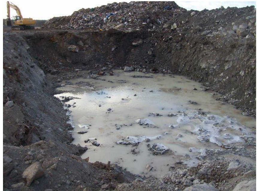
Photo 12 – Typical trench conditions (Nov 22)
