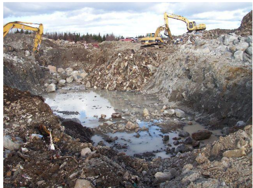
Photo 16 – East waste stockpile being placed in trench (Nov 22)
