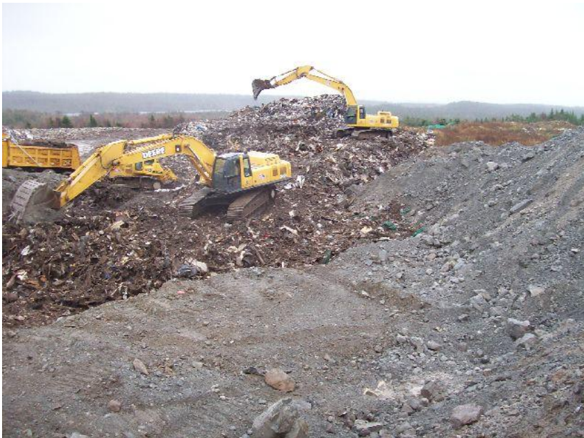
Photo 11 – Excavator and dozer placing waste in the trench (Nov 18)
