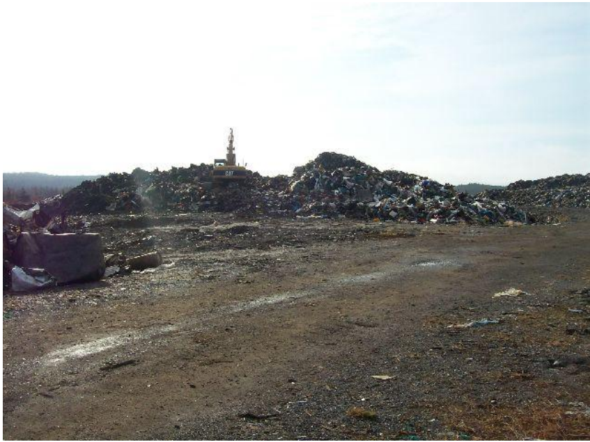
Photo 1 – West waste stockpile (Nov 14)
