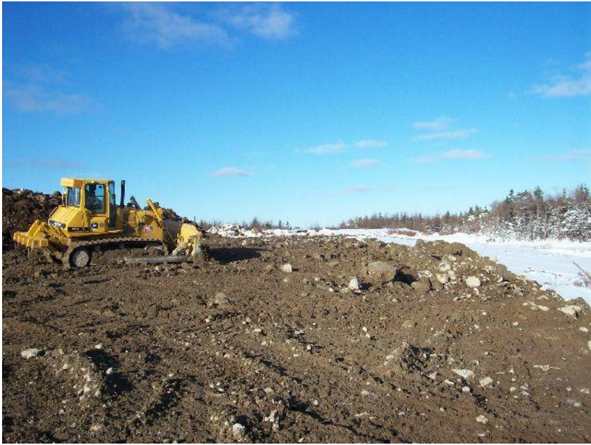
Photo 21 – Typical placement of interim cover (Nov 25)
