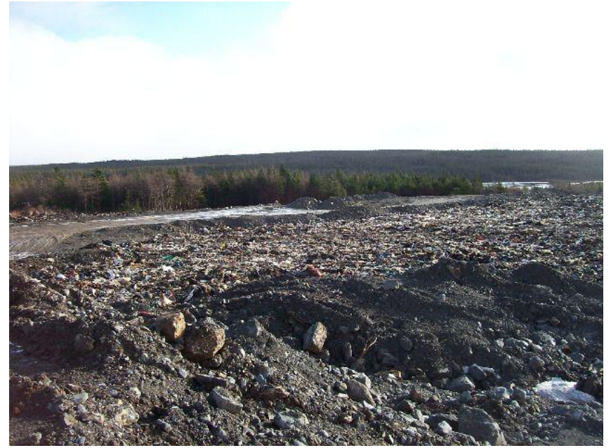
Photo 22 – East stockpile removed (looking Southeast) (Nov 29)
