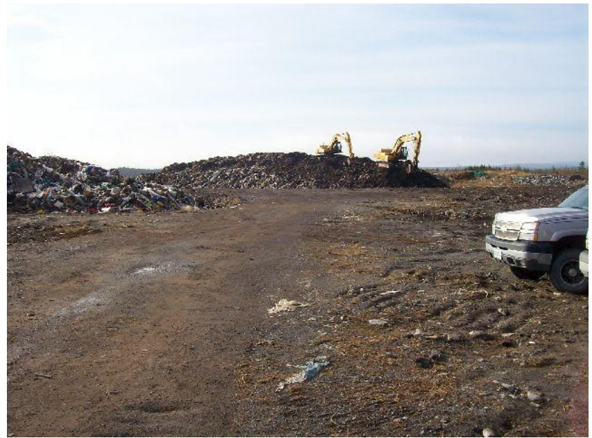
Photo 2 – East waste stockpile (Nov 14)
