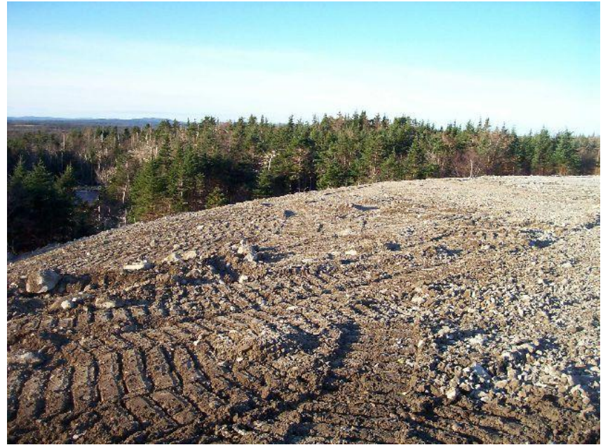
Photo 18 – South slope covered and compacted (Nov 23)
