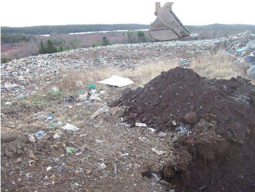
Photo 15 – East slope re-graded (looking South) (Nov 22)
