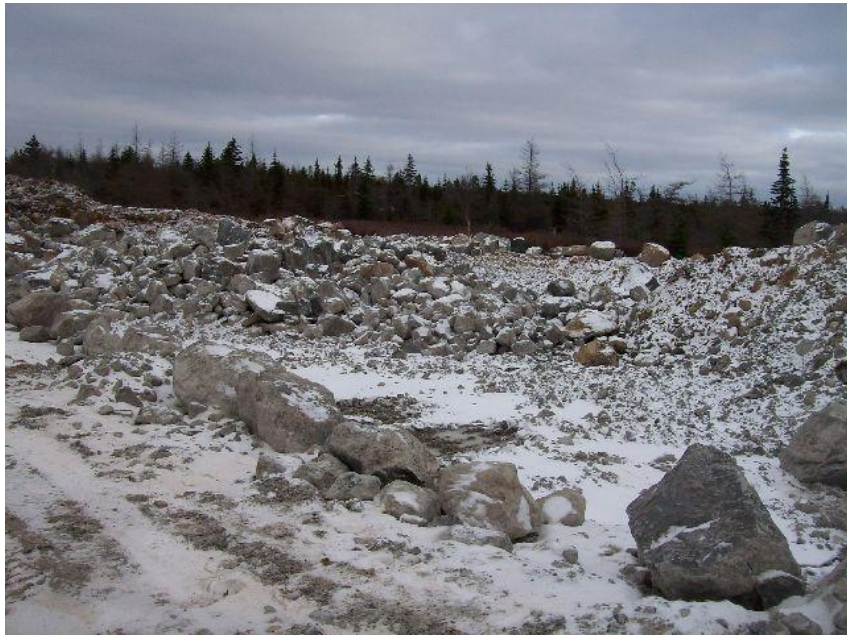
Photo 27 – Typical boulders encountered in main borrow source (Dec 14)
