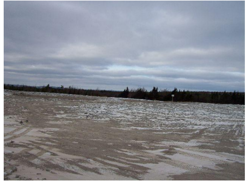
Photo 26 – Sawdust area covered (looking Southwest) (Dec 14)
