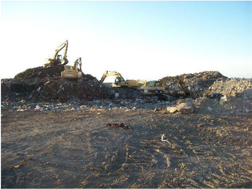
Photo 17 – Excavators placing waste from the East stockpile into the trench (Nov 23)
