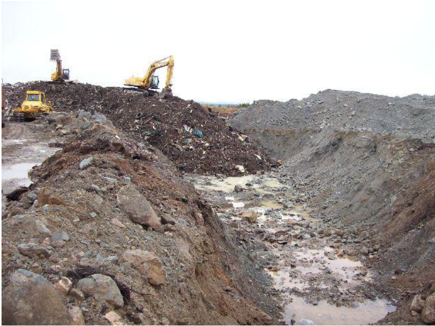
Photo 9 – Waste being placed in the trench (Nov 17)
