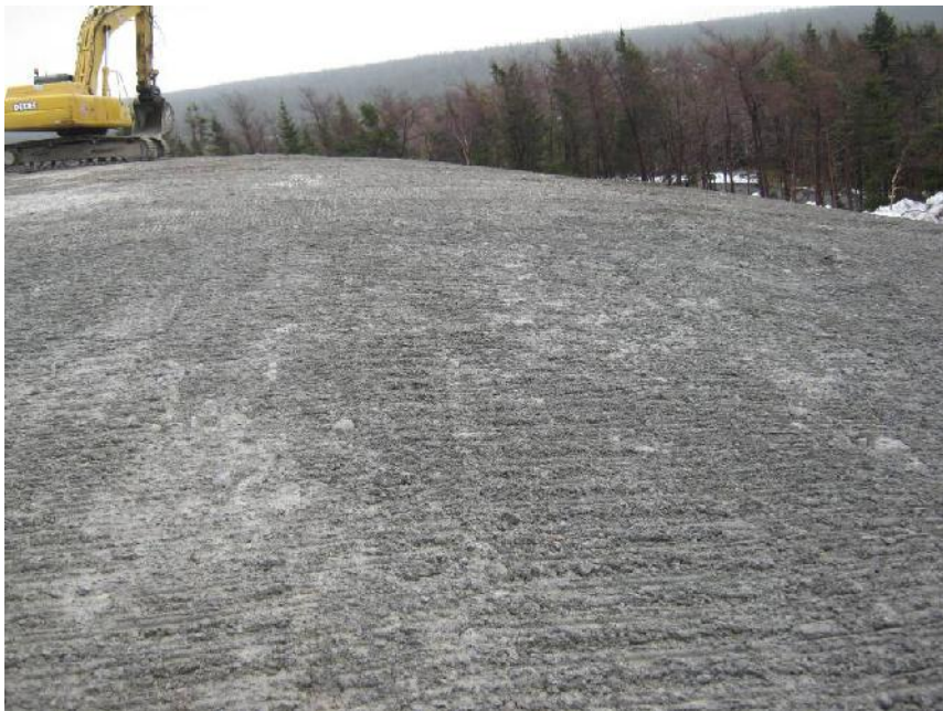
Photo 7 – Compaction of fill material on south slope looking east.
