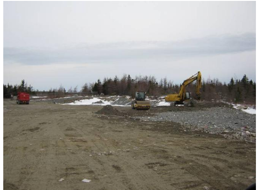
Photo 6 – Boulder section during fill placement.
