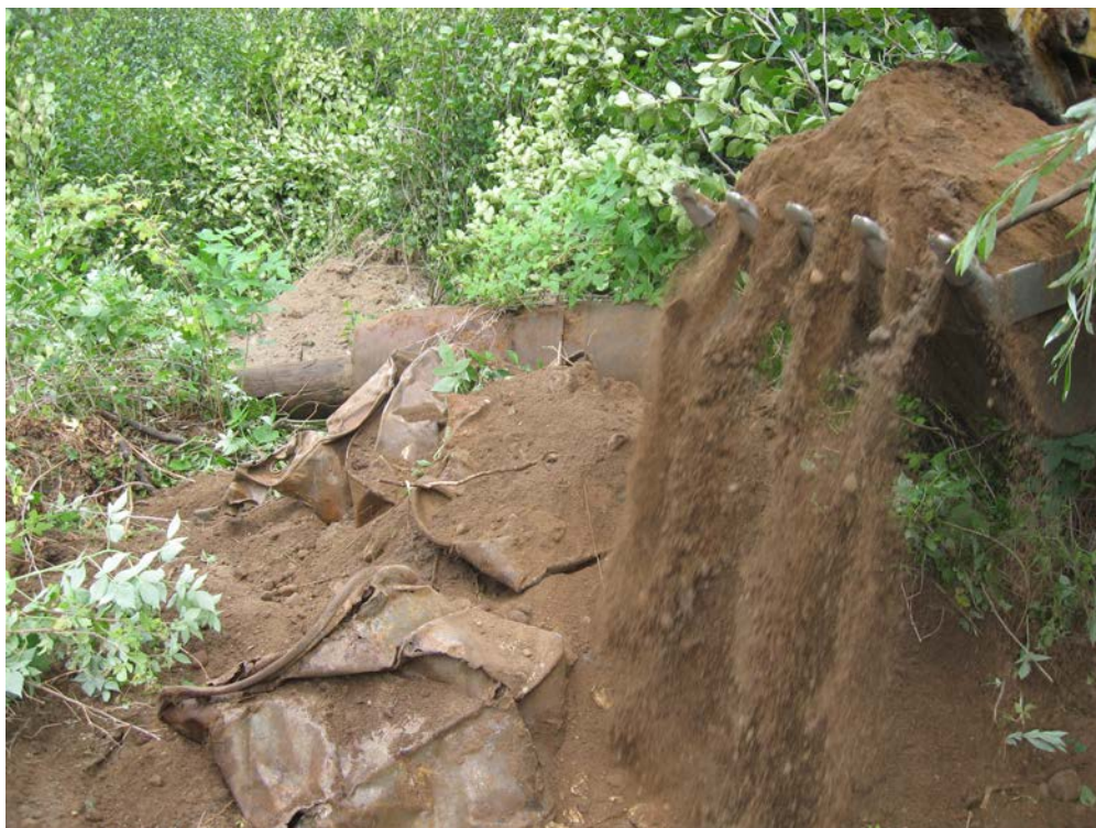
Photo 6 View of drums and metal debris encountered in 09-TP62
