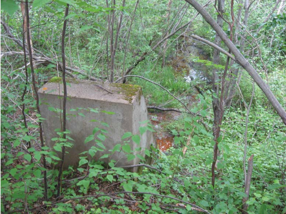
Photo 1 View of sewer outlet looking north
