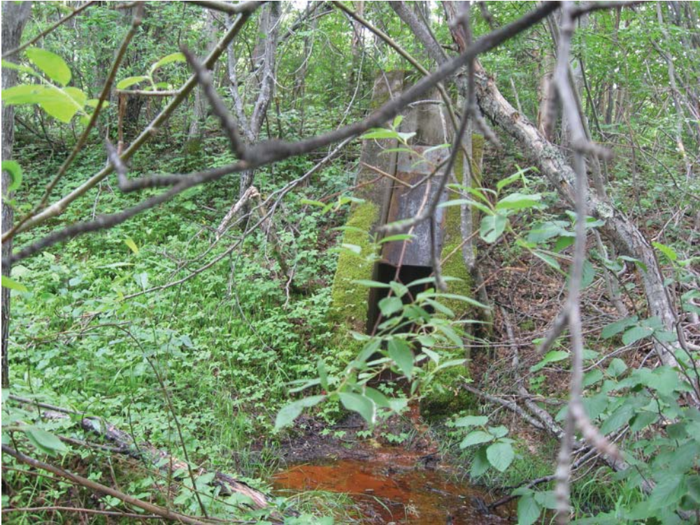
Photo 2 View of sewer outlet looking south
