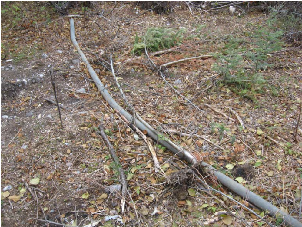
Photo 2 View of surface debris at the site (partially buried pipe, 09-SD9)
