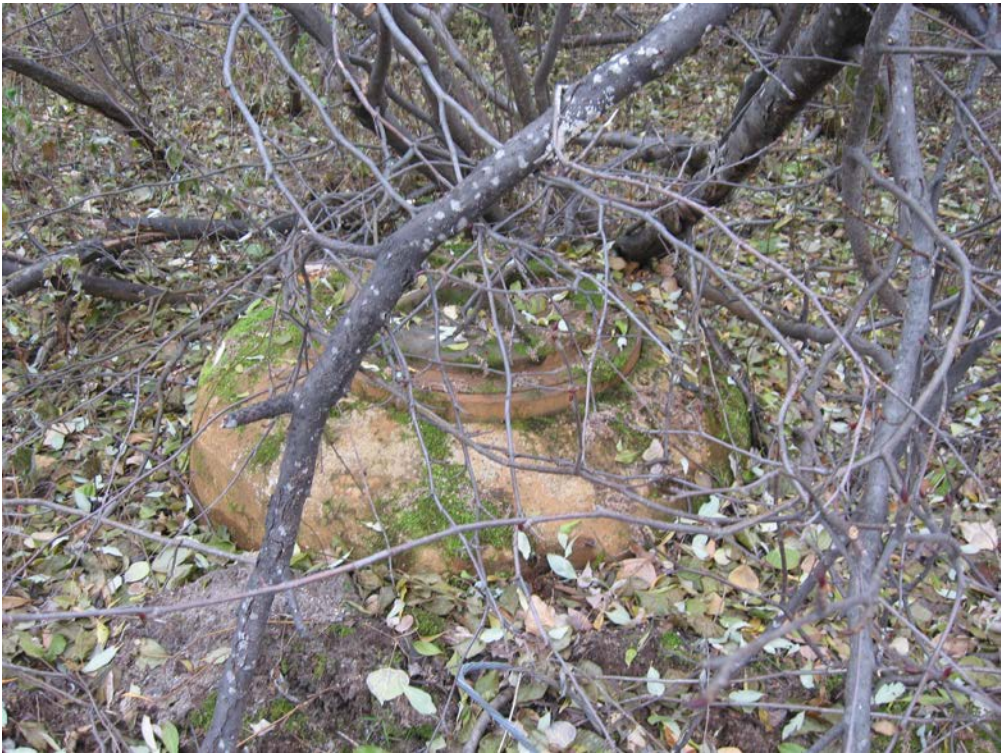
Photo 1 View of manhole cover (09-SD24) at the site
