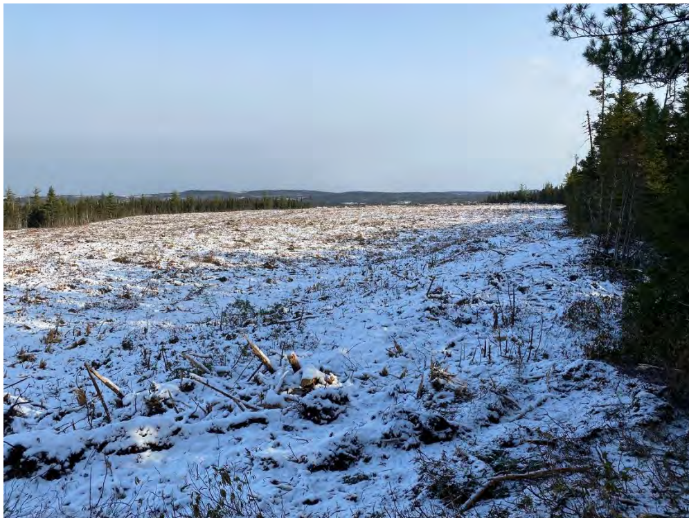
Plate 6: Example of current quarry ground conditions showing abundant grubbing material, looking northeast towards Phase 6-20
