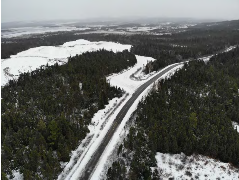
Plate 1: J-1 Quarry access road showing turn-off from Terra Nova Road, looking northeast
