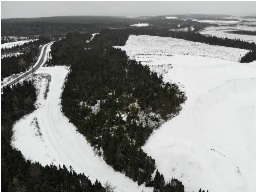
Plate 2: J-1 Quarry access road showing turn-off from Terra Nova Road, looking southwest towards Mac-Court quarry entrance
