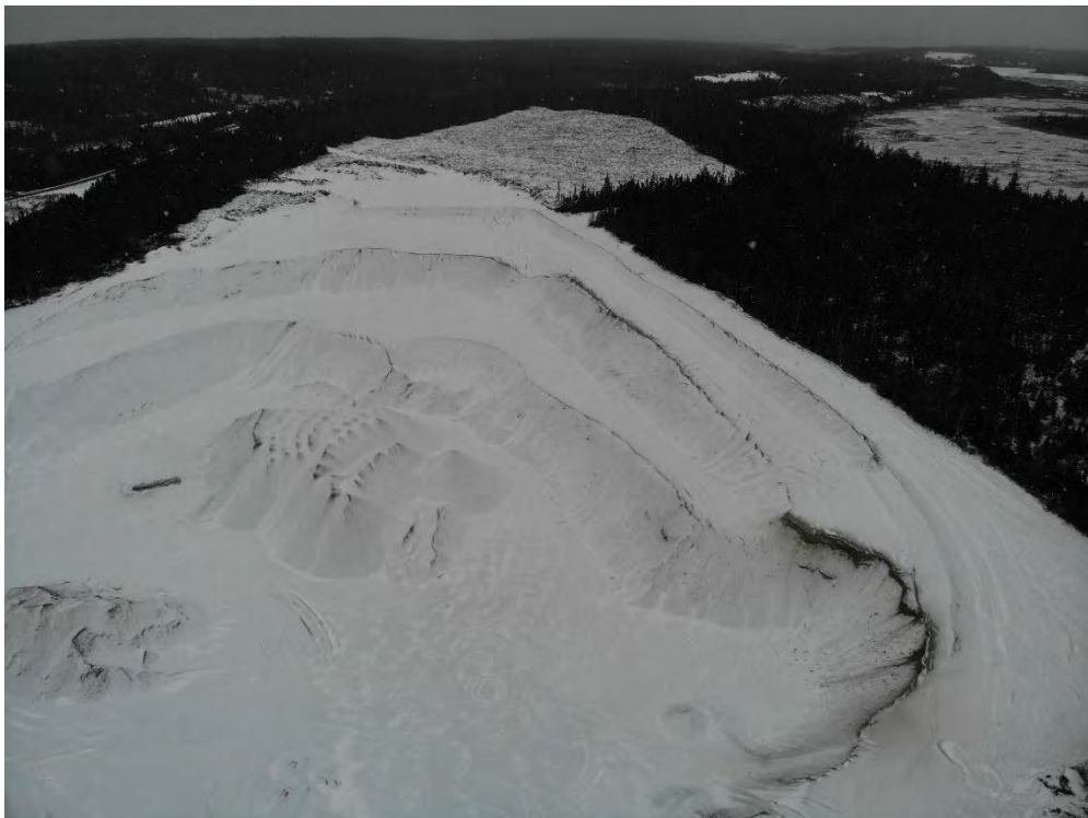
Plate 4: Quarry access road along J-1 lease boundary, looking southwest towards Mac-Court quarry entrance
