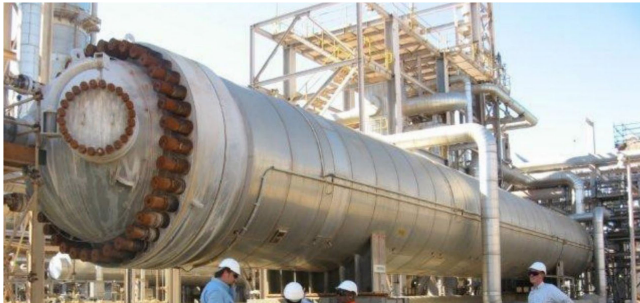
Figure 1.1 KBR's Horizontal Ammonia Synthesis Converter
