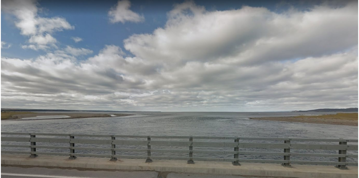
Fig. 5: Main Gut Trestle Downstream
