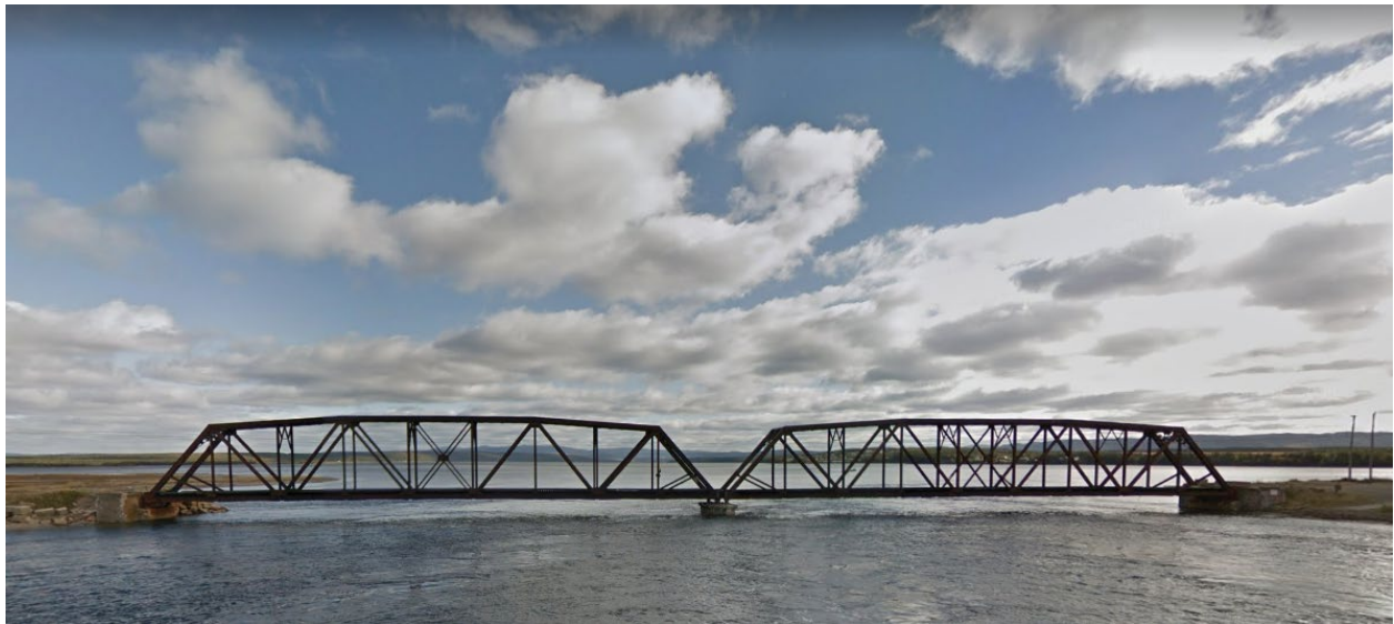
Fig. 4: Main Gut Trestle Upstream
