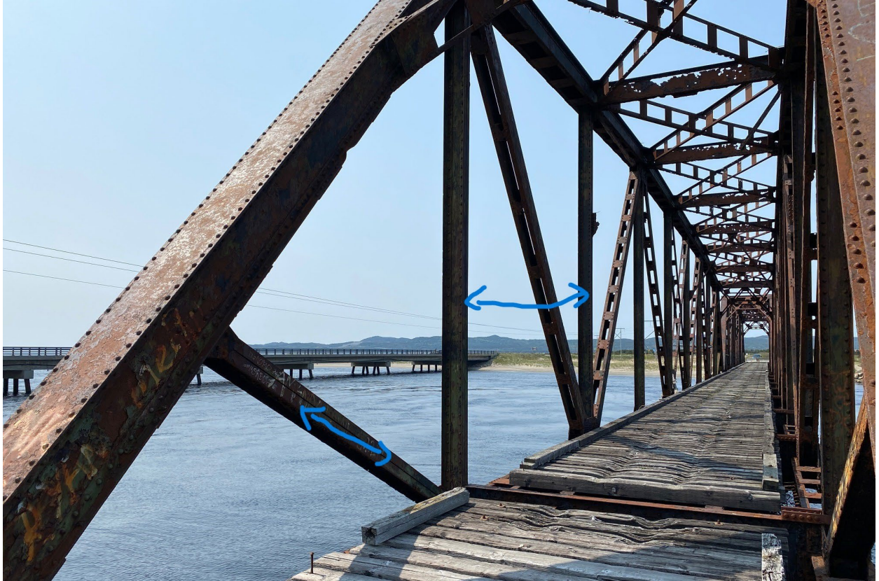
Fig. 6: Main Gut Trestle
