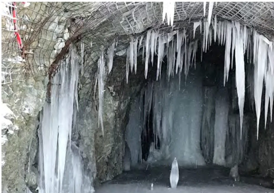
Figure 36: Adit Interior, February 2020
