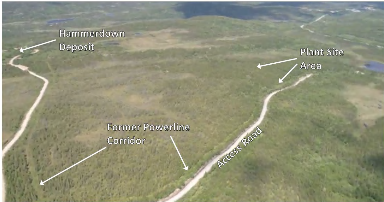
Figure 14: Existing Access Road and Electrical Infrastructure Corridor
