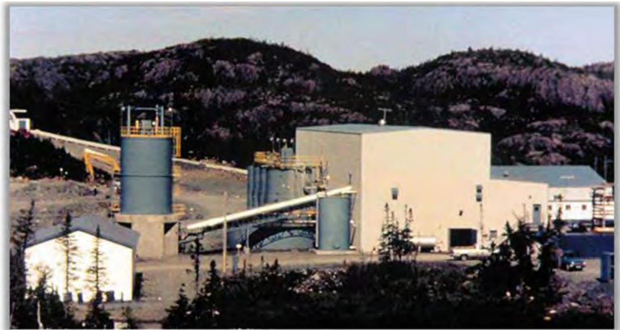
Figure 15: View of the Nugget Pond Mill
