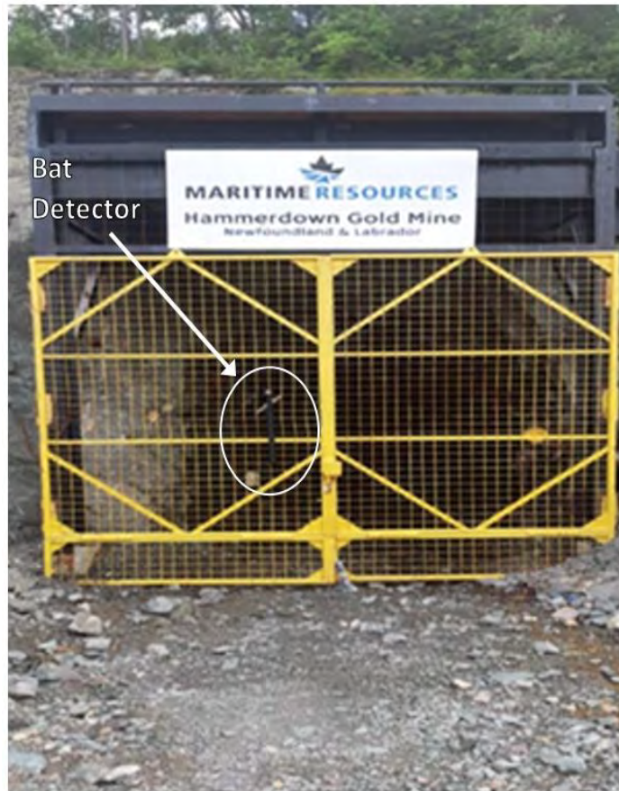
Figure 34: Bat Detector Installation at Existing Mine Portal
