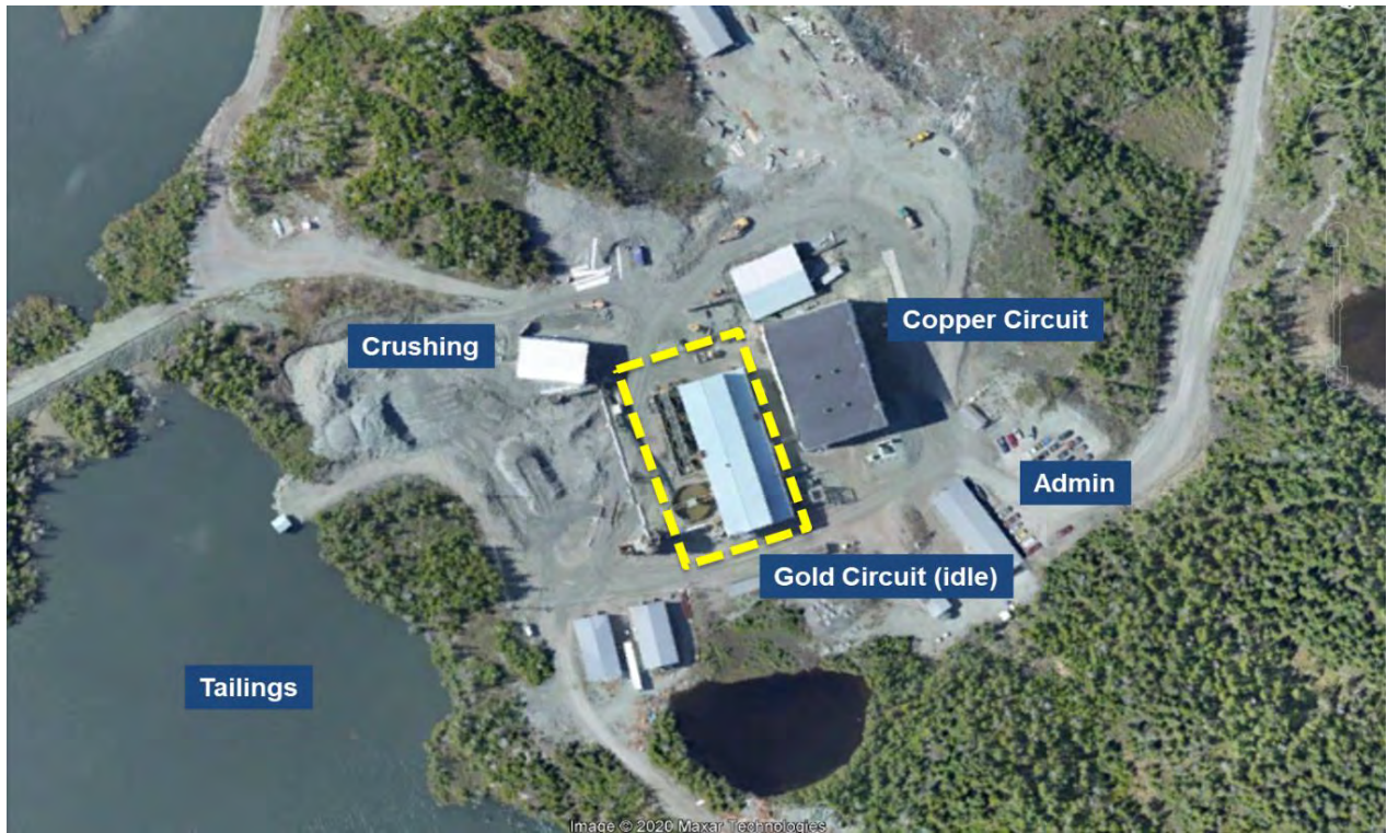
Figure 19: Existing Site Infrastructure at the Nugget Pond Mill
