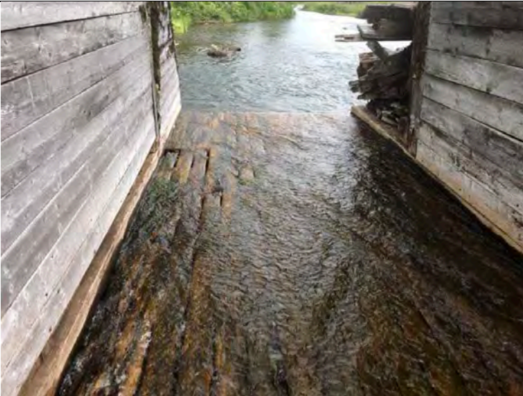
Photo 243 Deck of Long Lake Water Control Structure Facing Downstream
