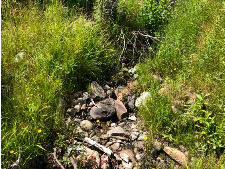
Photo 139 Stream Crossing C0023 0 to 50 m Upstream Facing Upstream
