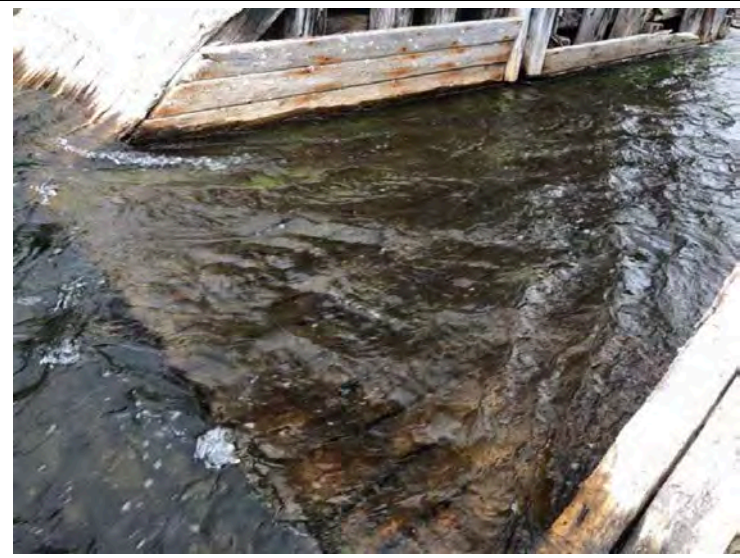
Photo 242 Deck of Long Lake Water Control Structure Facing Downstream
