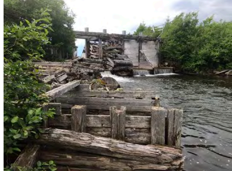
Photo 246 Long Lake Water Control Structure Facing Upstream
