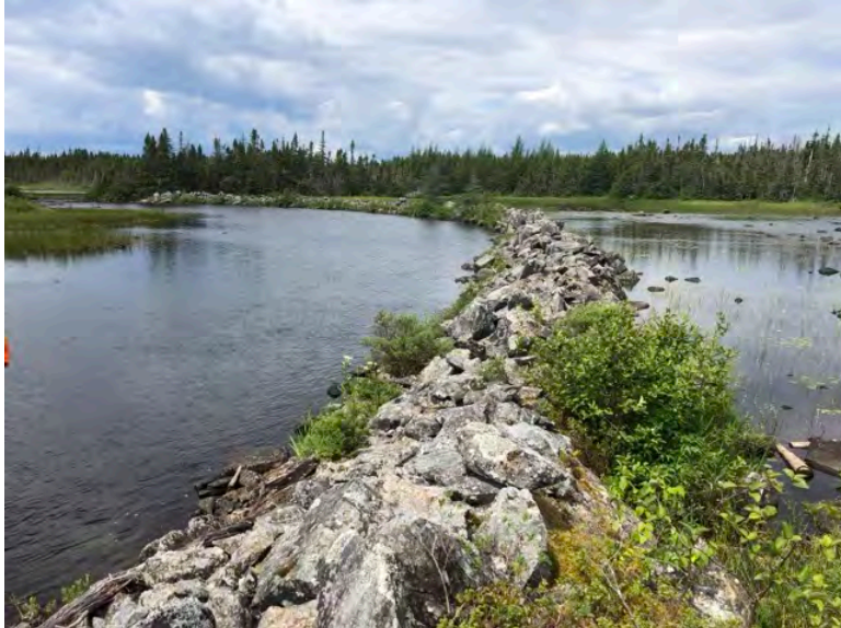
Photo 247 Main Channel Rock Wall (~130 m) in Outlet to Valentine Lake
