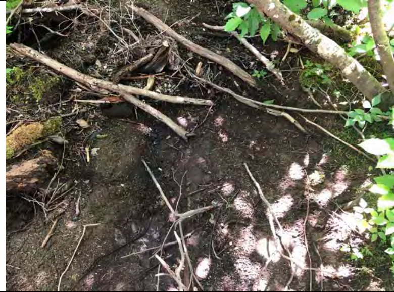
Photo 150 Stream Crossing C0028 0 to 50 m Downstream Facing Downstream
