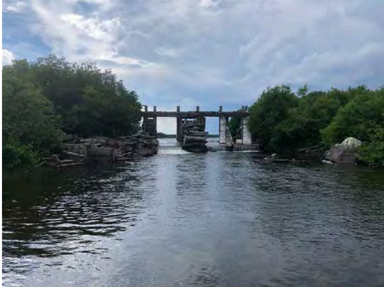
Photo 245 Long Lake Water Control Structure Facing Upstream
