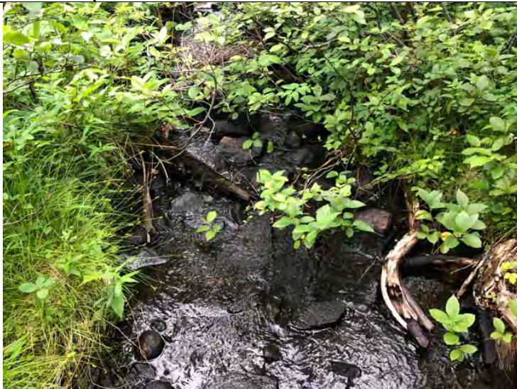
Photo 215 Stream Crossing C0057 0 to 50 m Upstream Facing Upstream
