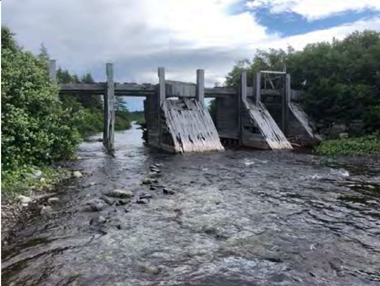
Photo 241 Long Lake Water Control Structure Facing Downstream
