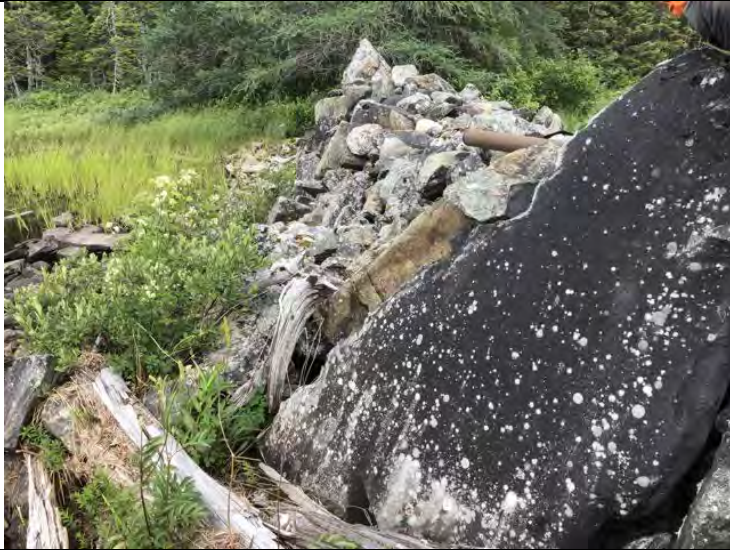
Photo 249 Upstream (20 m) Rock Wall in Outlet to Valentine Lake
