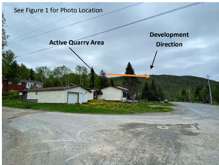
Plate 18: Photo Taken from Person Height Looking at Quarry Area (500 m to quarry boundary)
