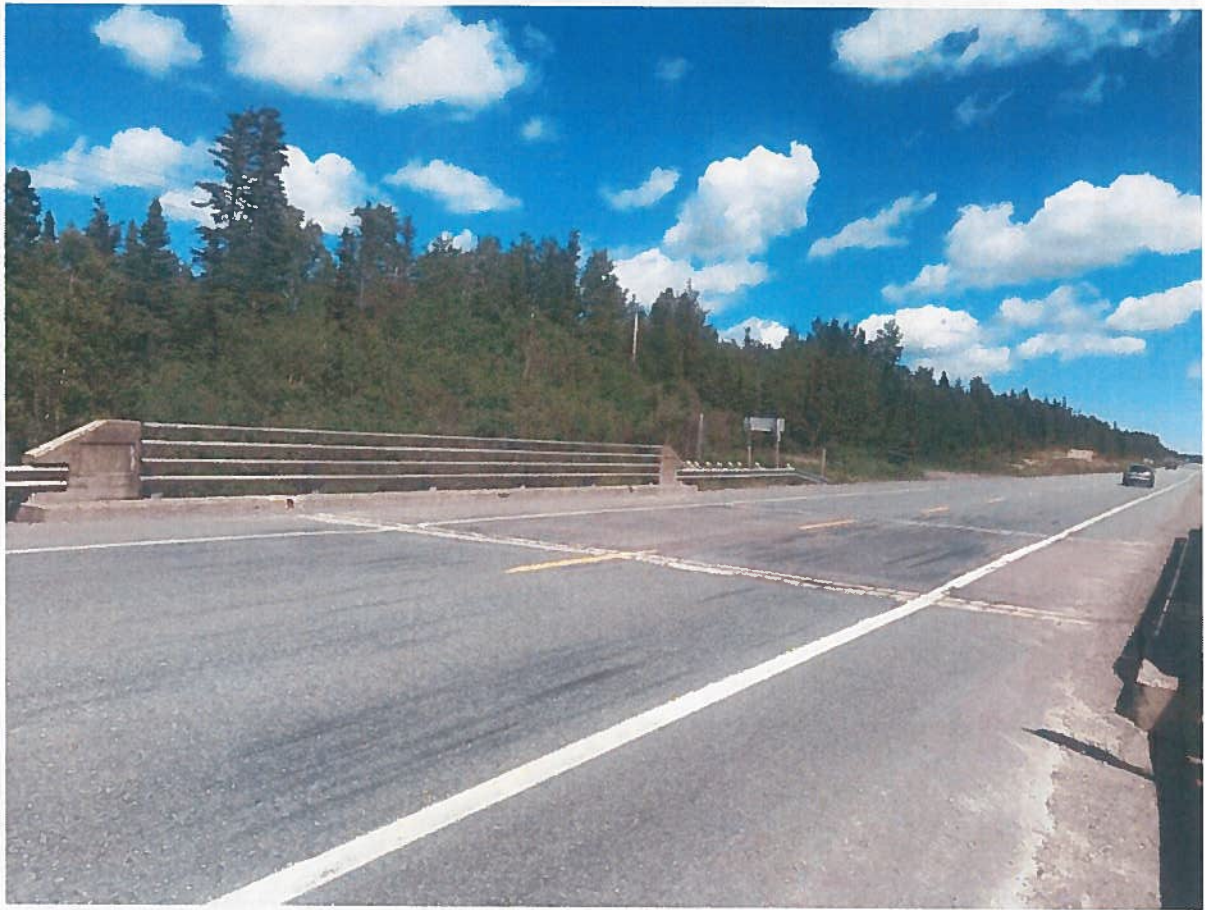
Photo 1: Bridge View Top
