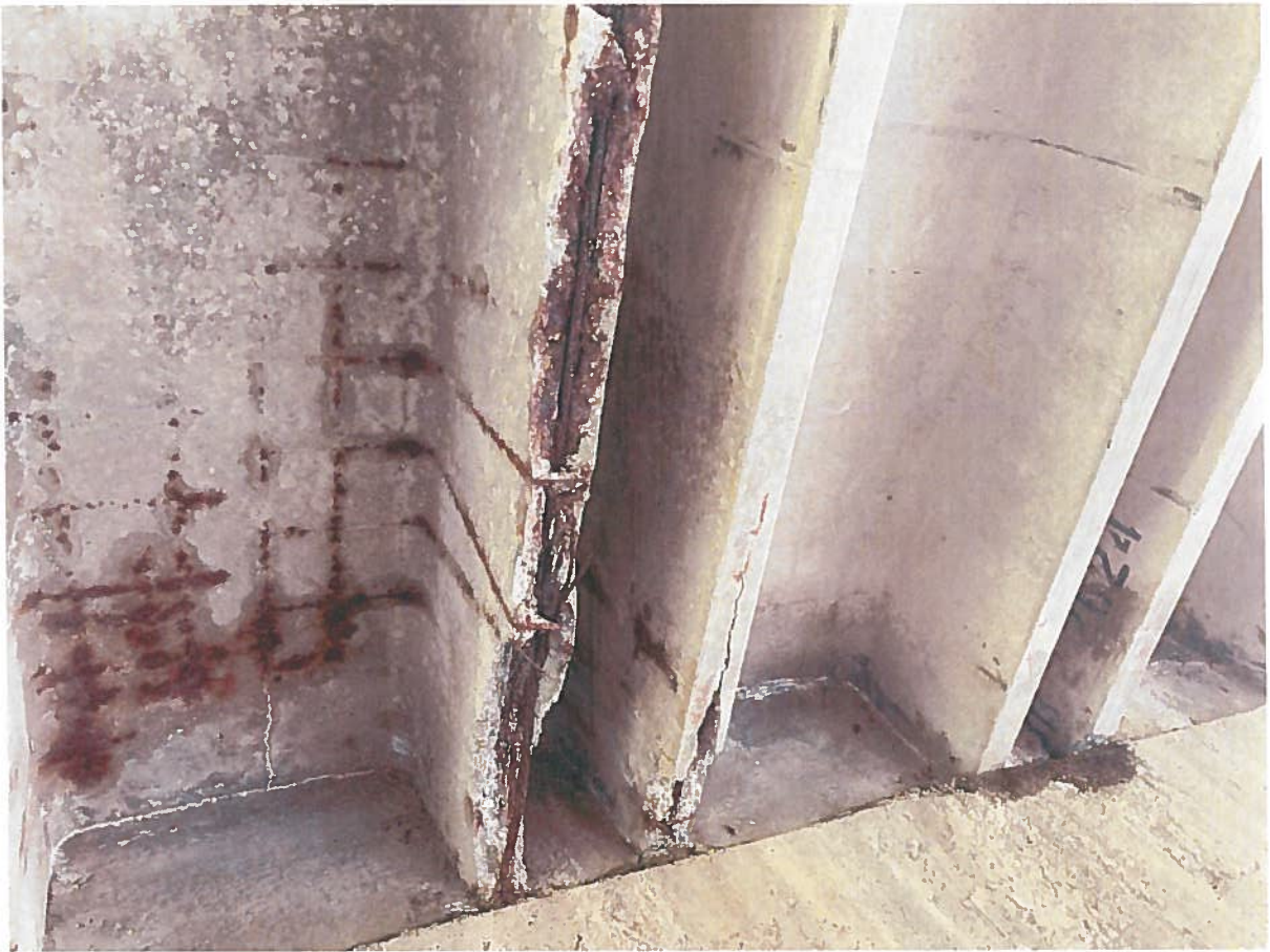
Photo 2: Bridge Deterioration
