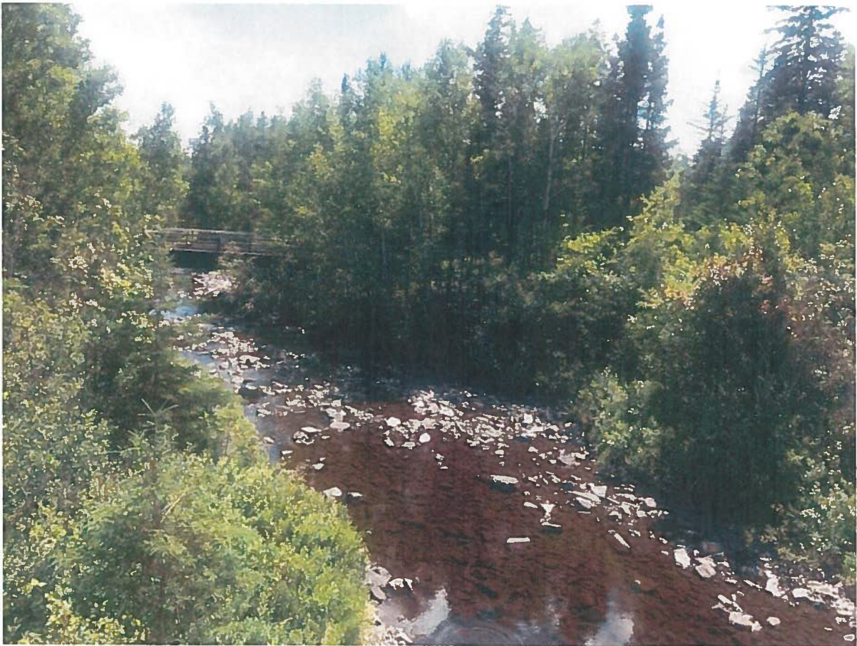
Photo 5: Downstream View of Aspen Brook
