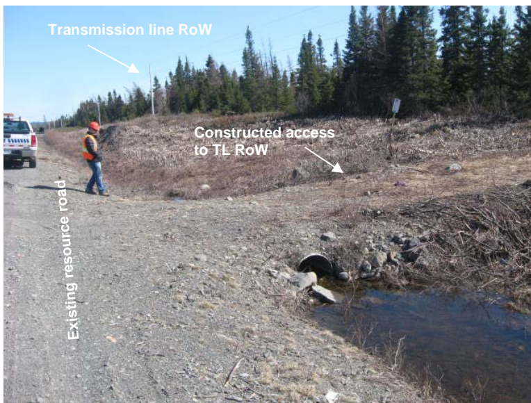
Photo 3 Typical Access to TL RoW from Existing Resource Road
