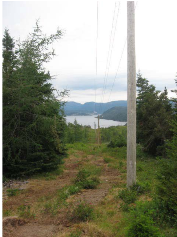
Photo 6 Typical RoW for a Single Pole Line
