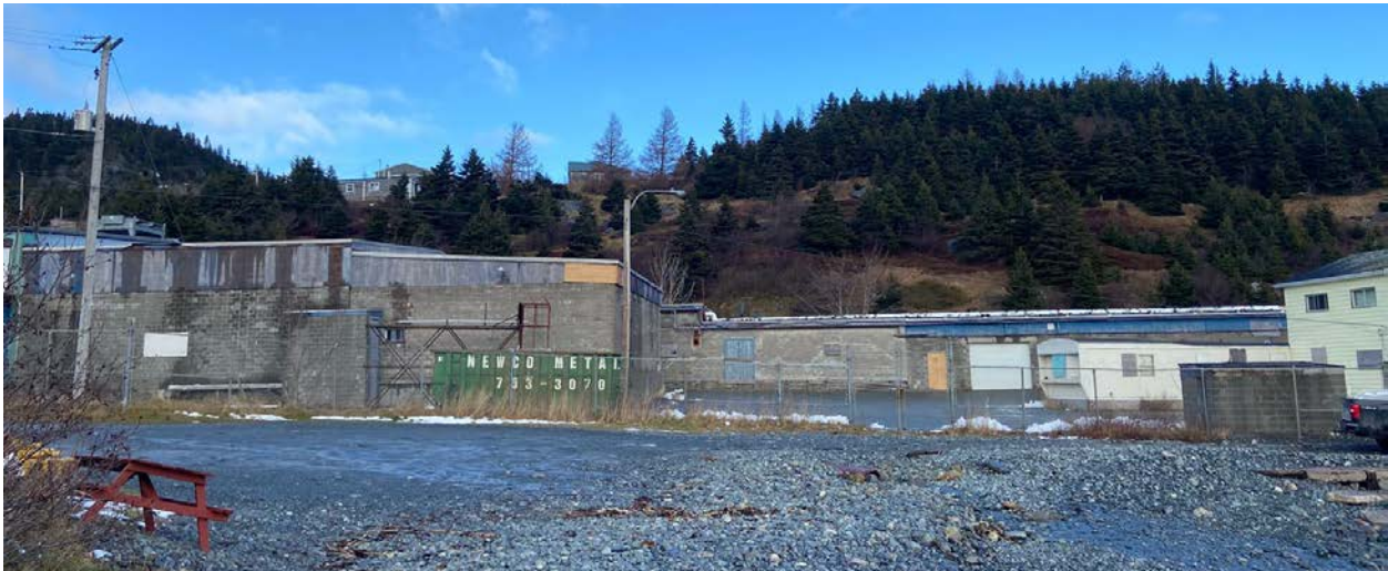
Figure 114 - Tors Cove Beach Street Light
