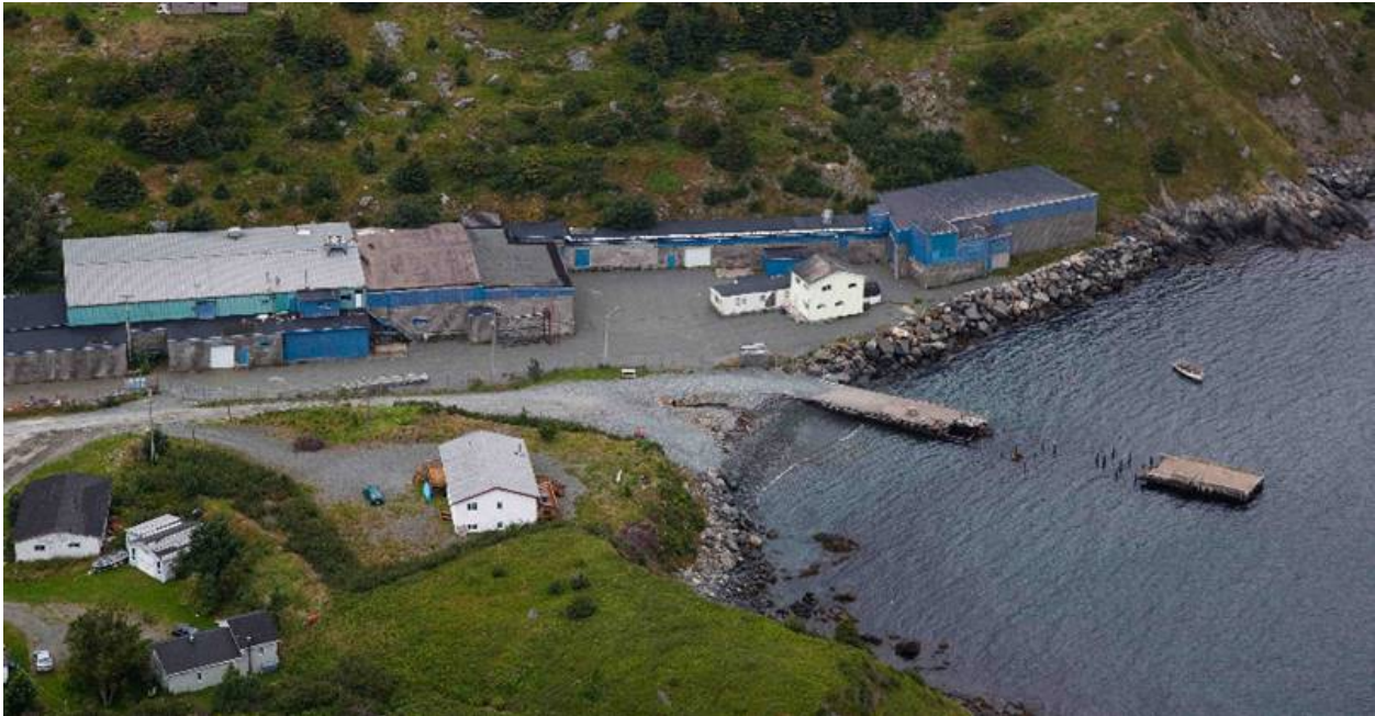
Figure 104 – Aerial Photo of Tors Cove Facility
