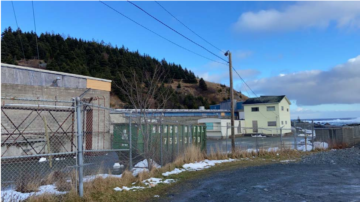
Figure 116 - Tors Cove Beach Street Light
