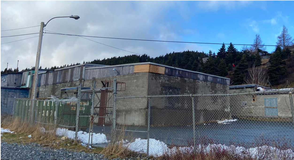
Figure 115 - Tors Cove Beach Street Light
