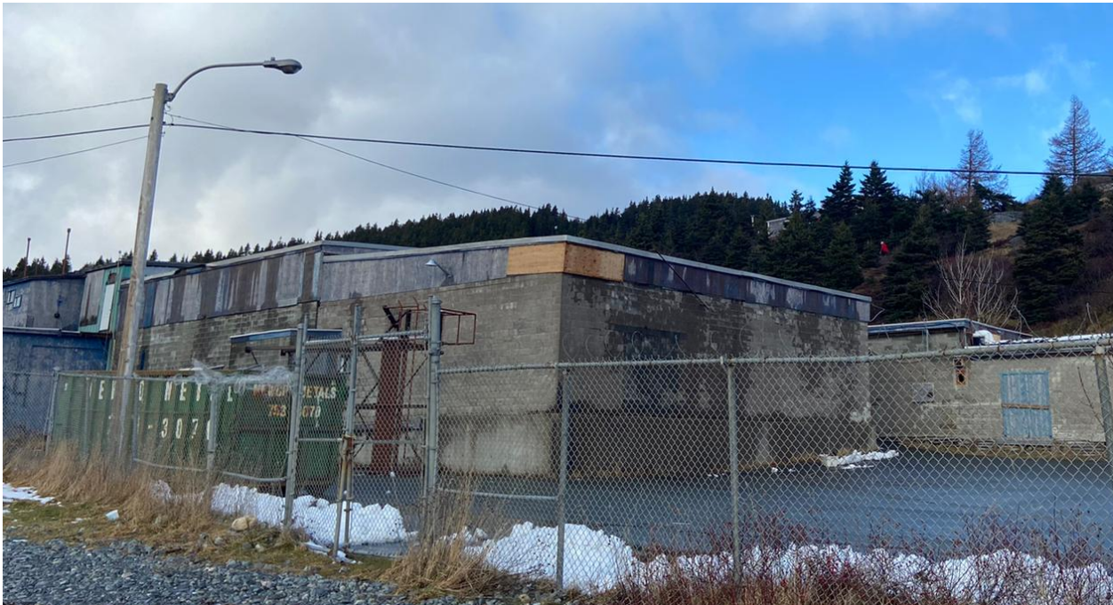
Figure 63 - Tors Cove Beach Street Light
