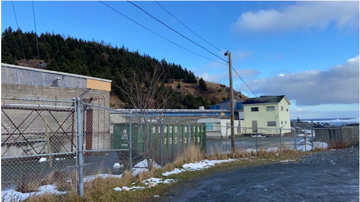
Figure 64 - Tors Cove Beach Street Light
