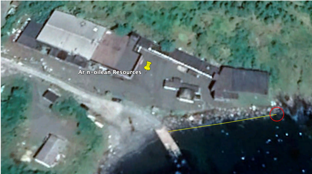
Figure 8 - Facility's Discharge Outflow (satellite view)
