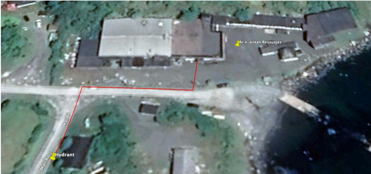
Figure 7 - Fire Hydrant Supply Route
