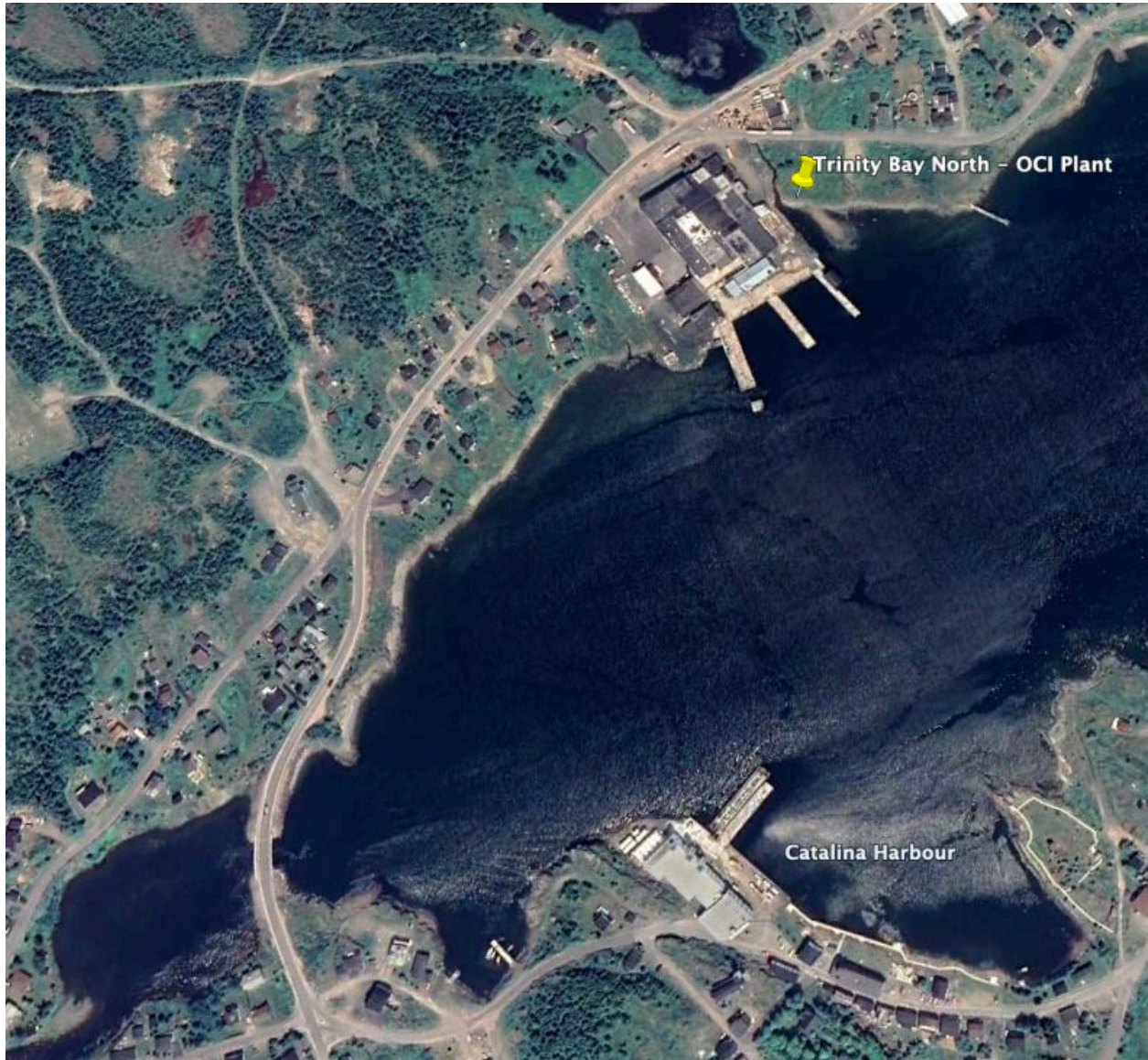
Figure 67 - Trinity Bay North - OCI Fish Plant
