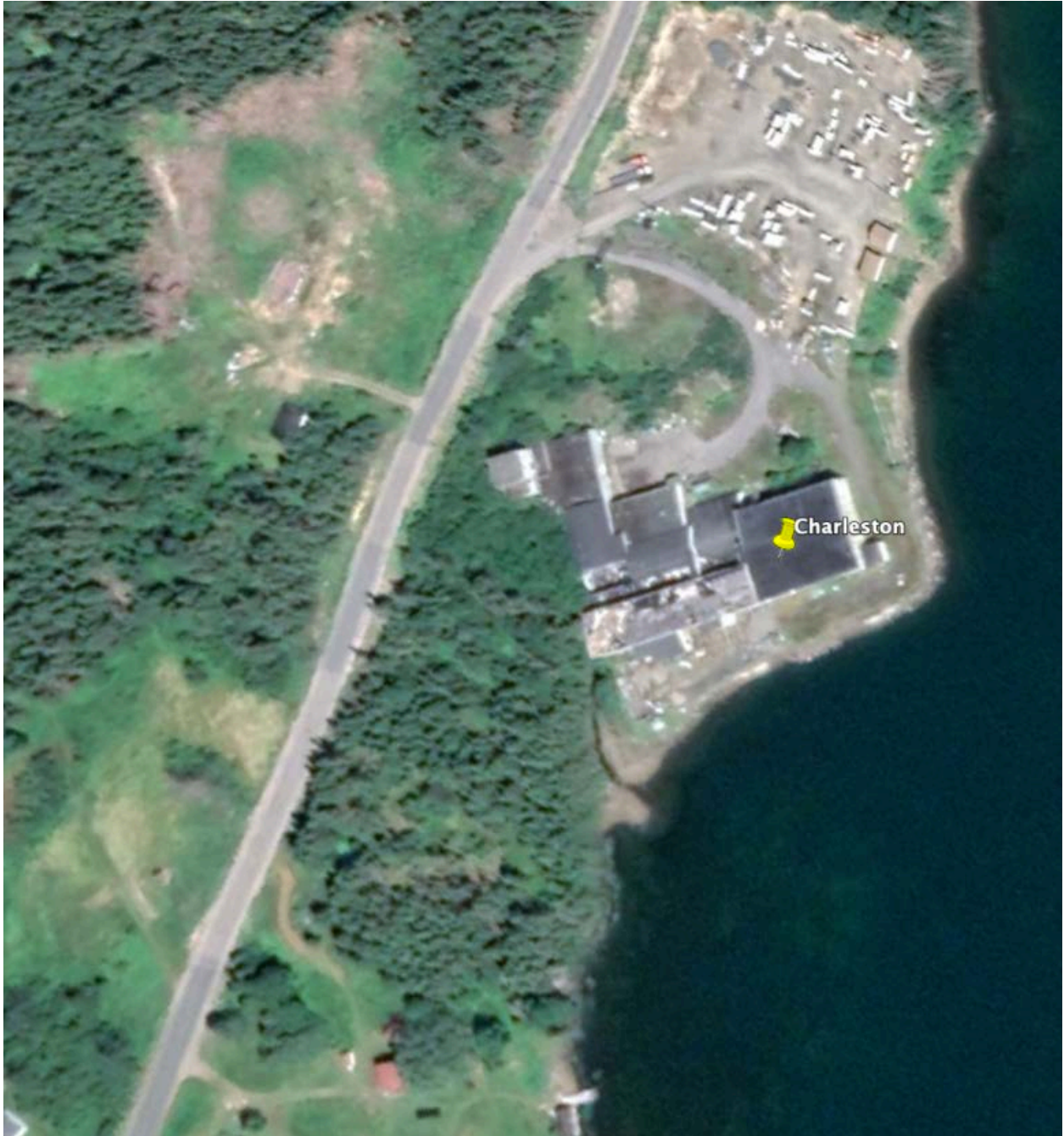
Figure 70 - Charleston Fish Plant
