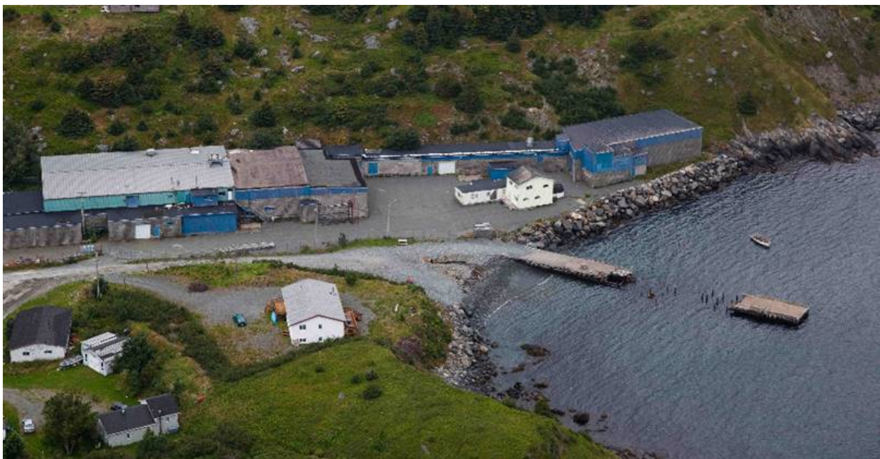
Figure 78 - Tors Cove Facility - Aerial Photo
